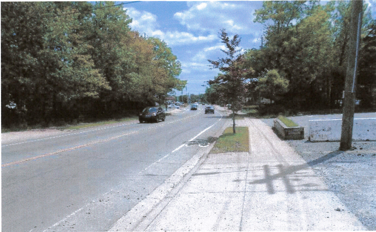
Figure 5: Site Access #1 Sight Line South of Access (Looking to the Right)
