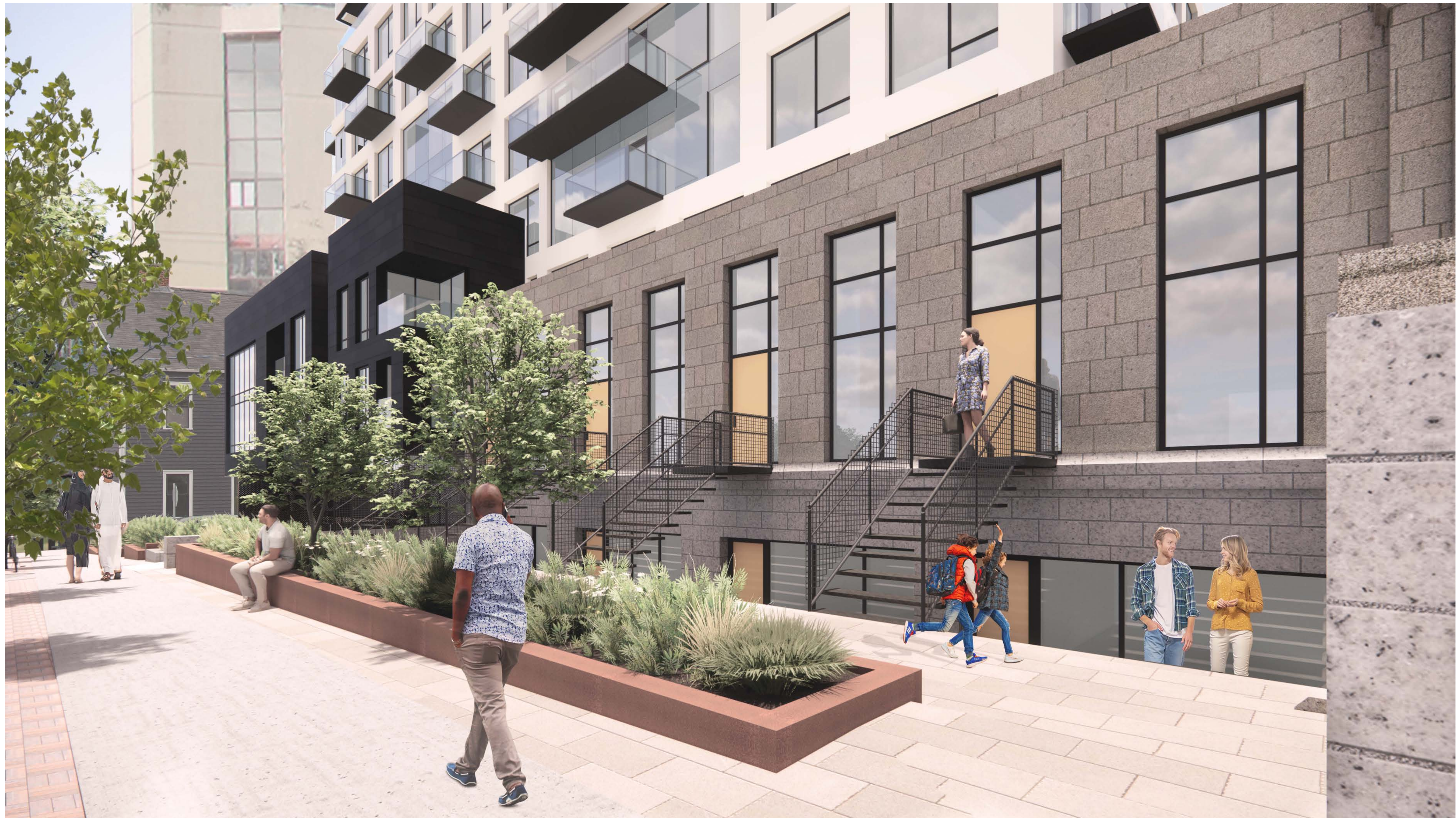
View from Queen Street (Townhouse entrance)
