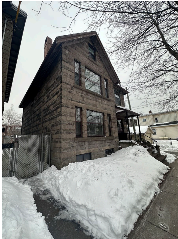
Figure 18: West and north elevations of 1735 Henry Street (February 16, 2024)
