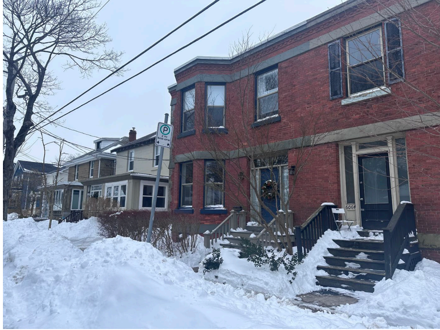
Figure 26: Maxwell constructed houses along Cedar Street near Henry Street intersection (February 2024)
