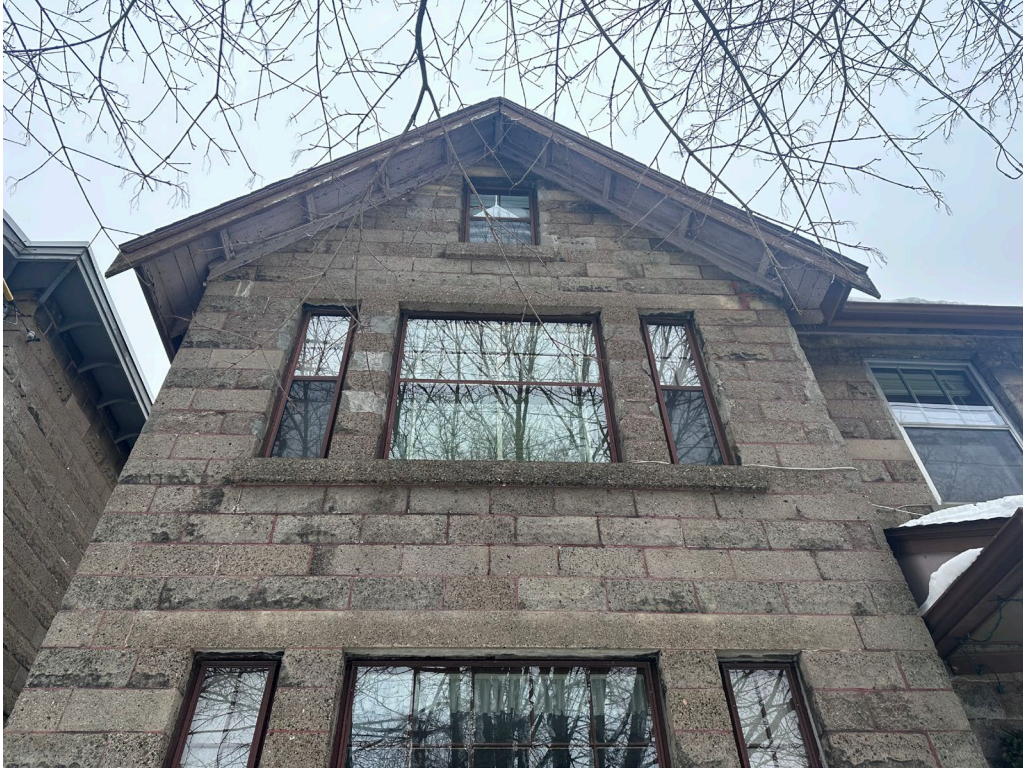
Figure 21: Wood bracketed cornice on 1735 Henry Street (February 16, 2024)
