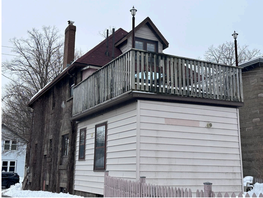
Figure 19: East and south elevation of 1735 Henry Street (February 16, 2024)
