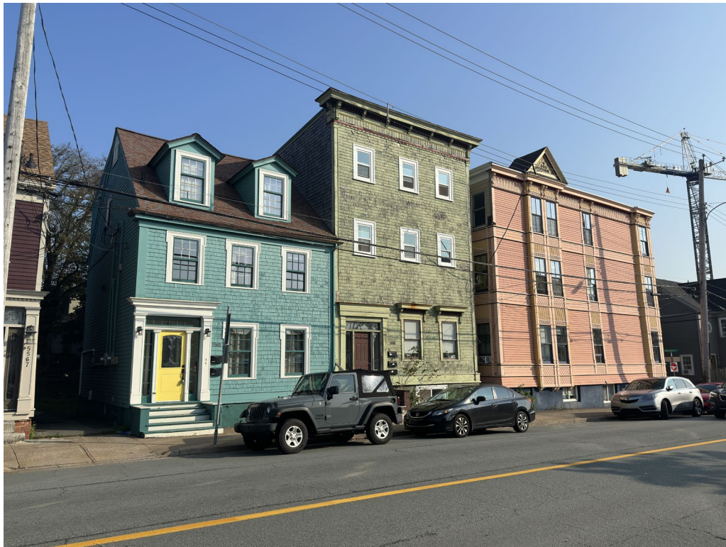
Figure 11: South and west elevations of 5561 Cogswell Street (September 2023)
