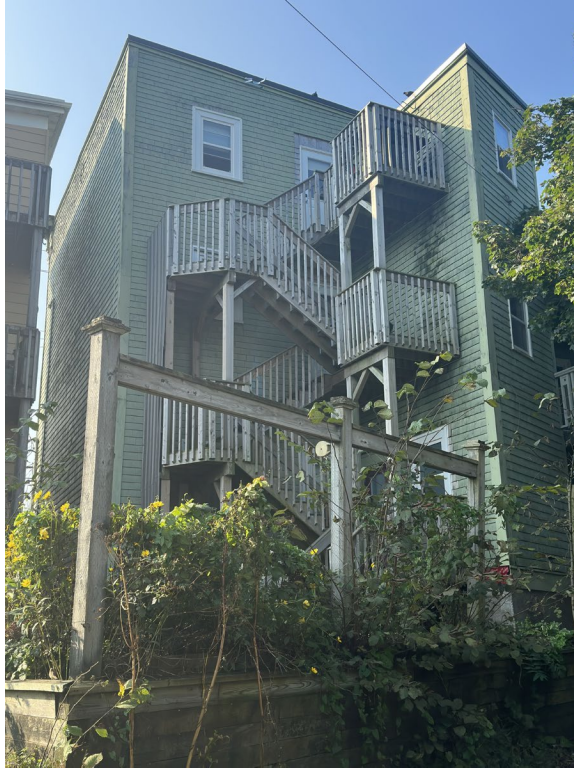
Figure 12: North and east elevations of 5561 Cogswell Street (September 2023)
