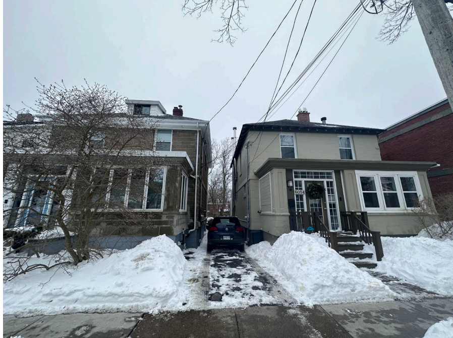
Figure 9: 6050 and 6054 Cedar Street (February 2024)
