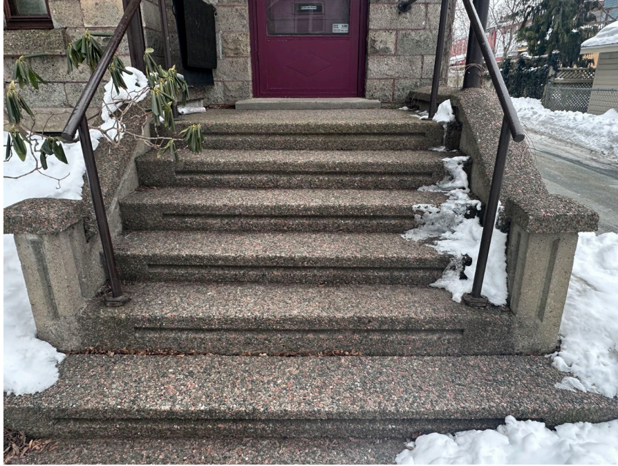
Figure 23: Stairs leading to main entrance on the west elevation (February 16, 2024)
