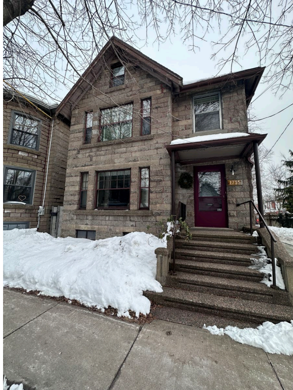
Figure 17: West Elevation of 1735 Henry Street (February 16, 2024)
