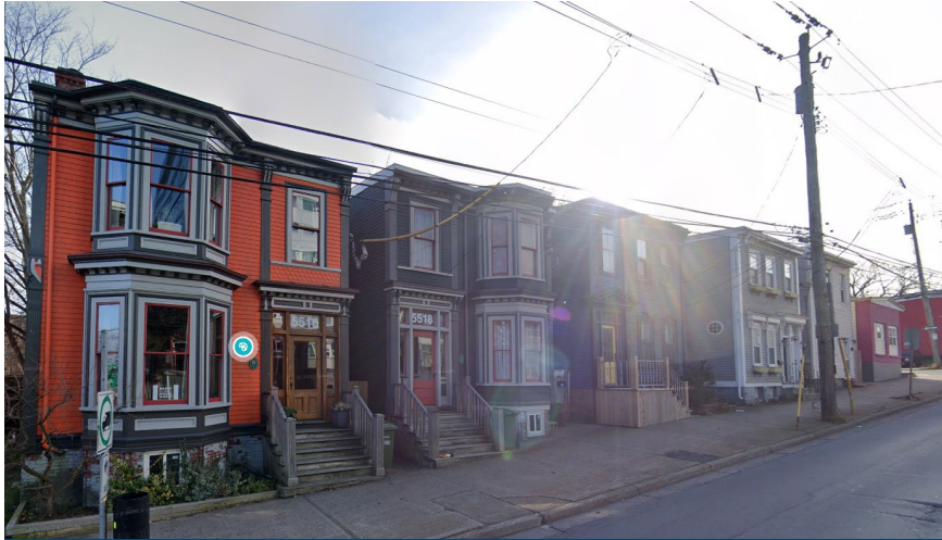
Late Victorian streetscape on North Street (November, 2022).
