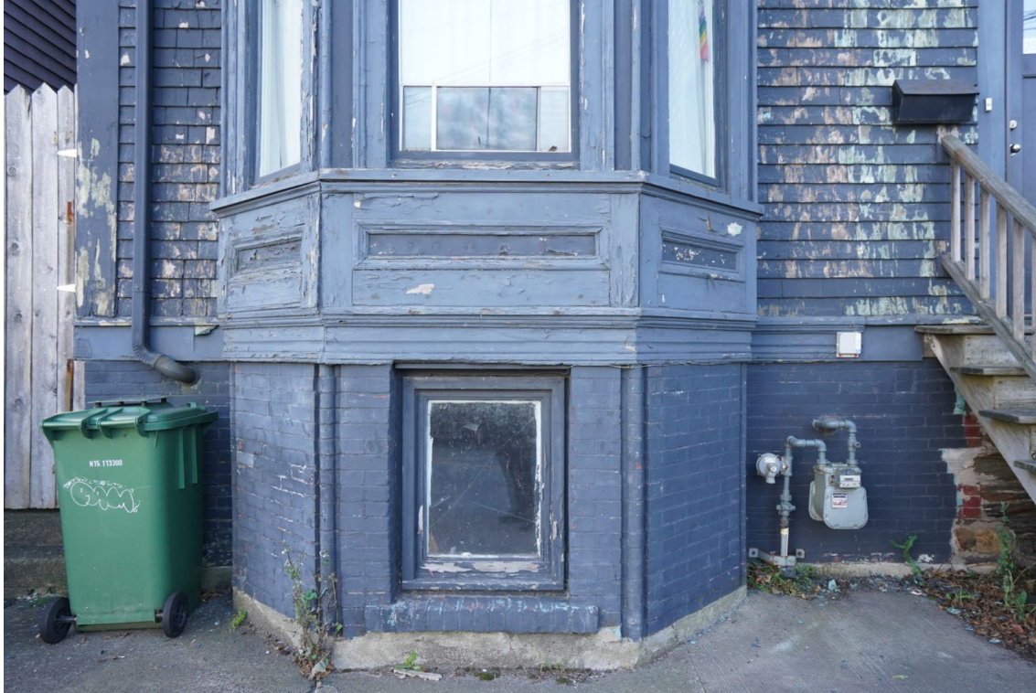
Above: Close-up of stone and brick foundation
