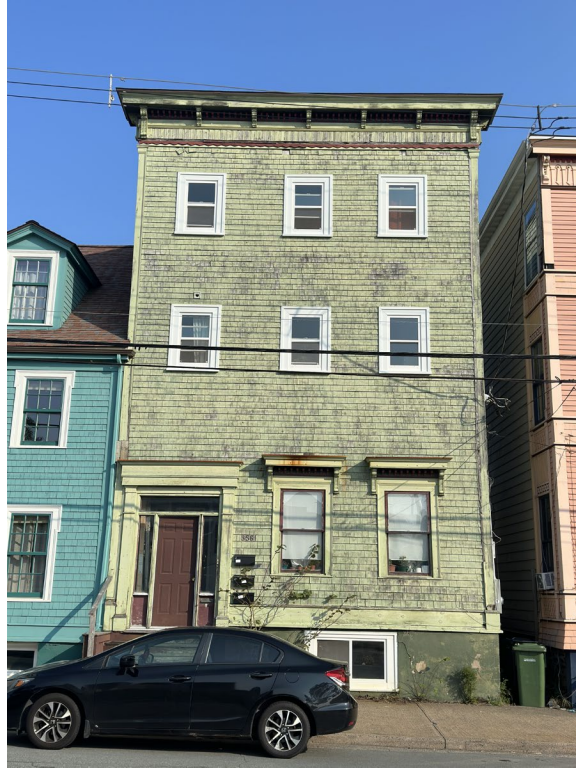
Figure 10: South elevation of 5561 Cogswell Street (September 2023)
