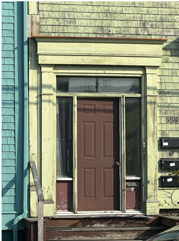
Figure 15: South elevation entrance with moulded entablature, transom, and sidelights (September 2023)
