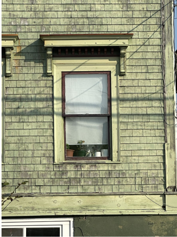
Figure 14: South elevation first-storey windows with bracketed moulding hoods (September 2023)
