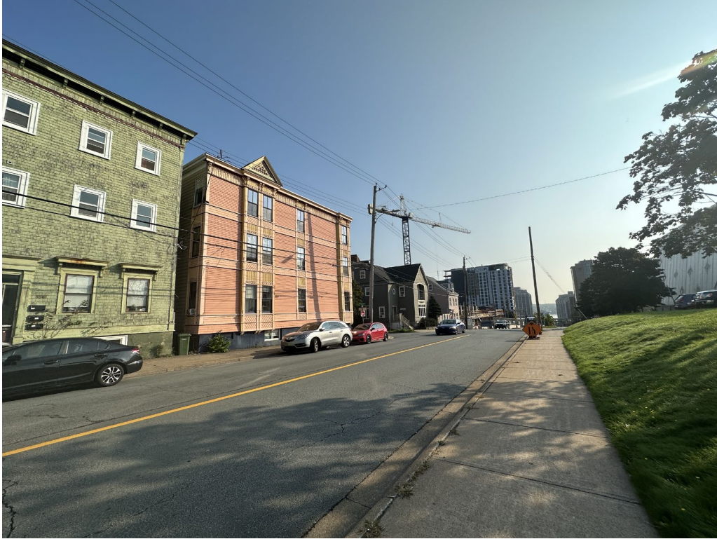
Figure 22: Cogswell Street facing east from across the street from 5561 Cogswell Street, showing 2010 Creighton Street in the centre (September 2023)
