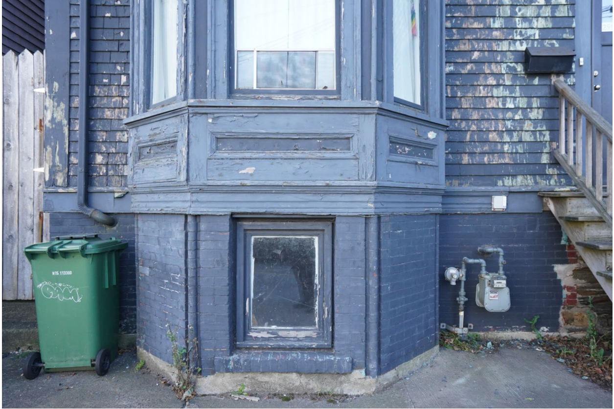
Figure 16: Details of foundation (October 23, 2023)
