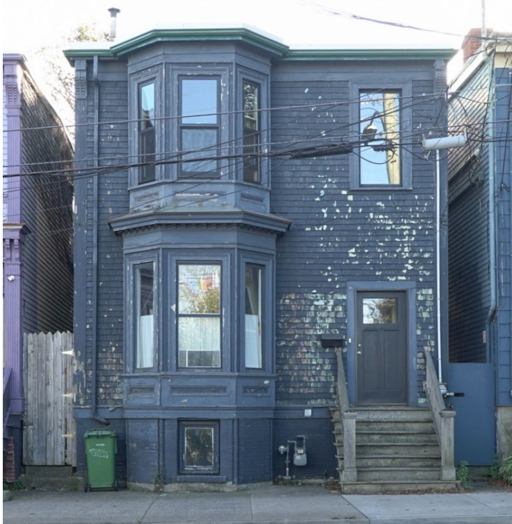
Figure 12: East elevation (October 23, 2023)
