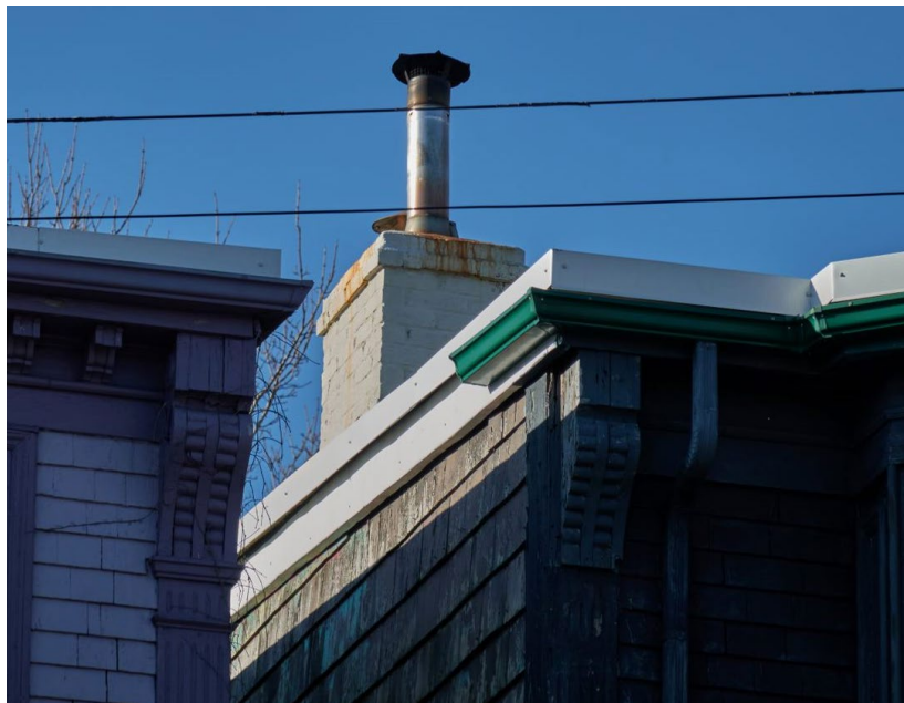
Figure 15: Details of brick chimney (November 17, 2023)
