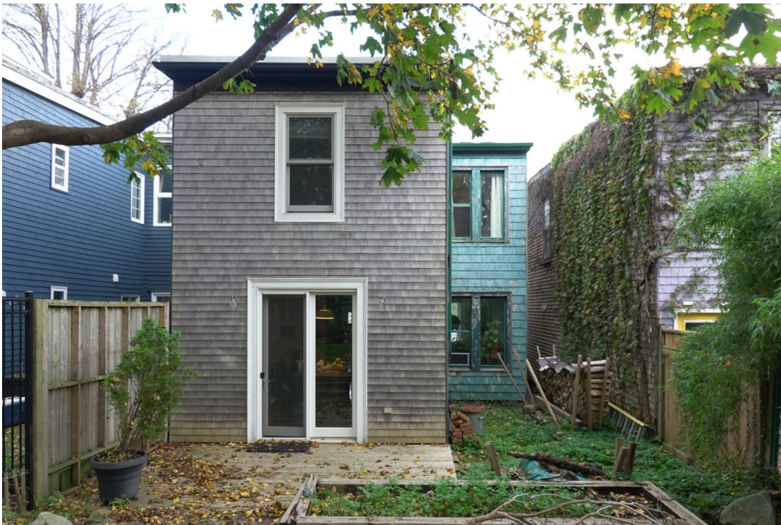
Figure 13: West Elevation (October 23, 2023)
