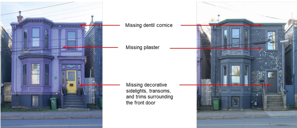
Figure 19: Façade comparison between 2548 and 2552 Gottingen Street (October 23, 2023)
