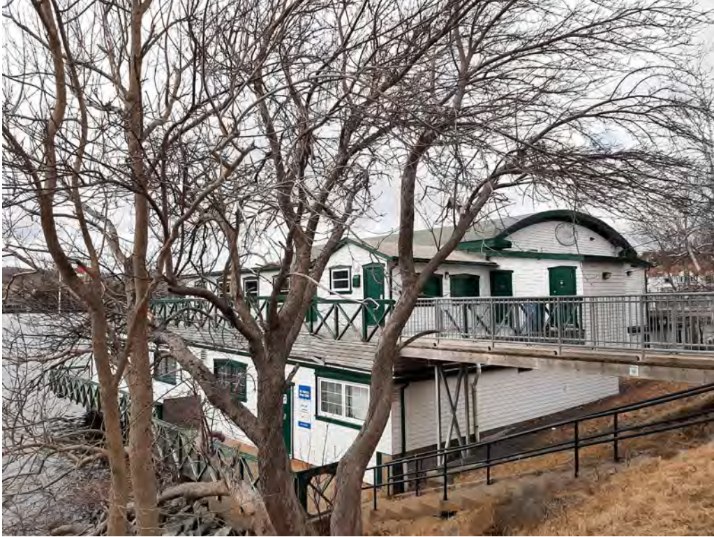
Figure 26: South elevation (30 March 2023)
