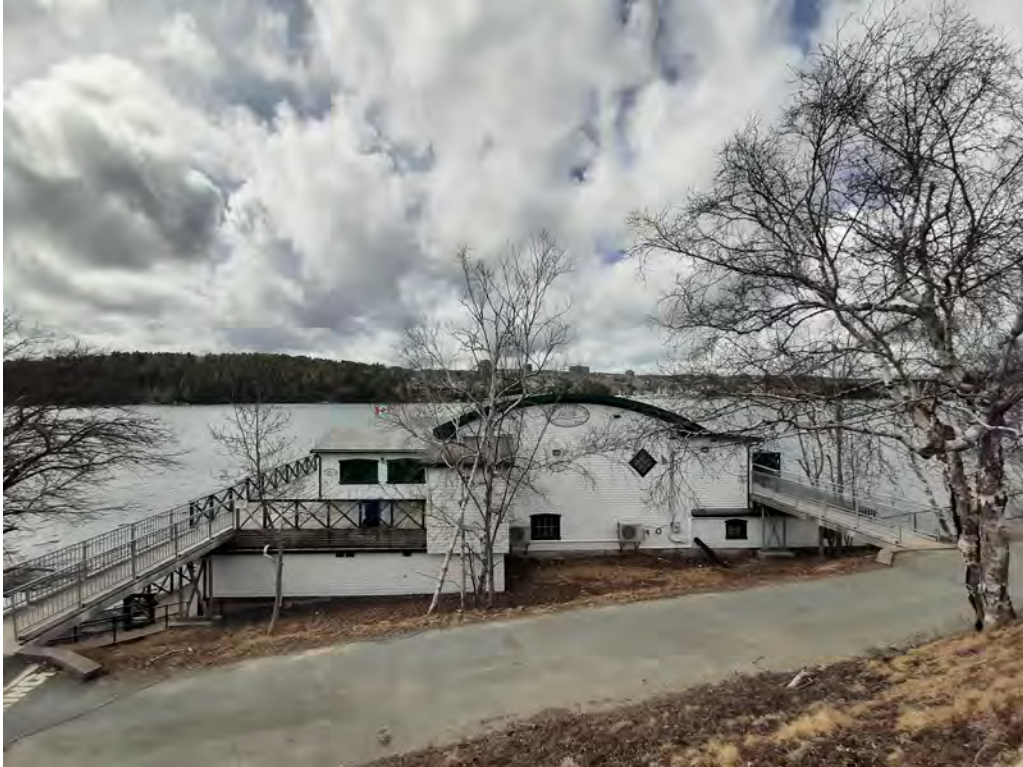
Figure 24: East Elevation of 1641 Fairfield Road (30 March 2023)
