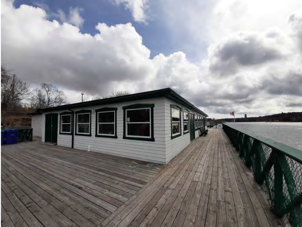
Figure 30: Upper decking (30 March 2023)
