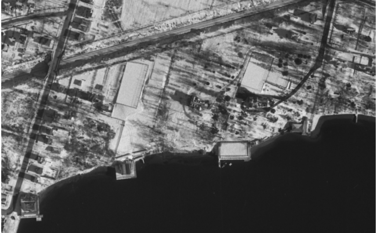
Figure 38: Aerial Imagery from 1955 with St. Mary's Boat Club identified in red (Source: Halifax Municipal Archives)
