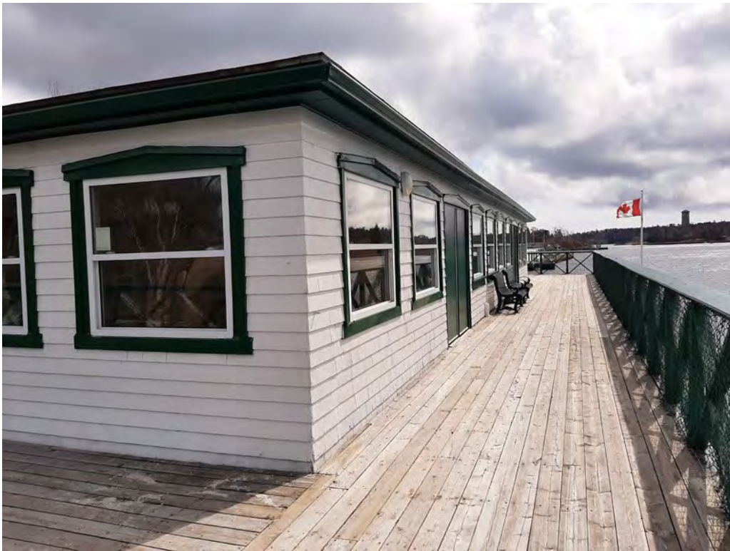
Figure 27: Upper deck of the west elevation (30 March 2023)
