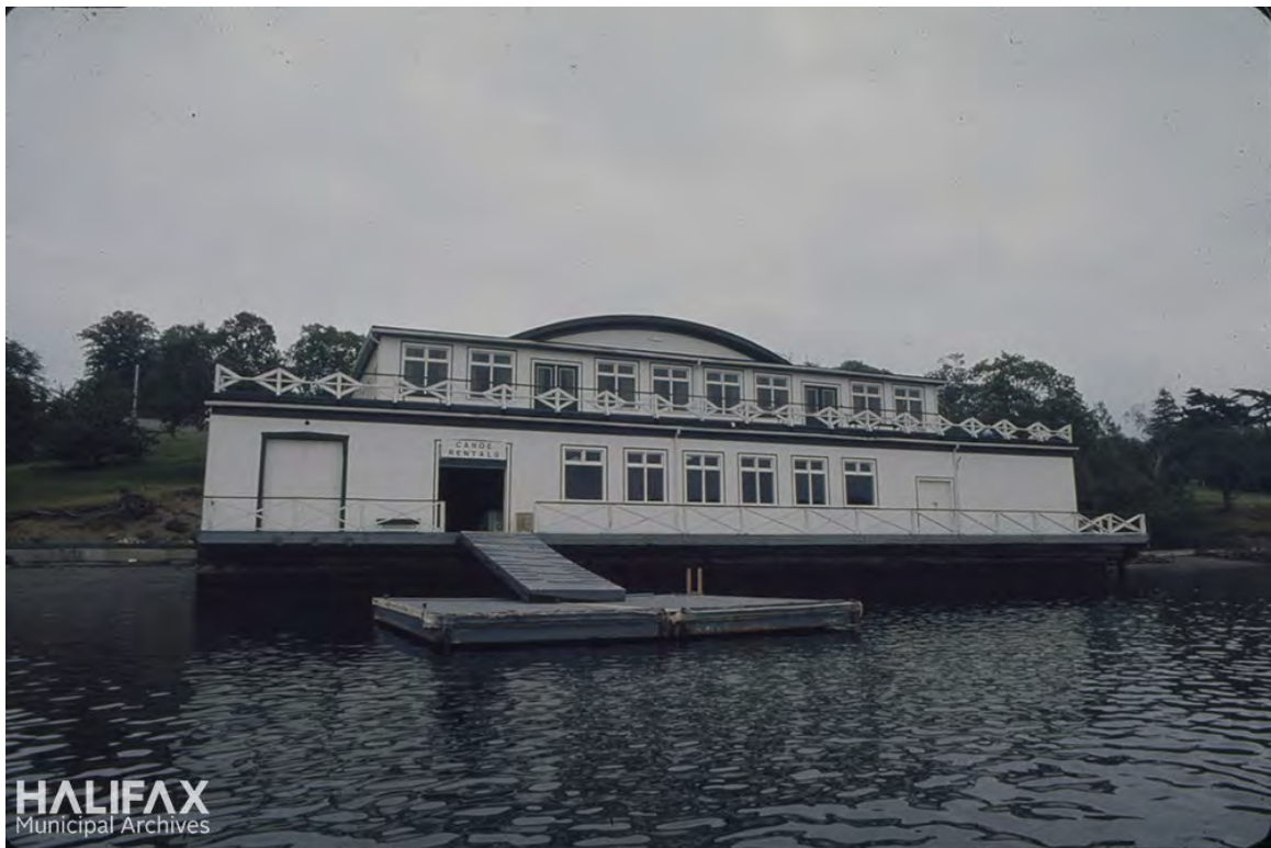
Figure 34: West elevation of St. Mary's Boat Club ca. 1970s (Source: Halifax Municipal Archives)
