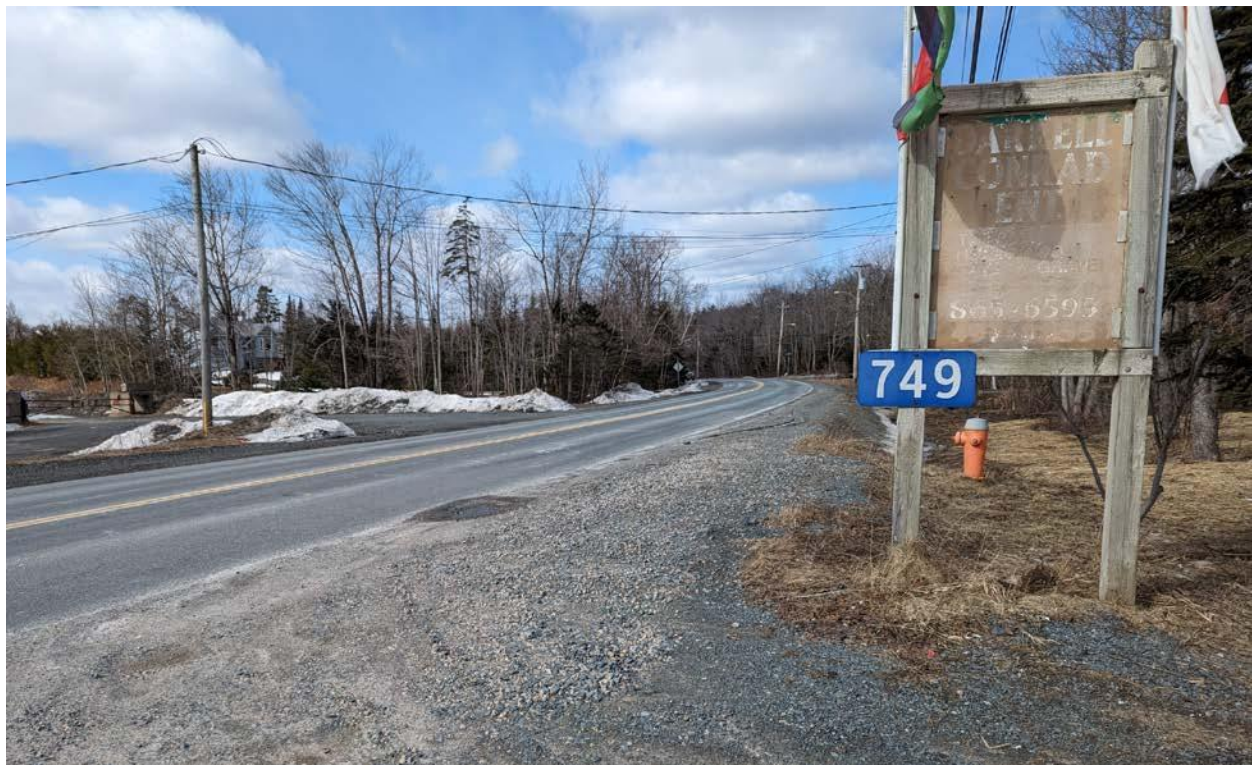
Figure 3: Sight Line West of Access (Looking to the Right)
