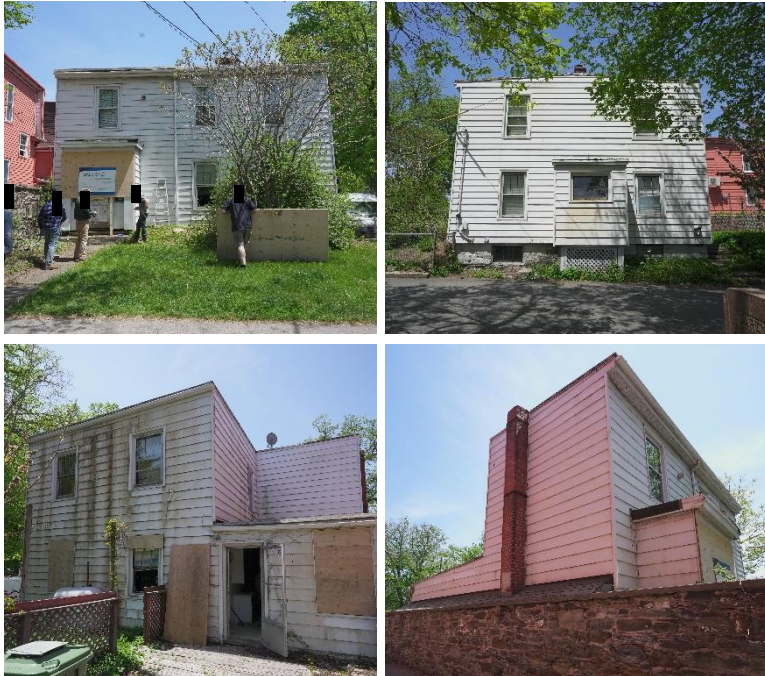
Elevation photos taken during site visit (May 31, 2023)
