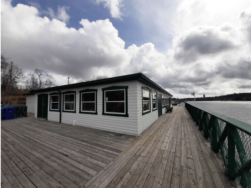
Figure 30: Upper decking (30 March 2023)
