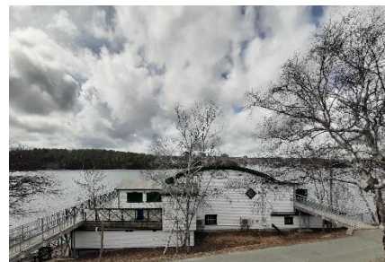
Figure 1: 1641 Fairfield Road (Staff photo, March 30, 2023)
