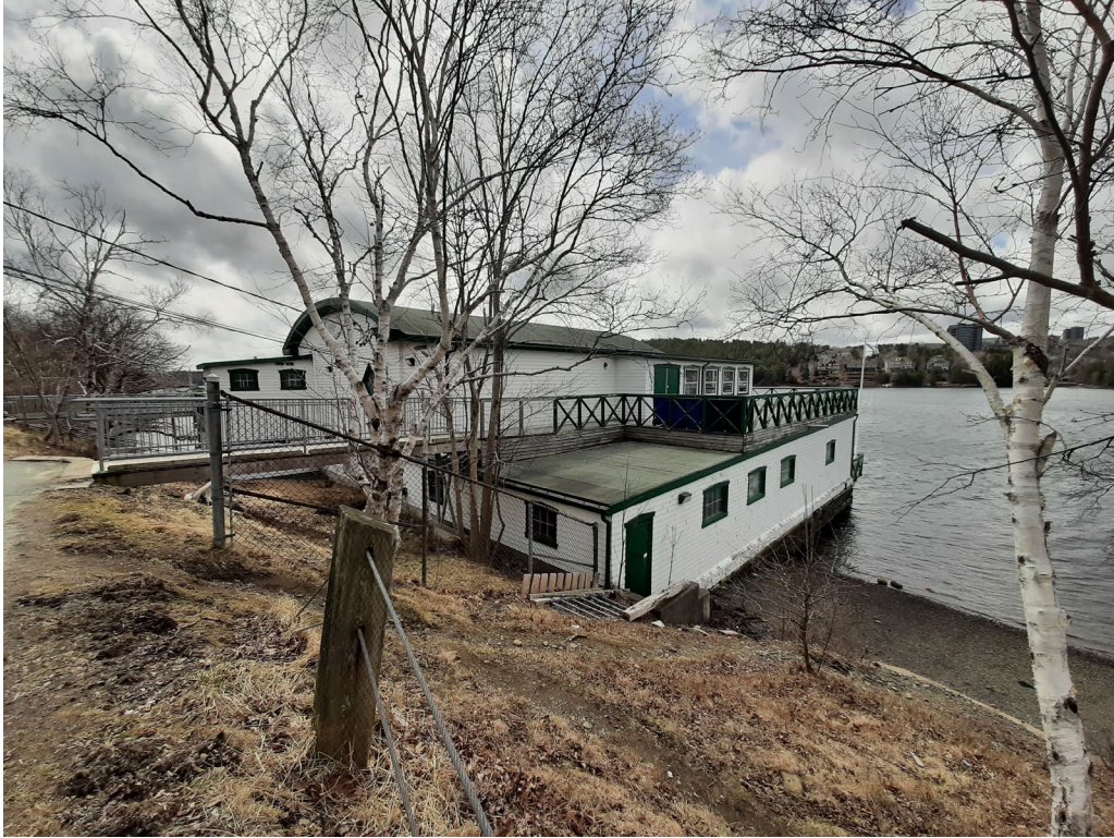
Figure 28: North elevation (30 March 2023)
