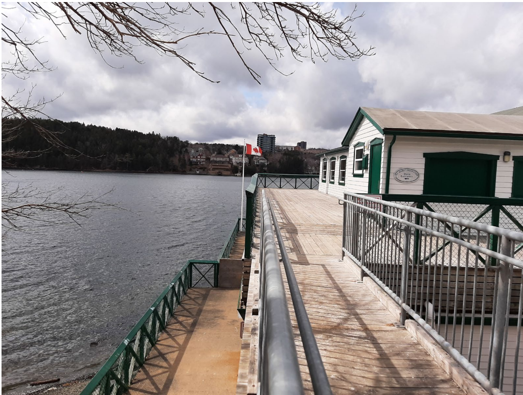
Figure 29: Upper and lower deck of south elevation (30 March 2023)
