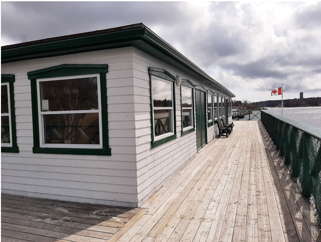
Figure 27: Upper deck of the west elevation (30 March 2023)
