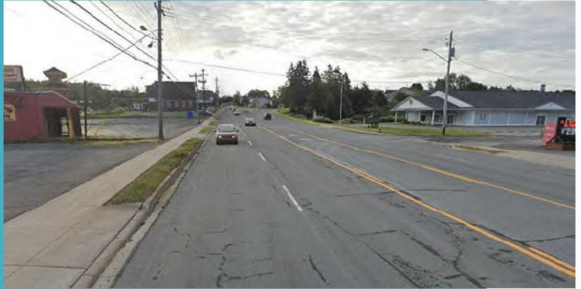
This configuration is shown at the **Cole Harbour Road and Bissett Road Intersection** in the figure to the right. The figure also shows that the cross section through the intersection and west of the intersection includes concrete curb and gutter and sidewalks on both sides of the street.
