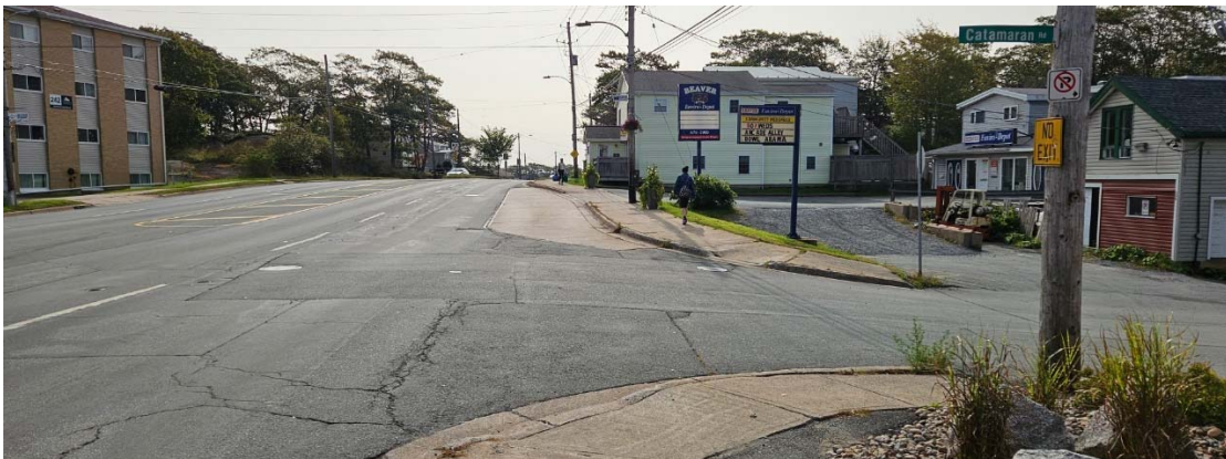
Herring Cove Road at Catamaran Road looking south
