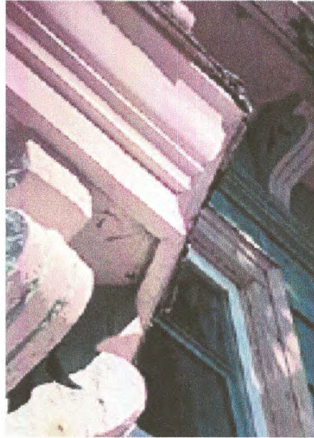
Fig. 33 Wood work will be scraped and repainted if not rotten or replaced using the original patterns.
