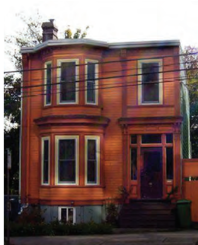
Fig. 12 Showing a remaining example of Halifax Box 5516 North St.
