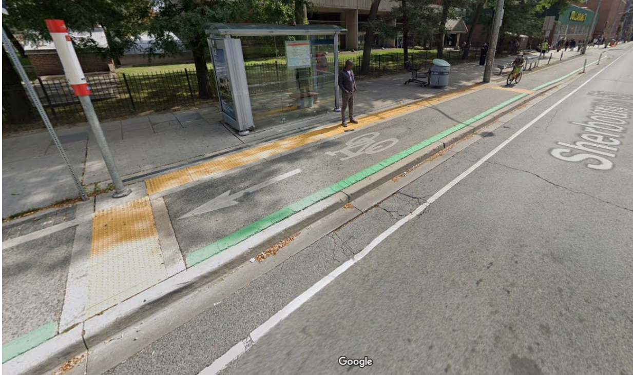
Figure 21: Example of an "integrated bus stop" in Toronto
