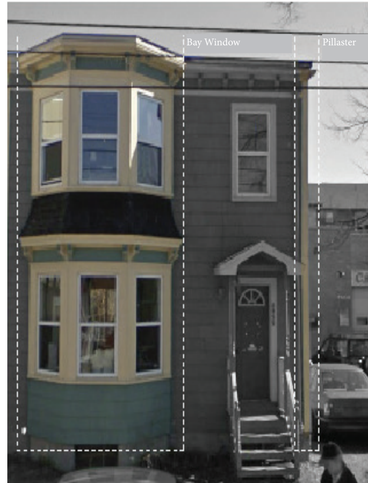
Fig. 14 Vertical Elements Showing characteristics of the Halifax Box style.
