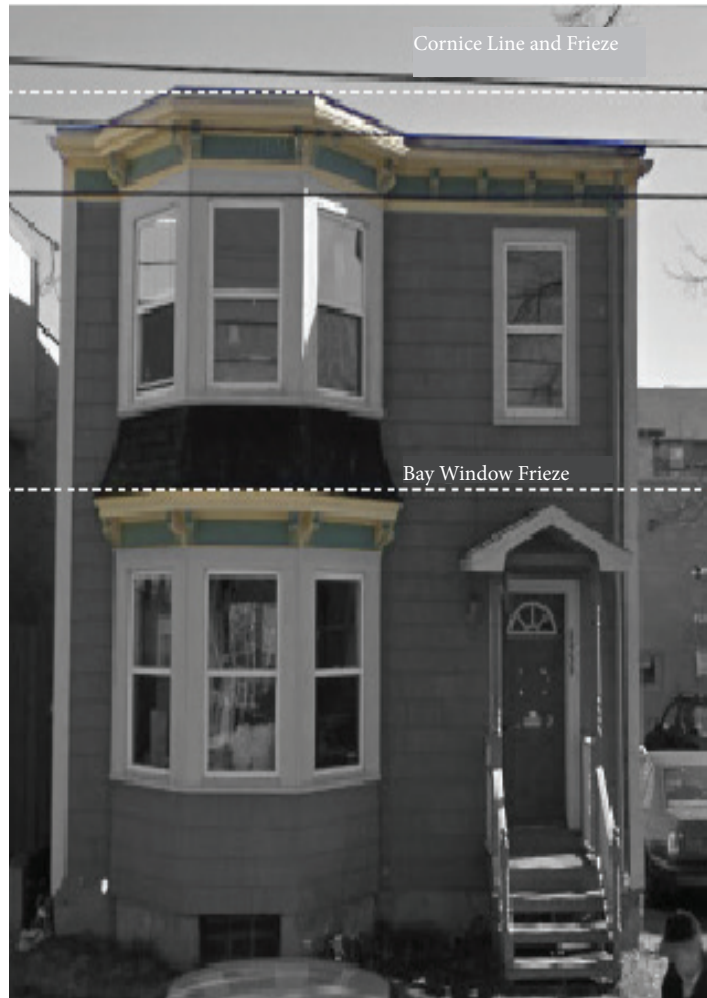
Fig. 13 Horizontal elements showing characteristics of the Halifax Box style. The frieze features ornamental cornice brackets to accentuate the roof lines.
