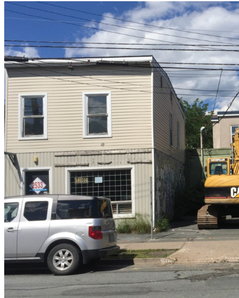
Fig. 8 Former Halifax box at 2533 Agricola St “Nauss Bicycle” demolished to build Compass Pag.9
