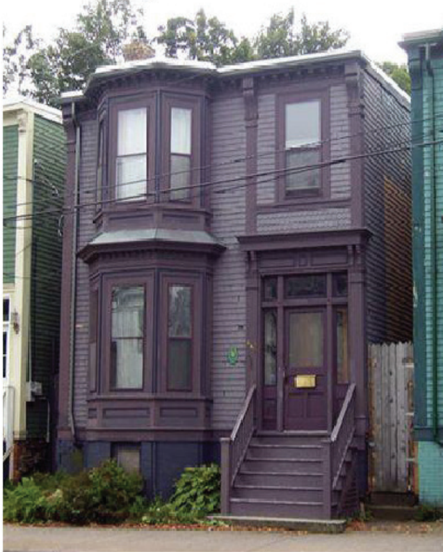
Fig. 11 Showing a remaining example of Halifax Box 2548 Gottingen St.
