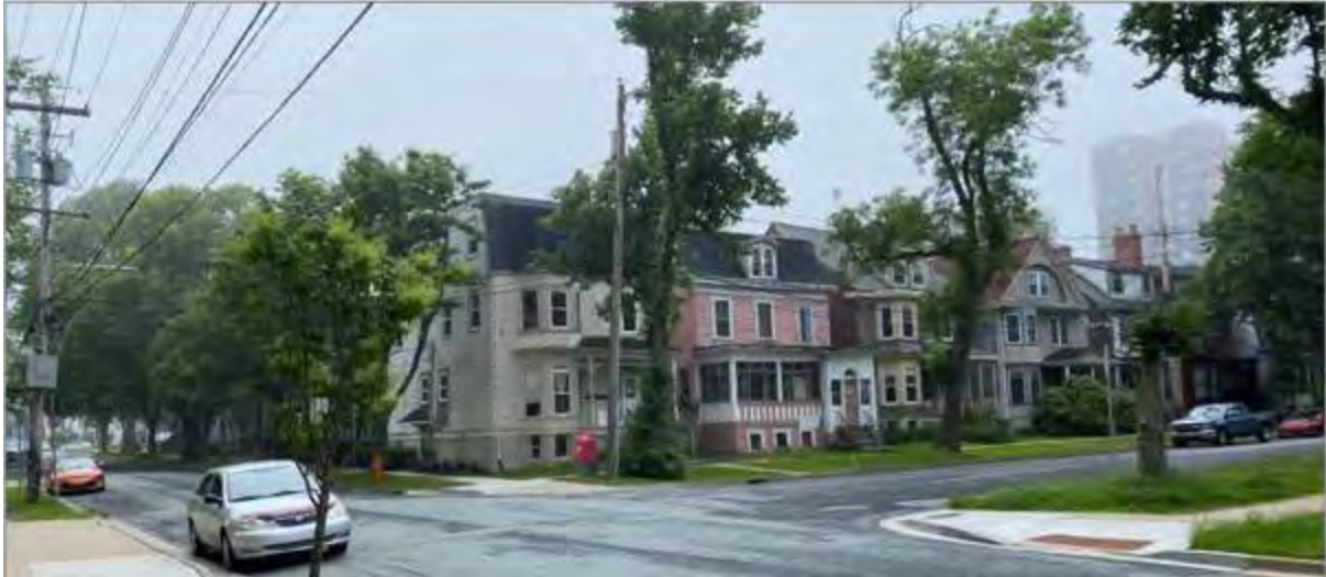
Some of the houses in the Carlton Block that would be demolished to make way for new highrises if the HRM Council approves the development project. (Photo: Heritage Advisory Committee) 21
