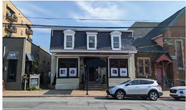
L2) 62 OCHTERLONEY ST - INTERLUDE SPA (COMMERCIAL)
