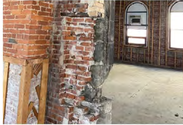
BMR Photo 4.4.B: Damaged load-bearing masonry below west end of steel header beam at 1947 addition opening (28 Feb 2022).
