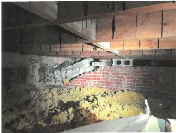
Photo No. 23 – Remaining Clock Tower base masonry visible in attic space.
