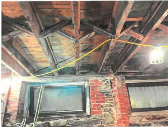
Photo No. 11 – View of 1914 main floor joists supported on wood lintel over window opening.
