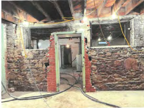
Photo No. 25 – Pier removal at door opening.
