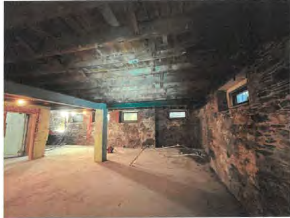
Photo No. 10 – View of 1914 basement masonry walls and wood framing overhead. Interior support girders and concrete encased columns visible.
