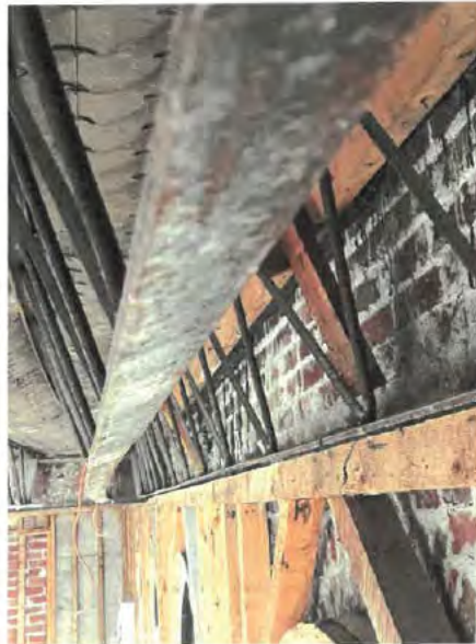
Photo No. 28 – Bend in 1947 roof joist.
