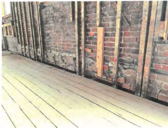
Photo No. 24 – Base of exterior wall at Second Floor. Masonry infill over steel lintel framing over west wall openings through 1914 building.
