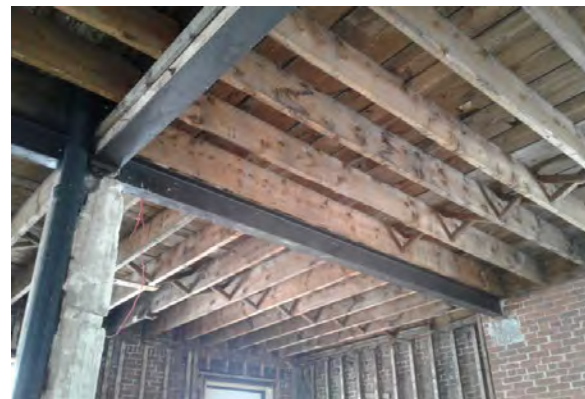
BMR Photo 4.2.D: 2"x10" timber joists supported on steel girder beams and concrete-encased W-columns (28 Feb 2022).
