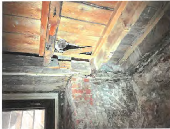
Photo No. 12 – Detail at basement window lintel with notched floor joists. Note ledger strips and forms supporting concrete infill between floor joists. Terrazzo floor topping above this area.
