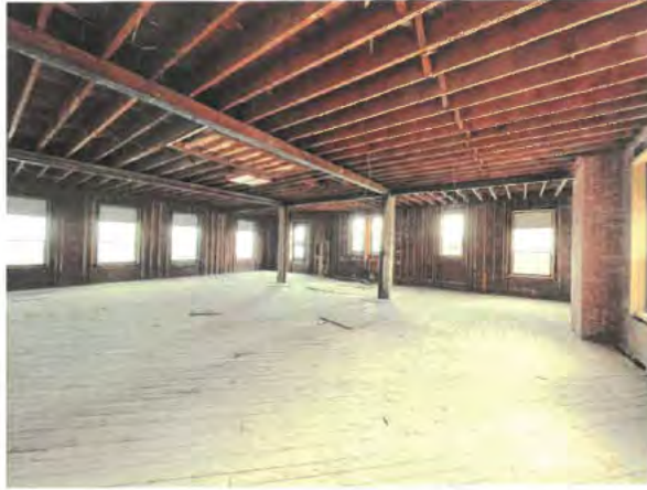
Photo No. 17 – Second floor of 1914 block with ceiling and roof support joists visible. Steel girders and concrete encased columns visible.
