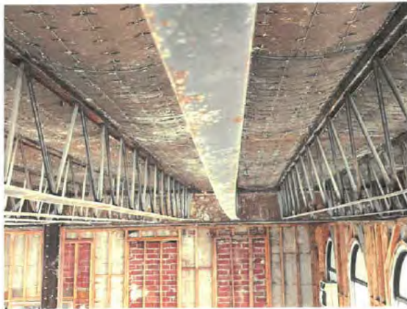
Photo No. 27 – Close view of 1947 roof joist.
