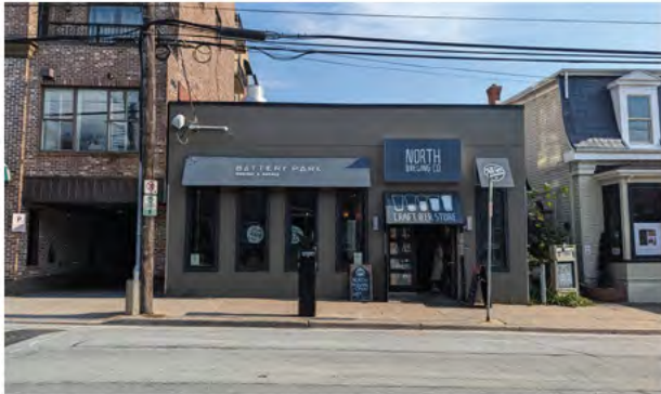
L1) 58 OCHTERLONEY ST - BATTERY PARK (COMMERCIAL)
