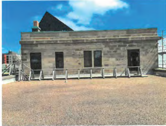
Photo No. 2 – West Elevation above 1961 addition roof.
