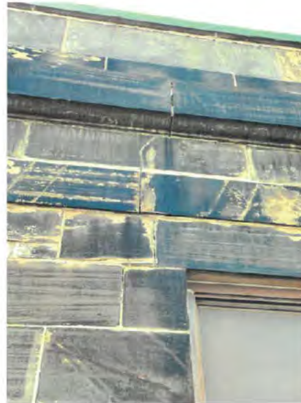
Photo No. 4 – North Elevation – Crack in sandstone above window jamb. Mortar missing in some joints.
