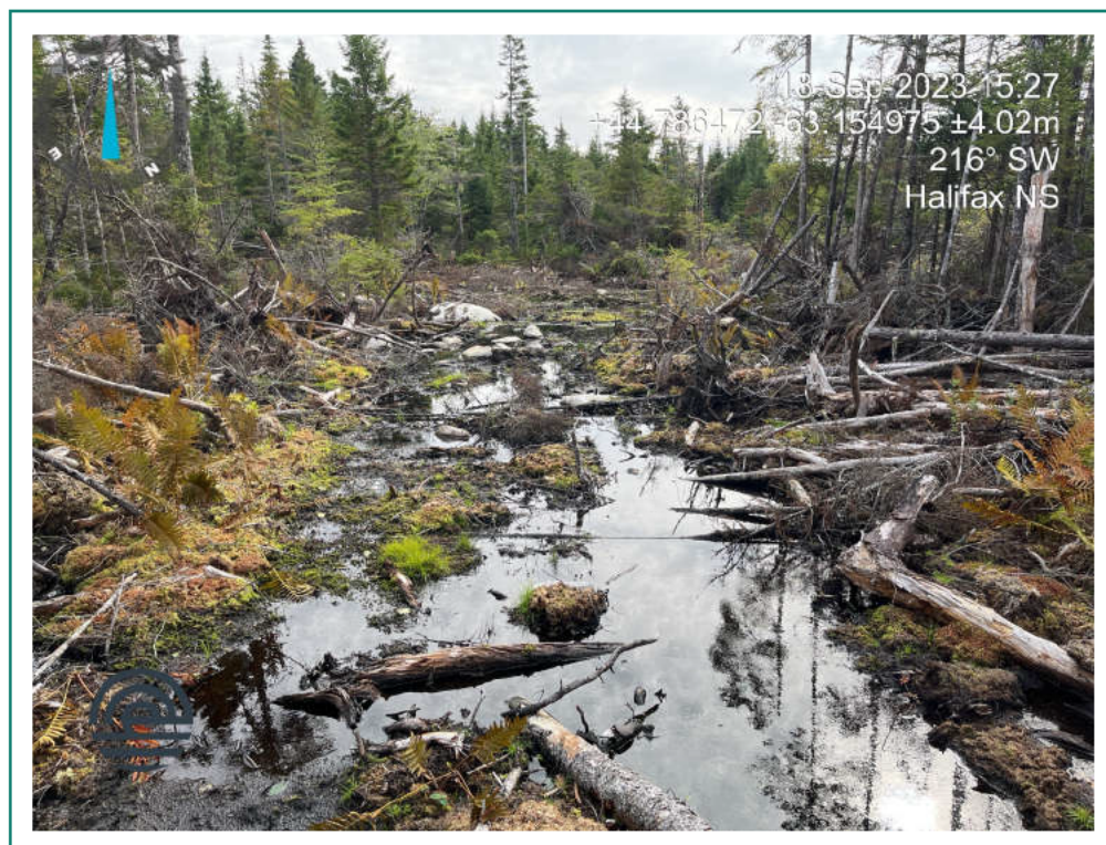
Photo 2: Wet area, significantly disturbed due to previous geotechnical test pit investigation. Photo taken in the central /northwest portion of the property where geotechnical machinery has made depressions in the landscape which hold water. Adjacent undisturbed areas did not appear to be wetland.
