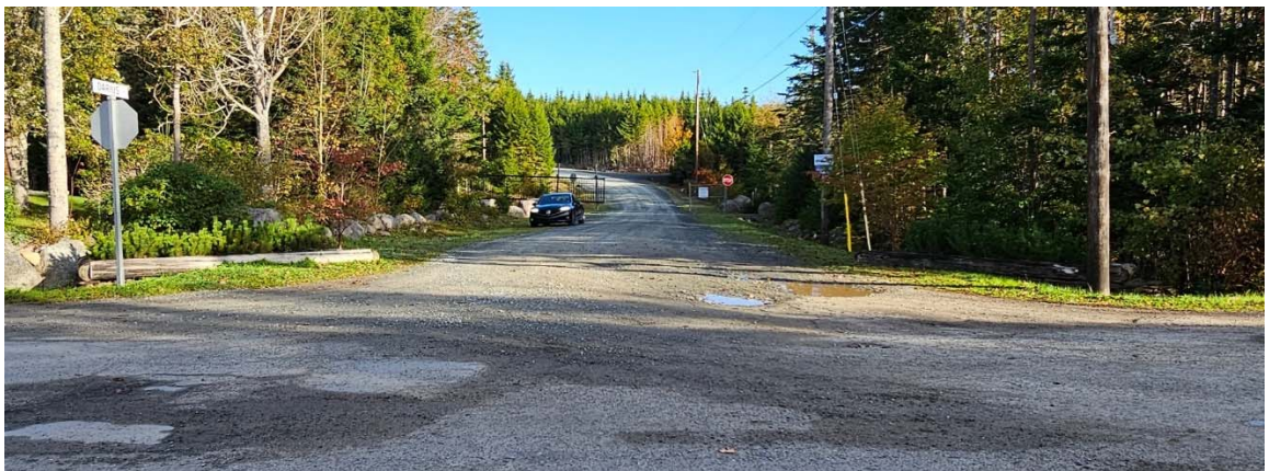
Darius Lane at Little River Drive looking north
