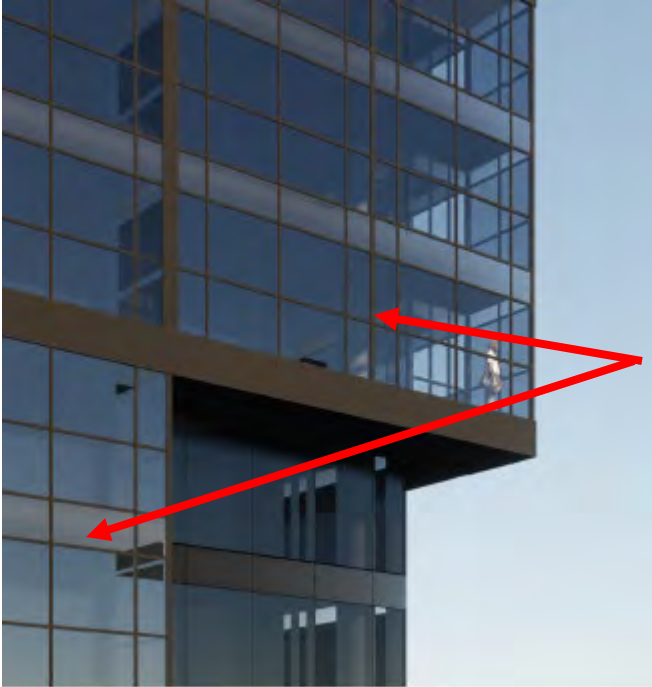
Figure 5: Signature architectural projections identified by red arrows
