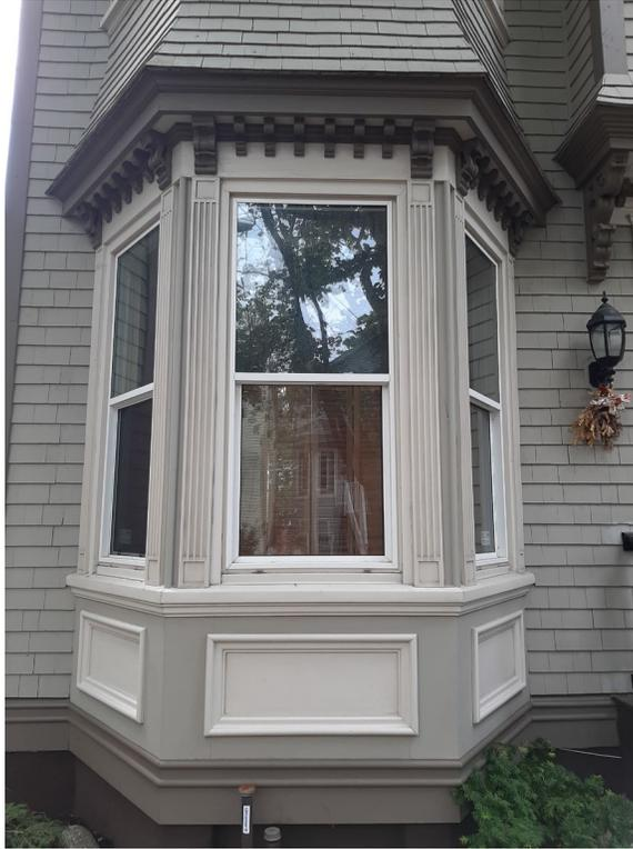
Figure 13: Two-storey Bay window with paneling, wood piers and bracket and corbel detailing on the north elevation (Staff photo, 16 June 2023)
