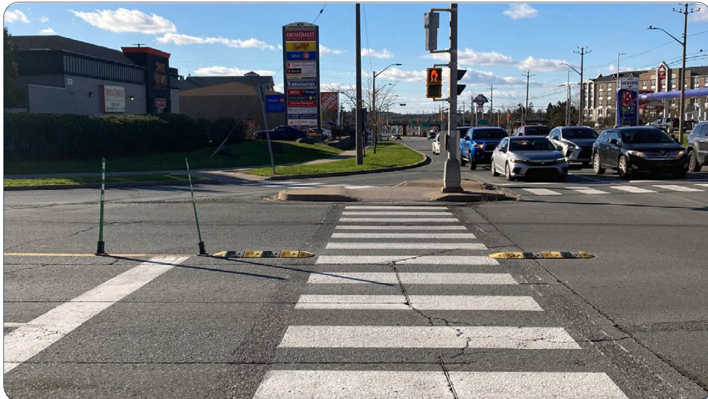
FIGURE 14: LEFT TURN CALMING AND HIGH VISIBILITY CROSSWALK MARKINGS AT LACEWOOD DRIVE AND PARKLAND DRIVE, REGENCY PARK DRIVE, 2022
