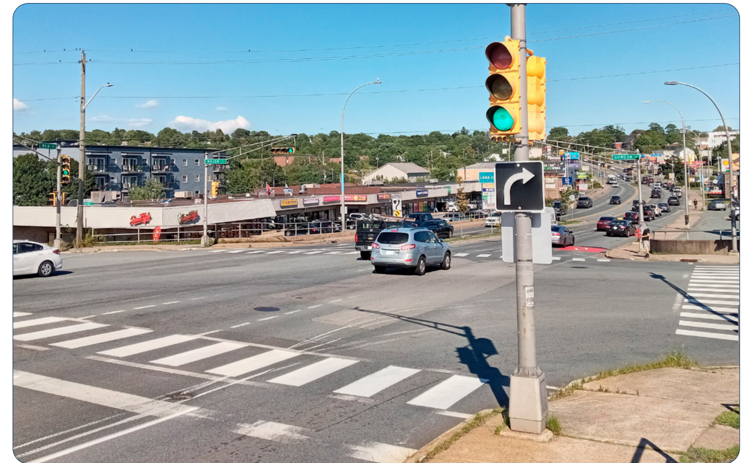
FIGURE 13: HIGH VISIBILITY CROSSWALK MARKINGS AT MAIN STREET AND MAJOR STREET, 2022 ✓
