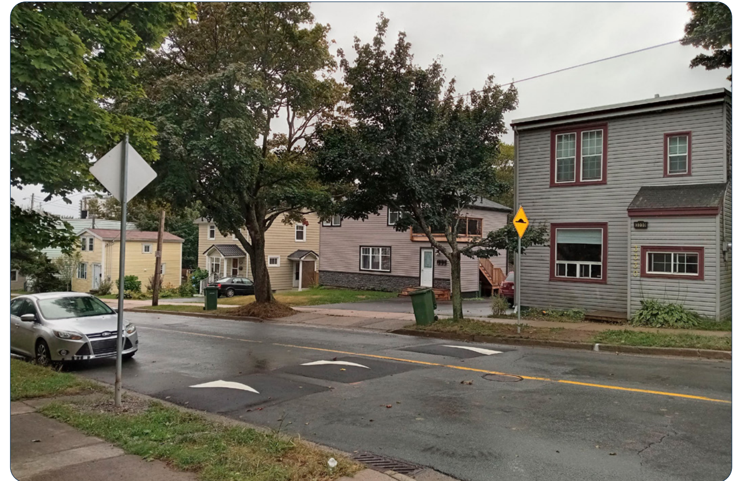
FIGURE 17: SET OF SPEED CUSHIONS ON ROBIE STREET, 2022 ^
