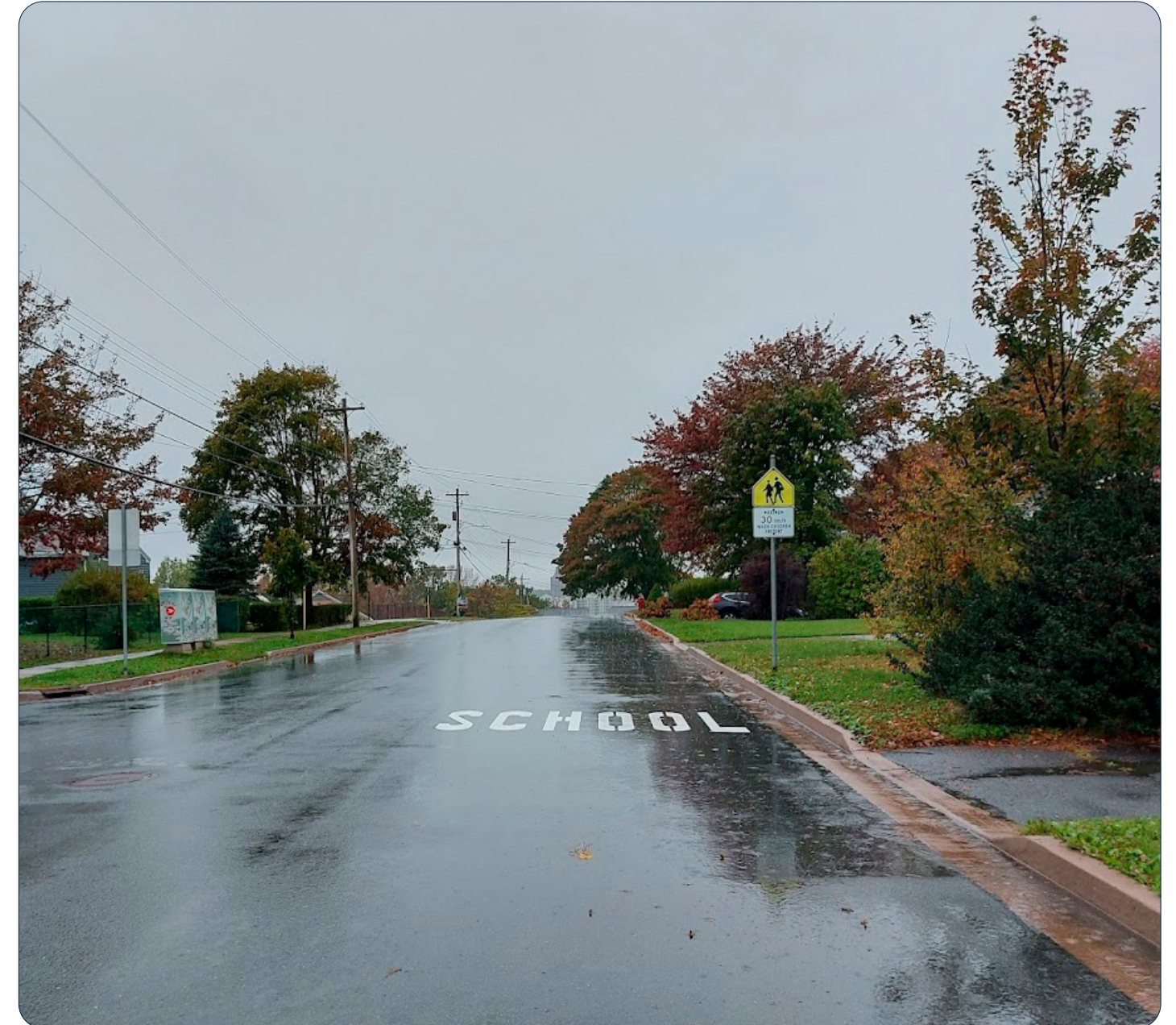
FIGURE 15: PAINTED 'SCHOOL' MARKINGS, PILOT ON PENHORN DRIVE, 2022
