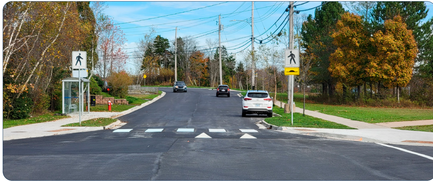
FIGURE 18: RAISED CROSSWALK INSTALLED ON AUBURN DRIVE, 2022 ^
