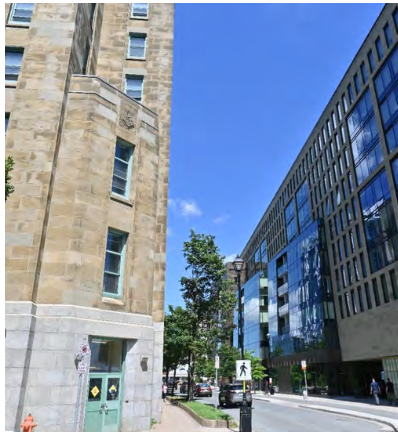
2. The new building on the right incorporates high quality materials that relate, and respond, to the heritage building on the left.
