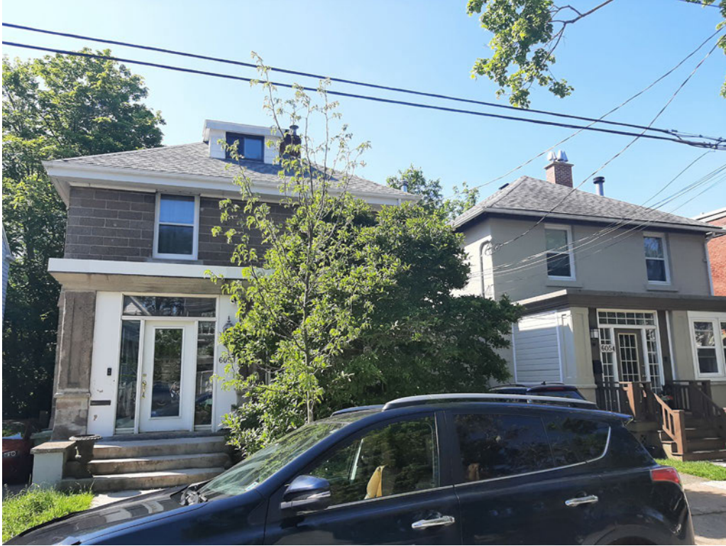
Figure 26: Concrete block homes on Cedar Street (16 June 2023)
