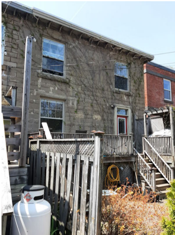
Figure 19: East elevation (19 May 2023)
