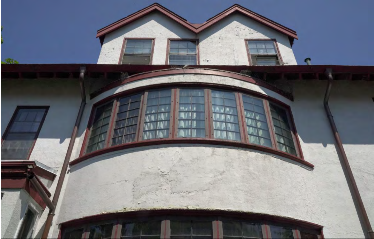
Figure 21: Detail of rear bay window (Jun. 22, 2023)
