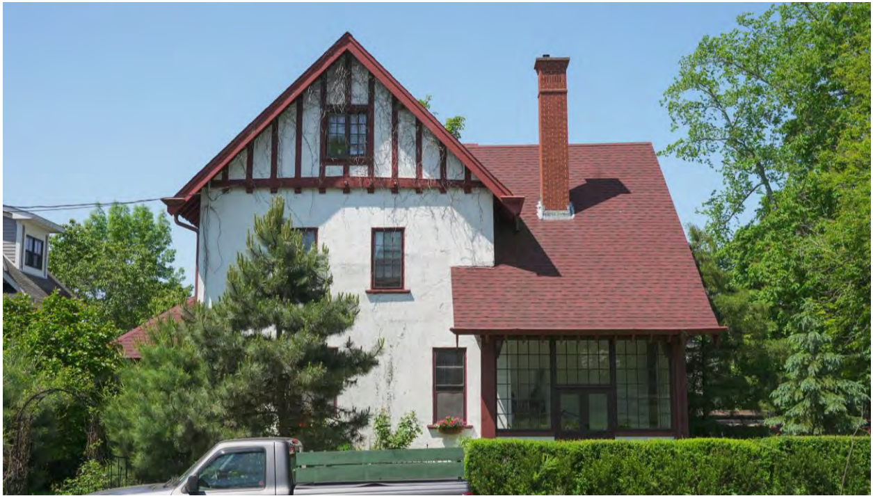
Figure 16: Eastern elevation (Jun. 22, 2023)
