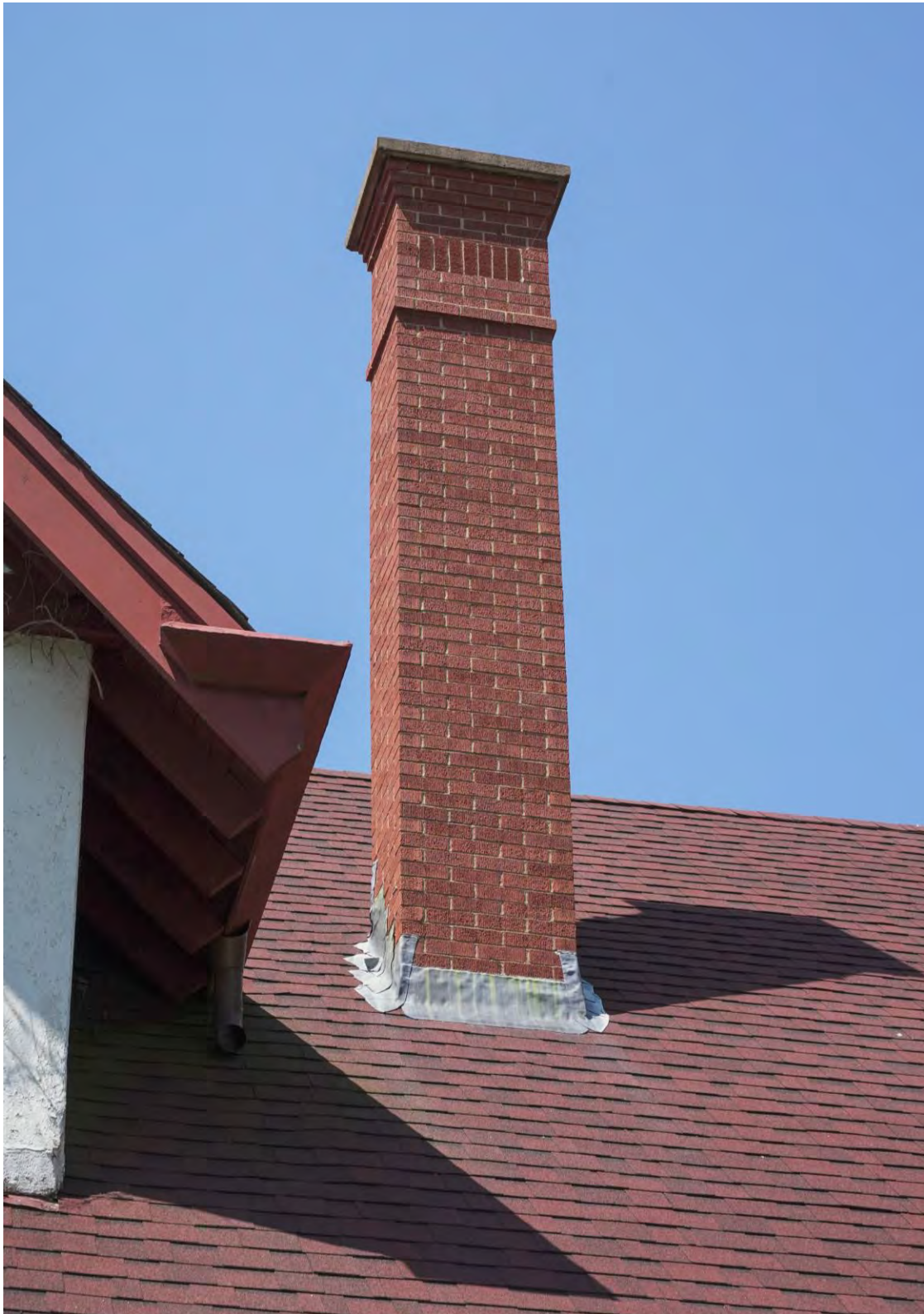
Figure 23: Detail of Chimney (Jun. 22, 2023)
