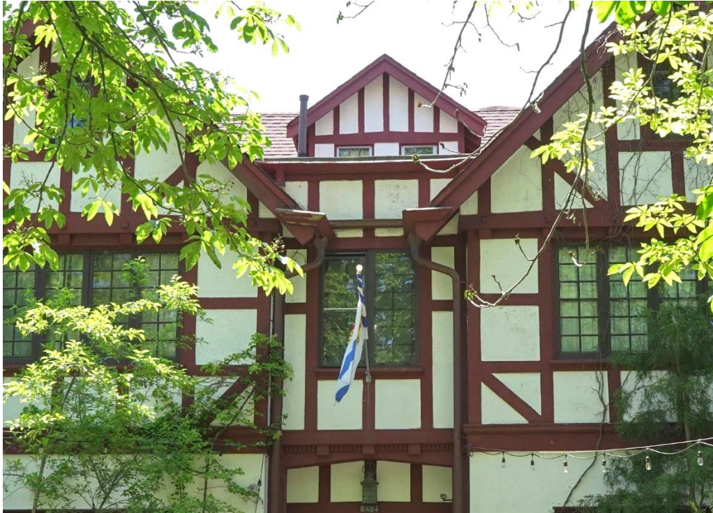
Above: Close-up of faux half-timbering on the front elevation
