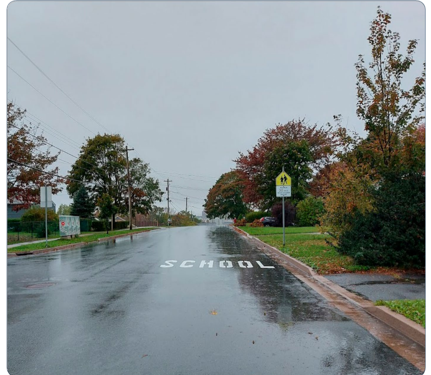
FIGURE 15: PAINTED 'SCHOOL' MARKINGS, PILOT ON PENHORN DRIVE, 2022
