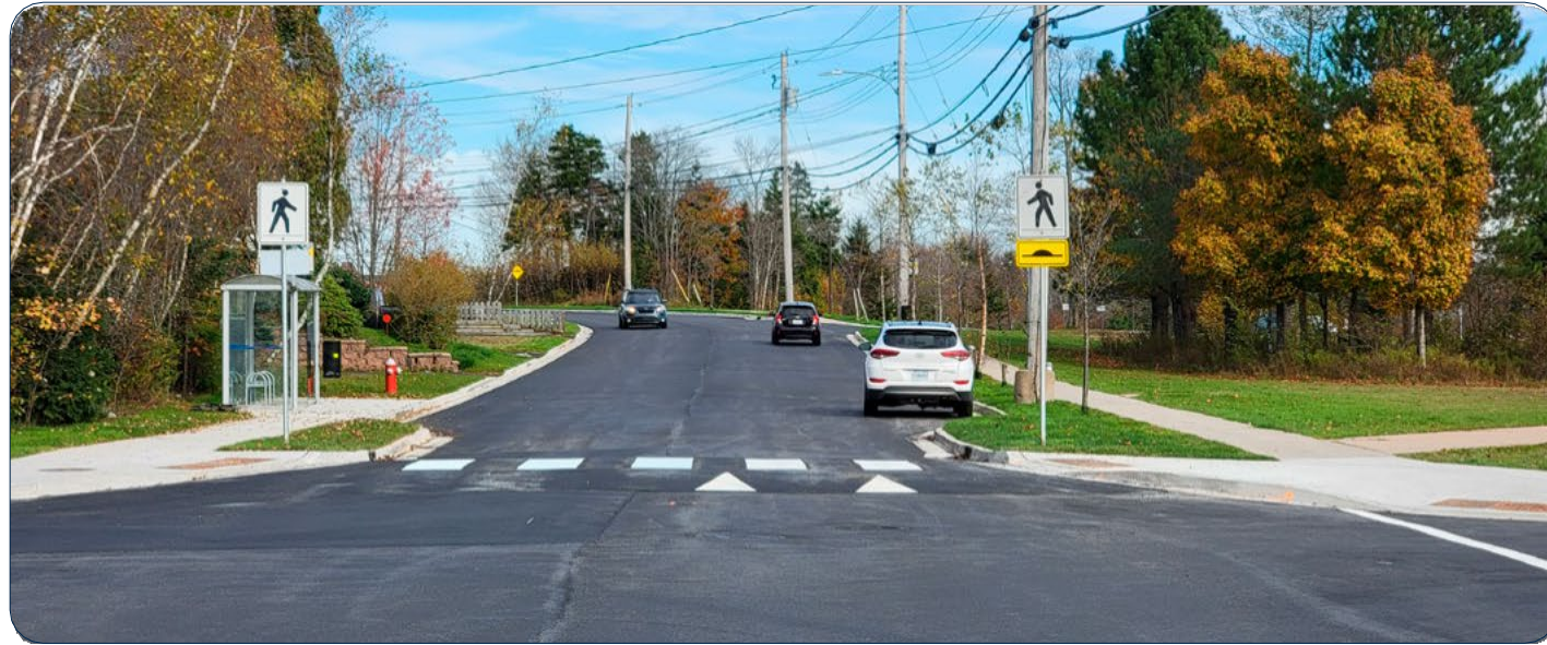
FIGURE 18: RAISED CROSSWALK INSTALLED ON AUBURN DRIVE, 2022 ^
