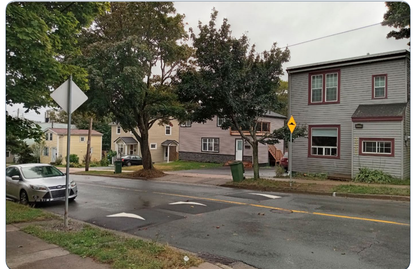
FIGURE 17: SET OF SPEED CUSHIONS ON ROBIE STREET, 2022 ^
