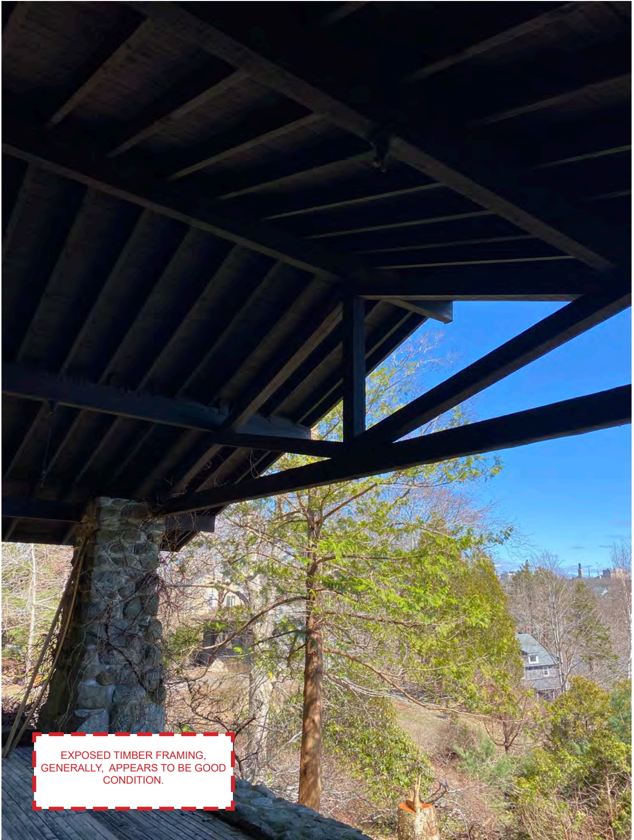
2.8 EXPOSED WOOD FRAMING AT COVERED PORCH (EAST SIDE).
