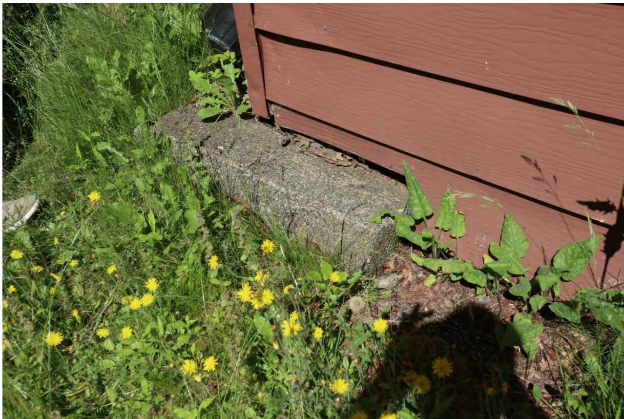
As is evident in the above photograph, the building is resting directly on the footing. Being on the surface of the ground, this footing has visible cracking.
