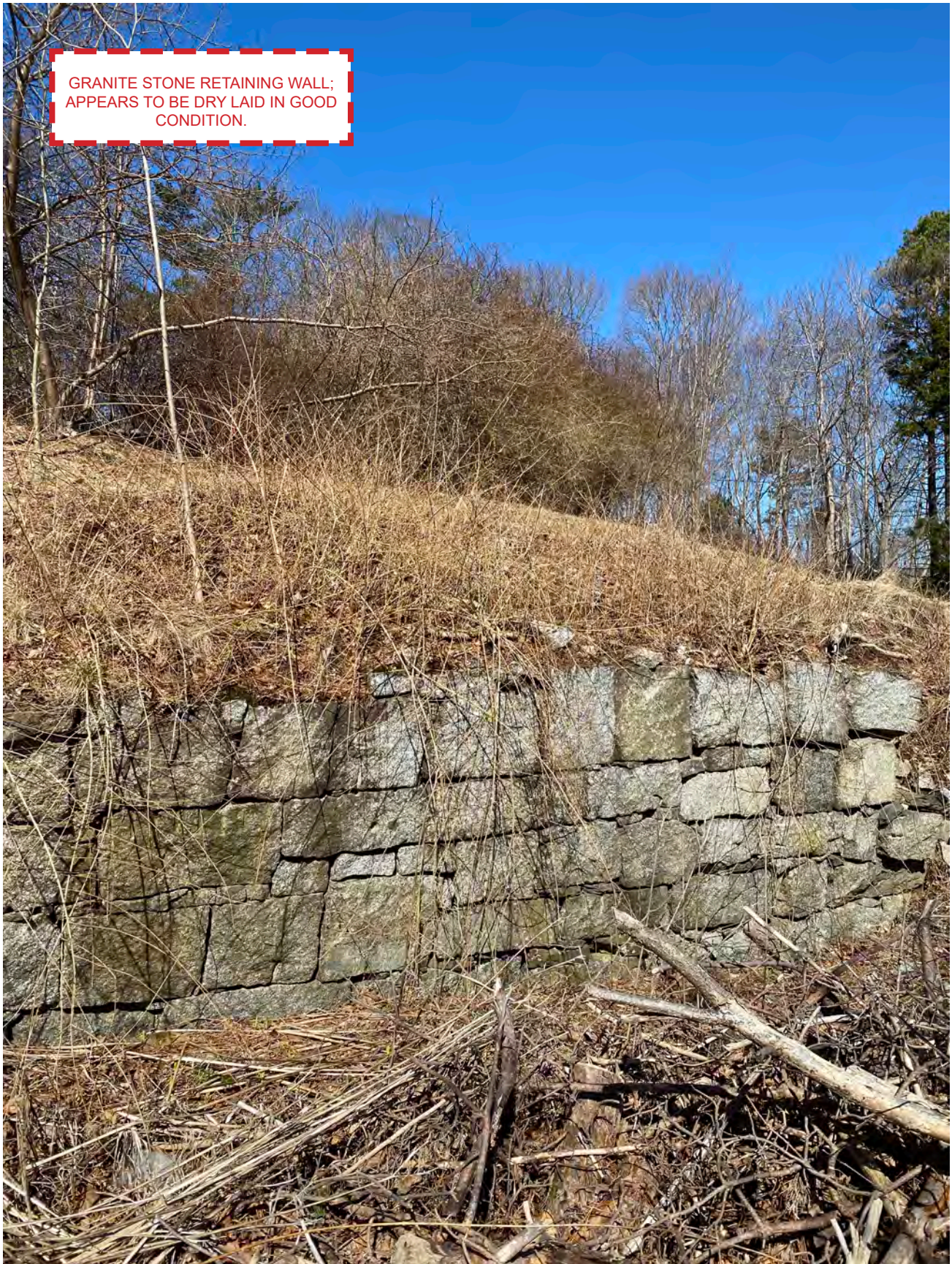
2.27 STONE WALL; SOUTH OF MAIN HOUSE (NORTH VIEW).
