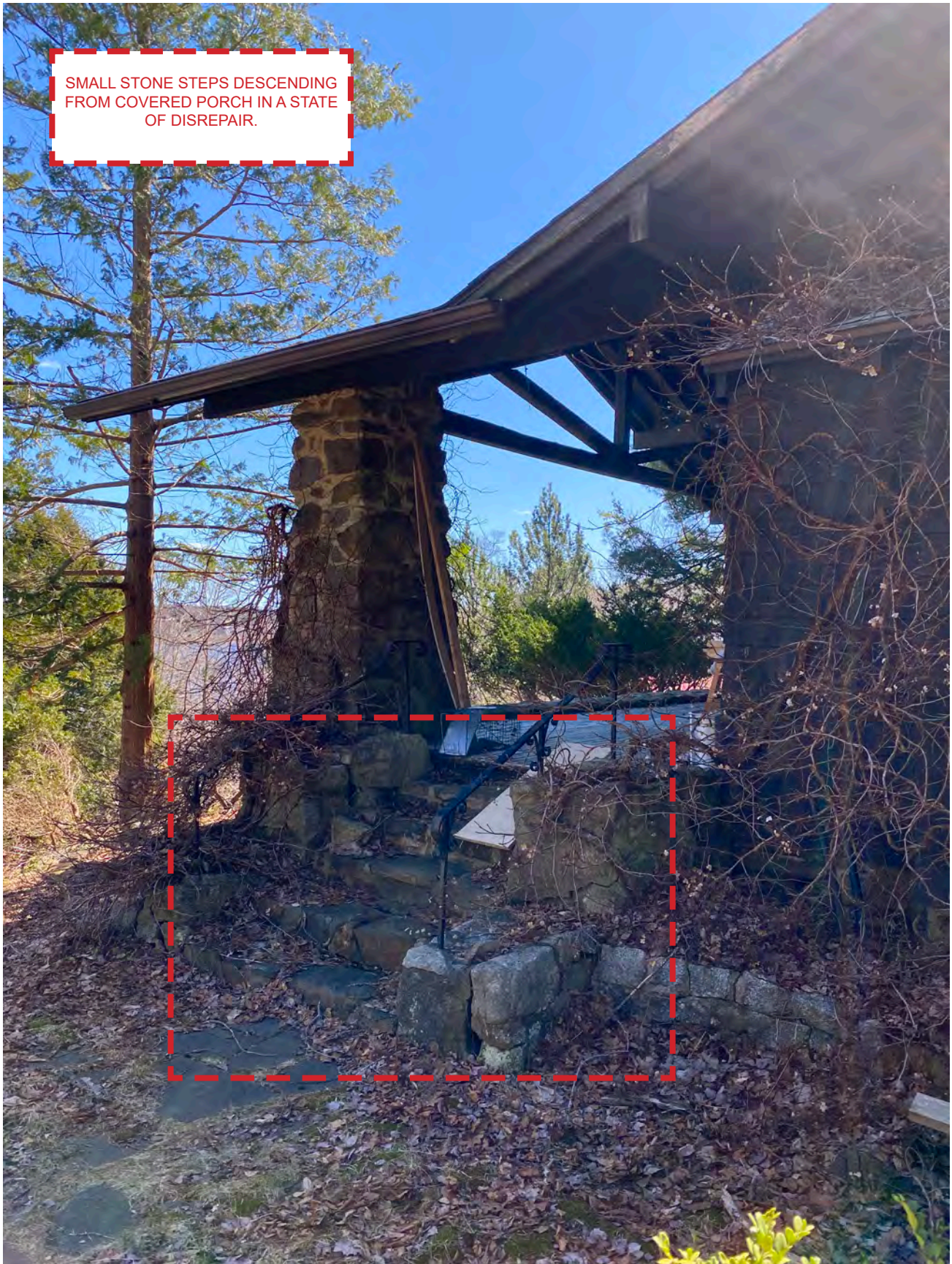
2.10 SMALL STONE STEPS LEADING TO COVERED PORCH (NORTH SIDE).
