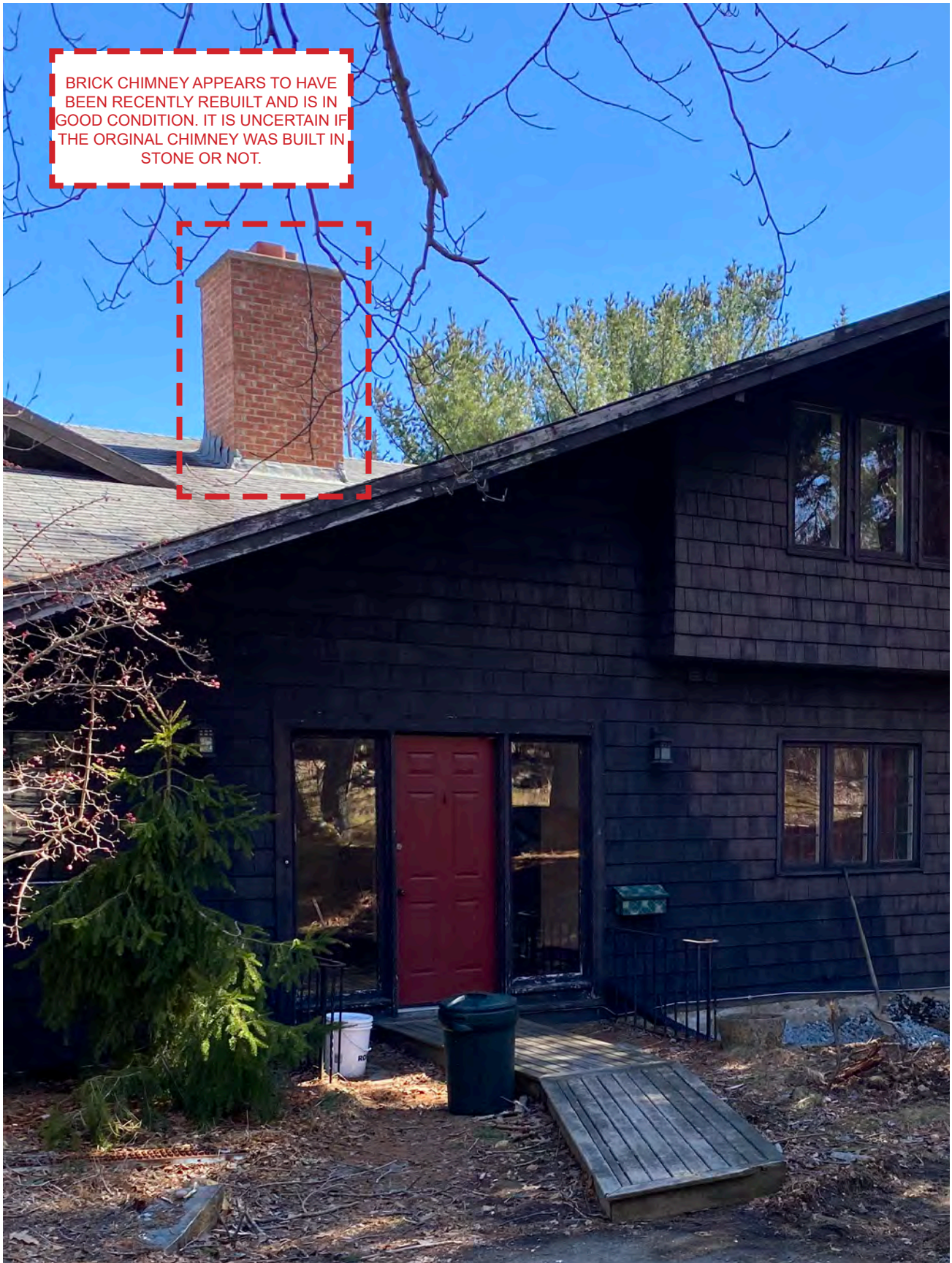
2.11 MAIN ENTRY AT WEST SIDE.
