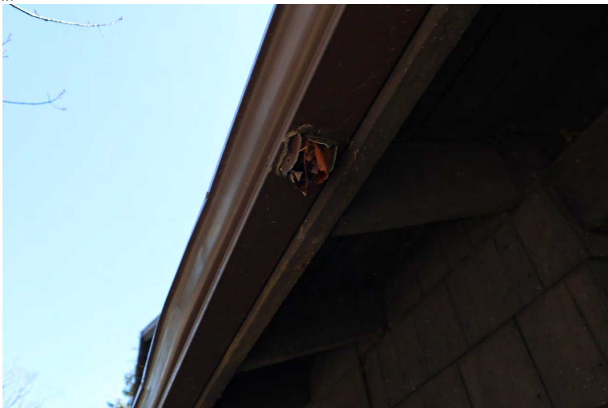
3) The gutters and downspouts were another item in very bad condition. See sample of damages in photograph below.
