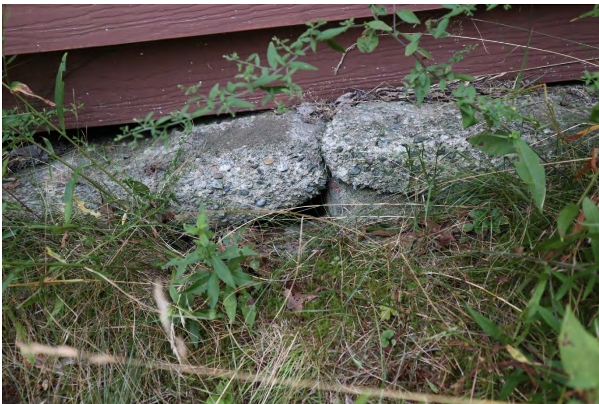
As is evident in the above photograph, the building is resting directly on the footing. Being on the surface of the ground, this footing has visible cracking.
