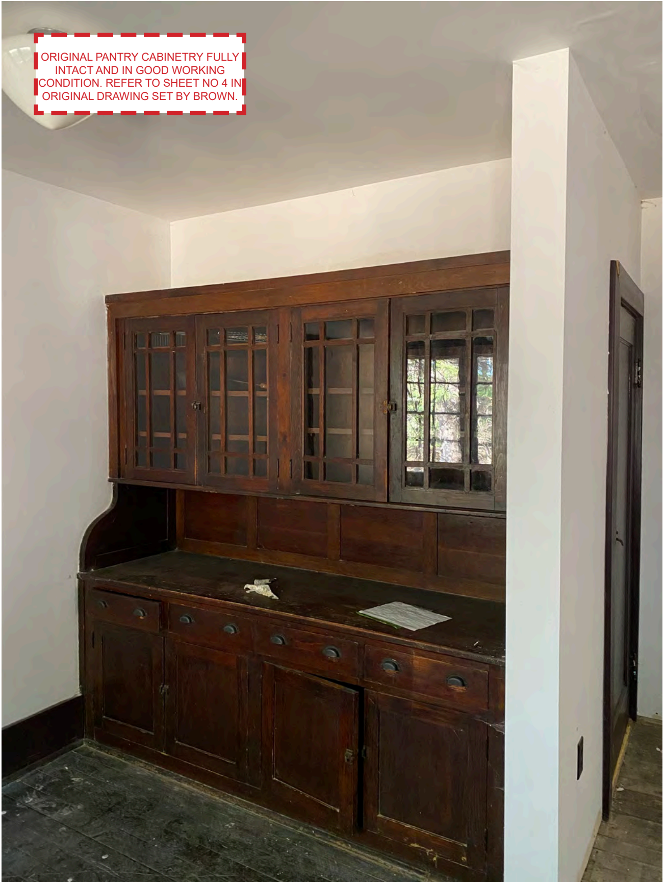
2.13 MAIN FLOOR PANTRY AREA (OPPOSITE DINING AREA).
