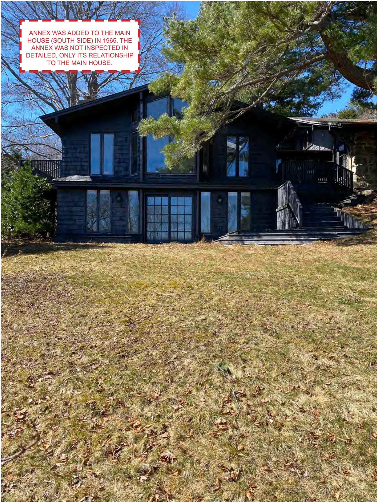
2.21 ANNEX (EAST SIDE).
