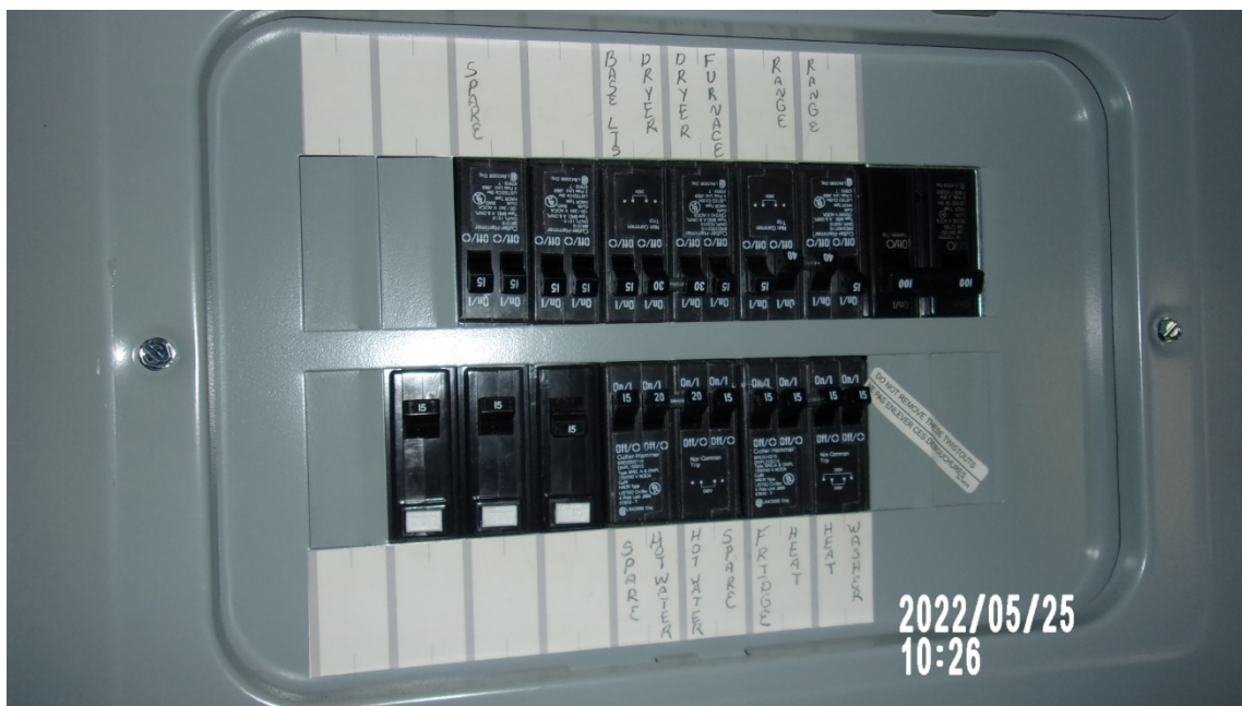
E4- Cutler-Hammer Electrical Load Centre, 16 Circuit Capacity with a 100A Main Breaker
