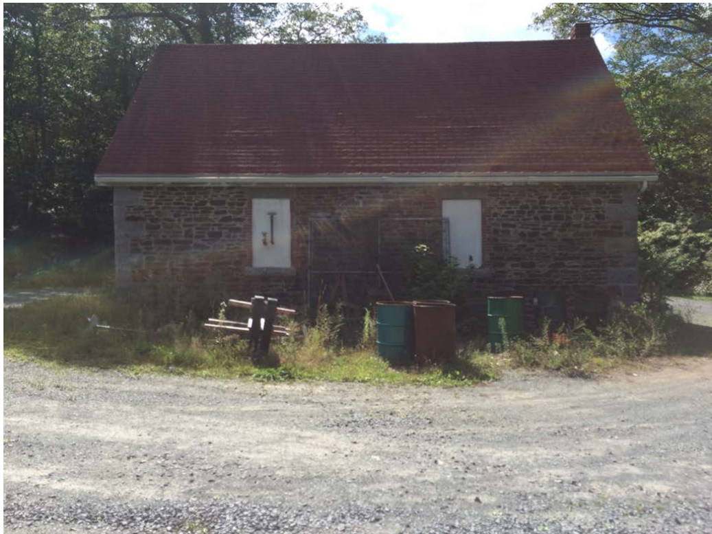
Figure 17 East elevation of barn
