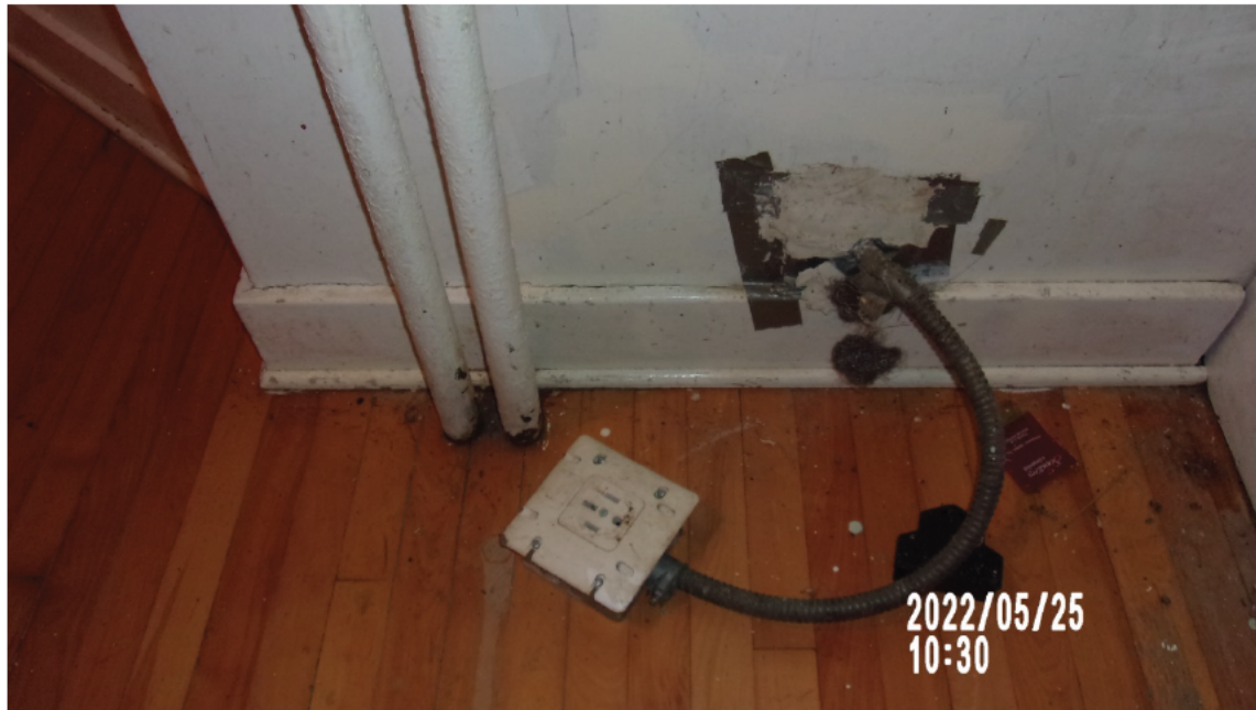
E7- Typical Ungrounded Receptacle.
