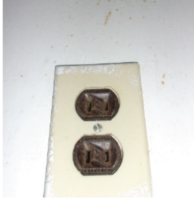
E7- Typical Ungrounded Receptacle.
