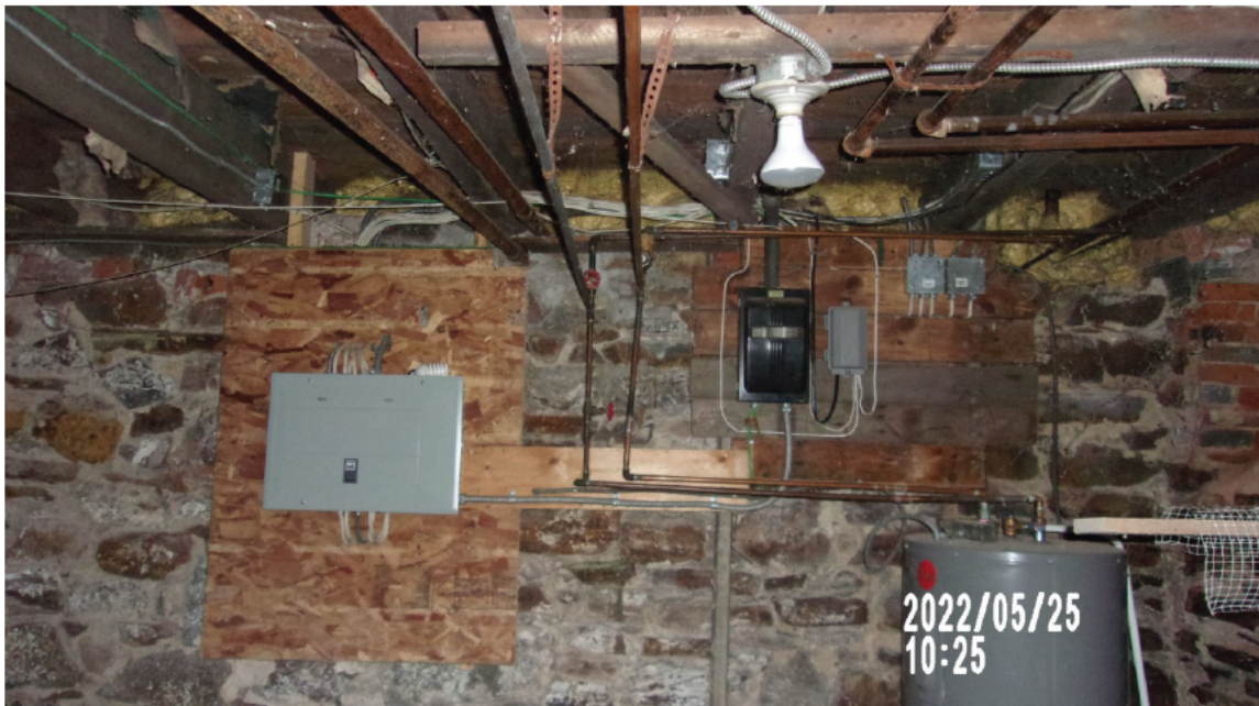
E2- Electrical Service Entrance Equipment
