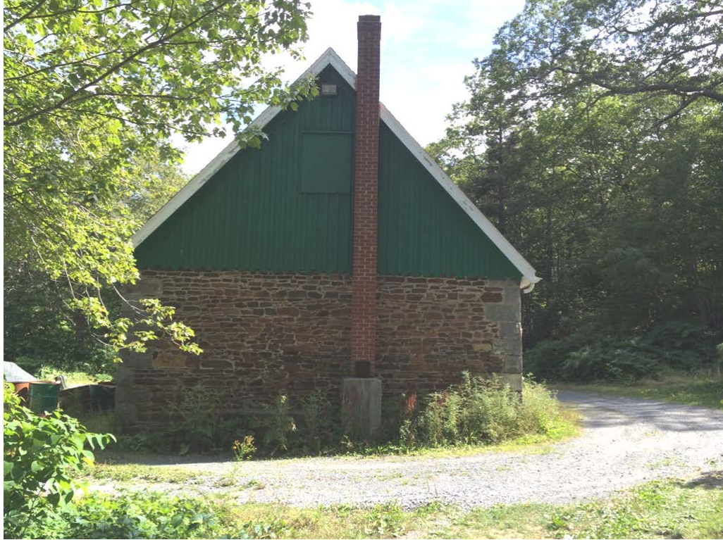
Figure 16 North elevation of barn
