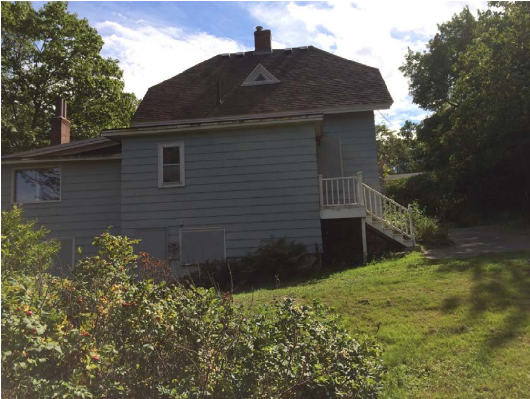
Figure 10 East addition viewed from north
