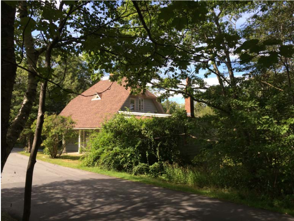
Figure 11 East addition viewed from south - note second floor windows
