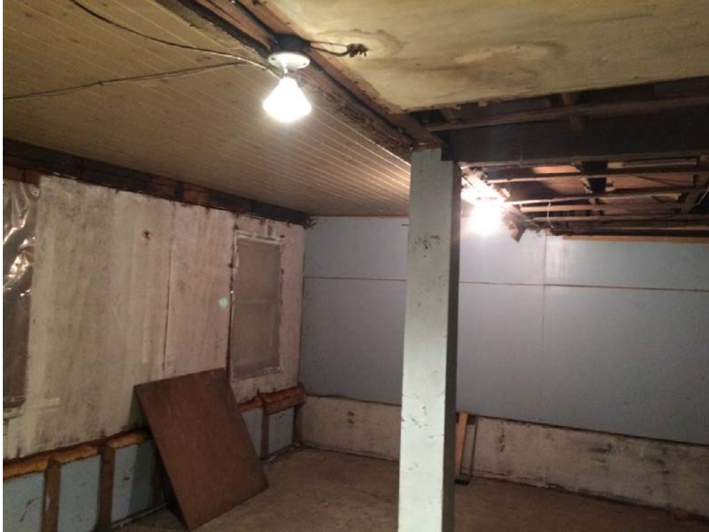
Figure 13 Basement of east addition
