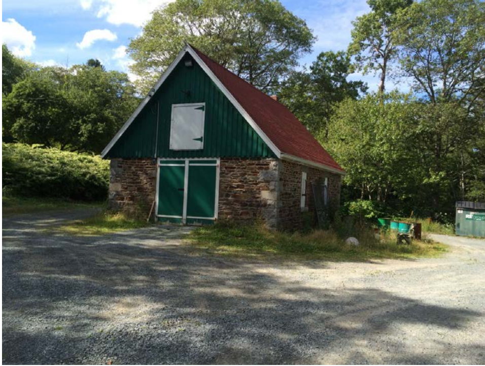
Figure 14 South elevation of barn
