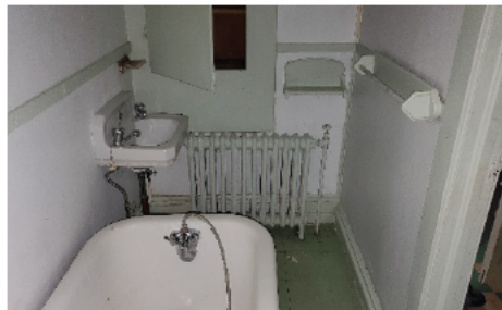
M3: Original Plumbing Fixtures.
