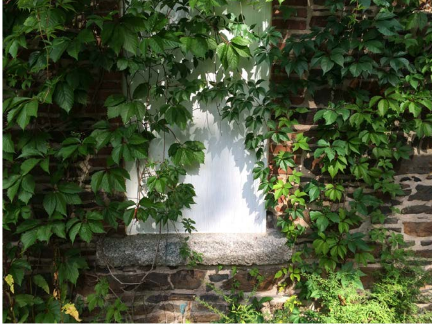
Figure 7 Ironstone foundation of original cottage
