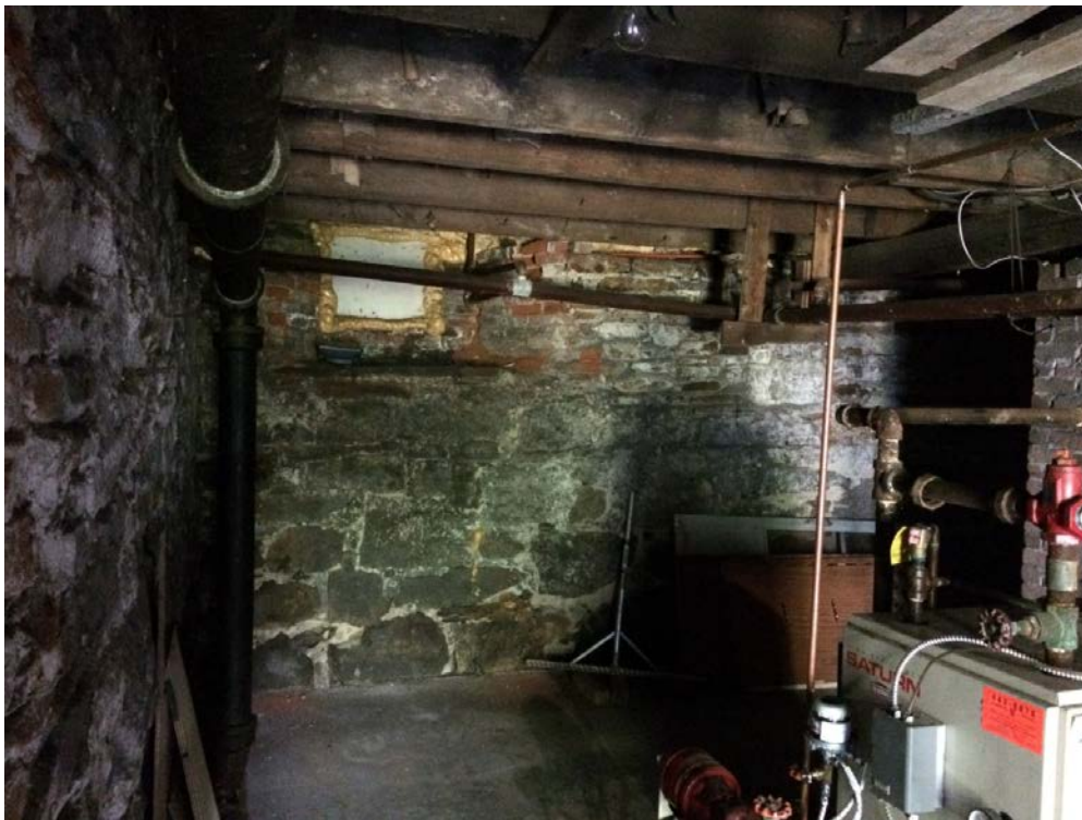
Figure 12 Ironstone foundation under original cottage
