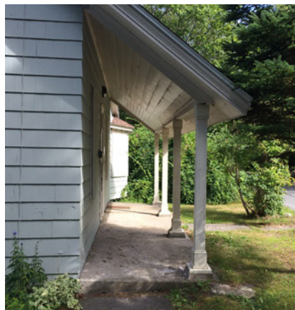
Step onto concrete porch
