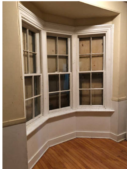
Original windows in kitchen
