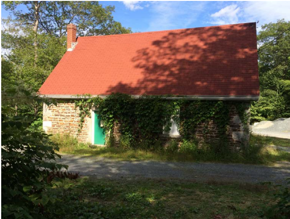
Figure 15 West elevation of barn
