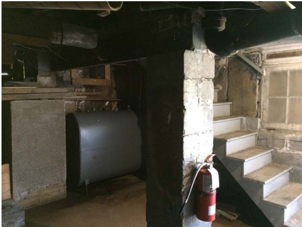
Figure 24 Stairs to basement
