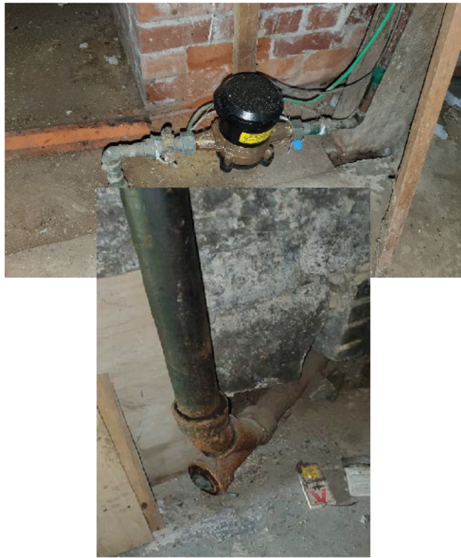
M1: Water Entrance
