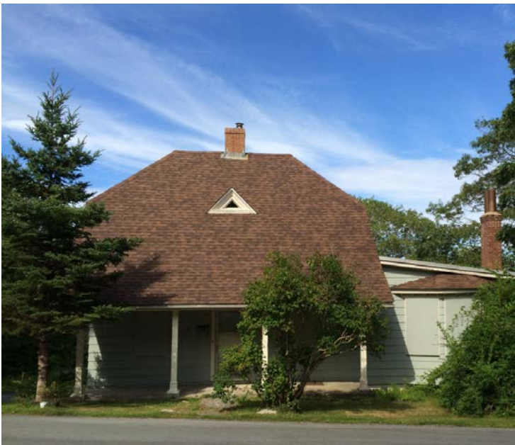
Figure 26 Cottage is very close to road
