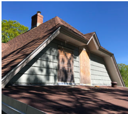
Asphalt shingle roof and modified bitumen roof
