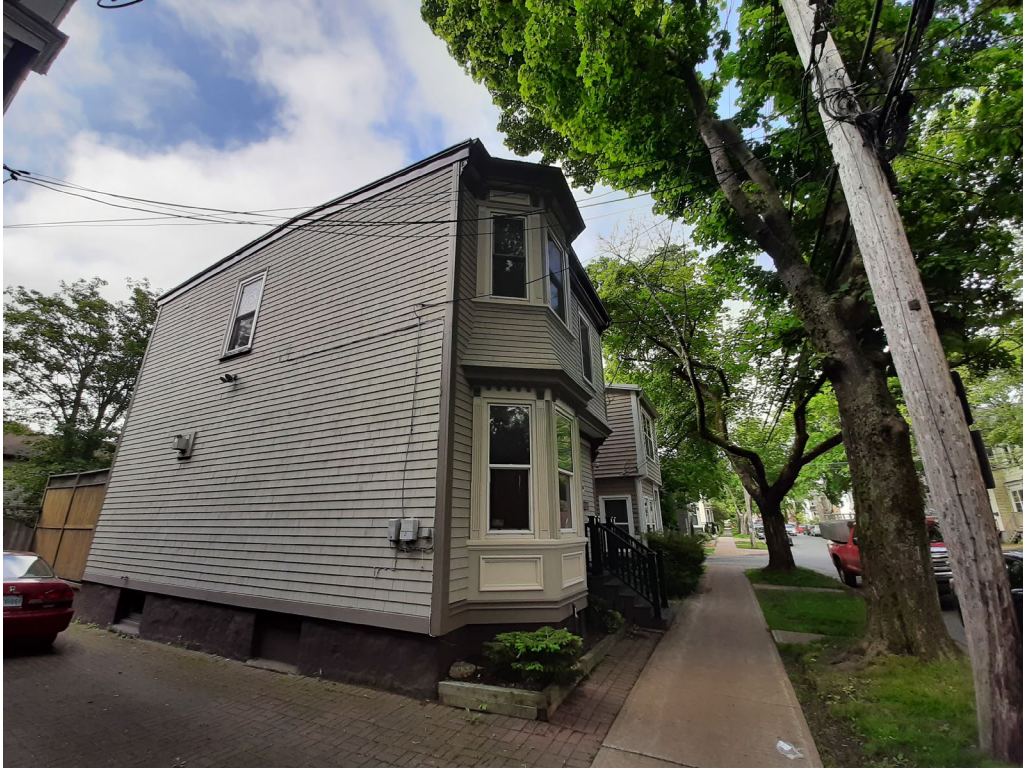
Figure 11: East elevation (Staff photo, 16 June 2023)
