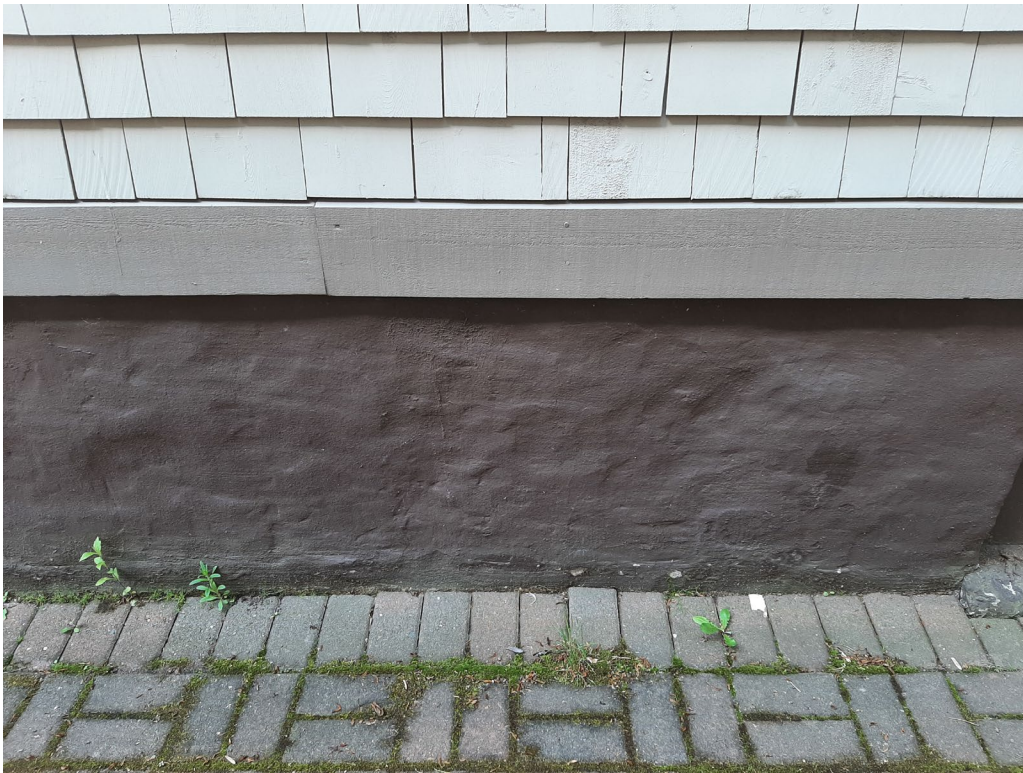
Figure 12: Foundation of 6038 Charles Street, showing concrete parging (Staff photo, 16 June 2023)
