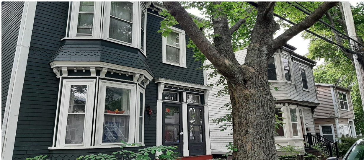
Figure 5: View of 6032-6034, 6038 and 6040 Charles Street from the east side of Charles Street (Staff photo, June 16, 2023)
