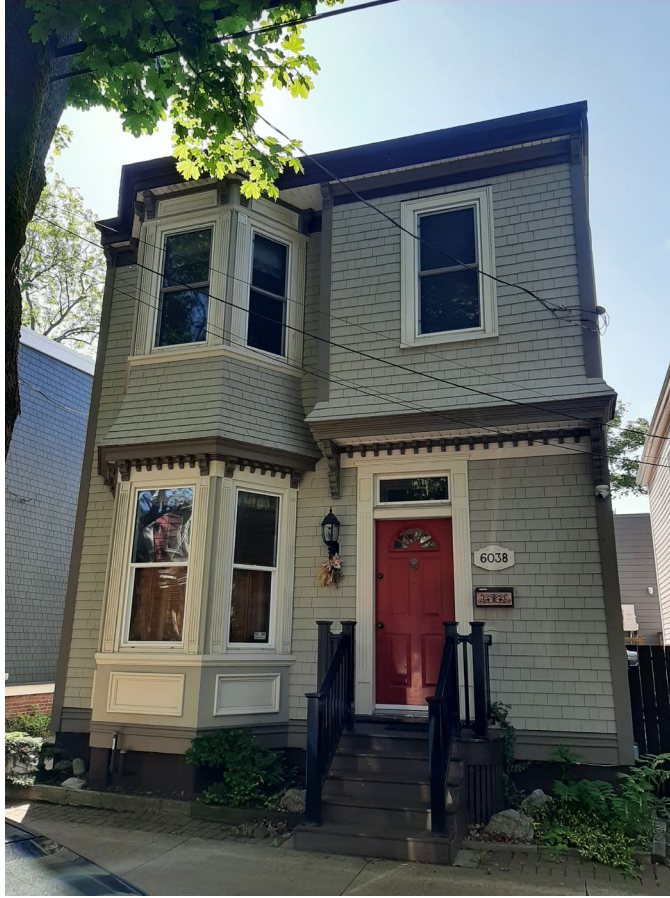
Figure 8: North elevation of 6038 Charles Street (Staff photo, 16 June 2023)
