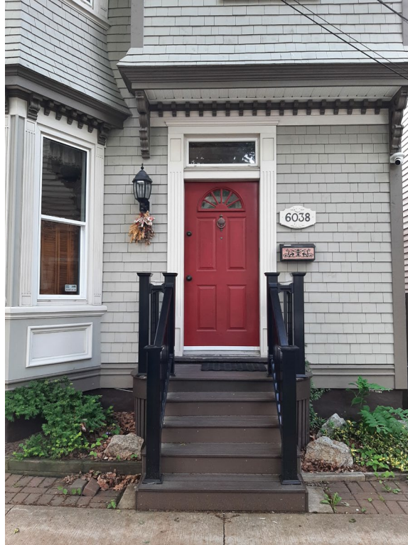
Figure 15: Main entrance to 6038 Charles Street, with wood piers and transom (Staff photo, 16 June 2023)
