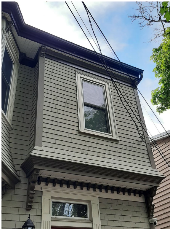
Figure 14: Second storey protruding square bay (Staff photo, 16 June 2023)
