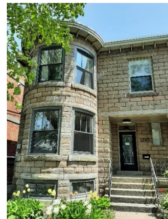
Figure 2: West elevation of 1745 Henry Street (Staff photo, 19 May 2023)
