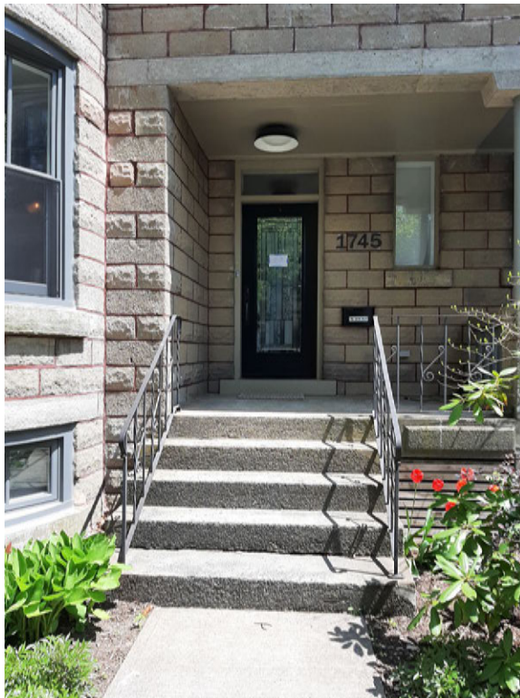
Figure 21: Main entrance and stairs of 1745 Henry Street (19 May 2023)
