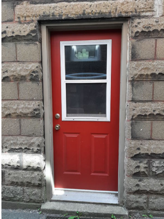
Figure 20: Basement entrance on the north elevation (19 May 2023)
