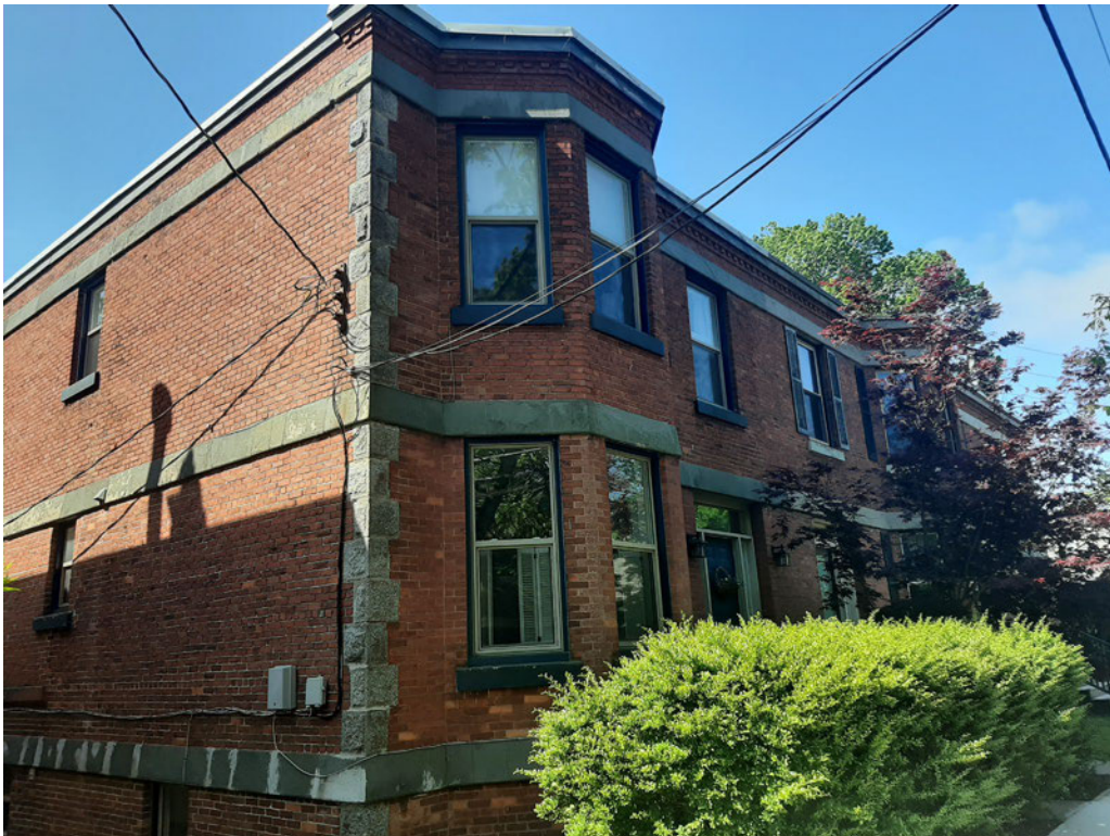
Figure 27: Brick homes on Cedar Street (16 June 2023)
