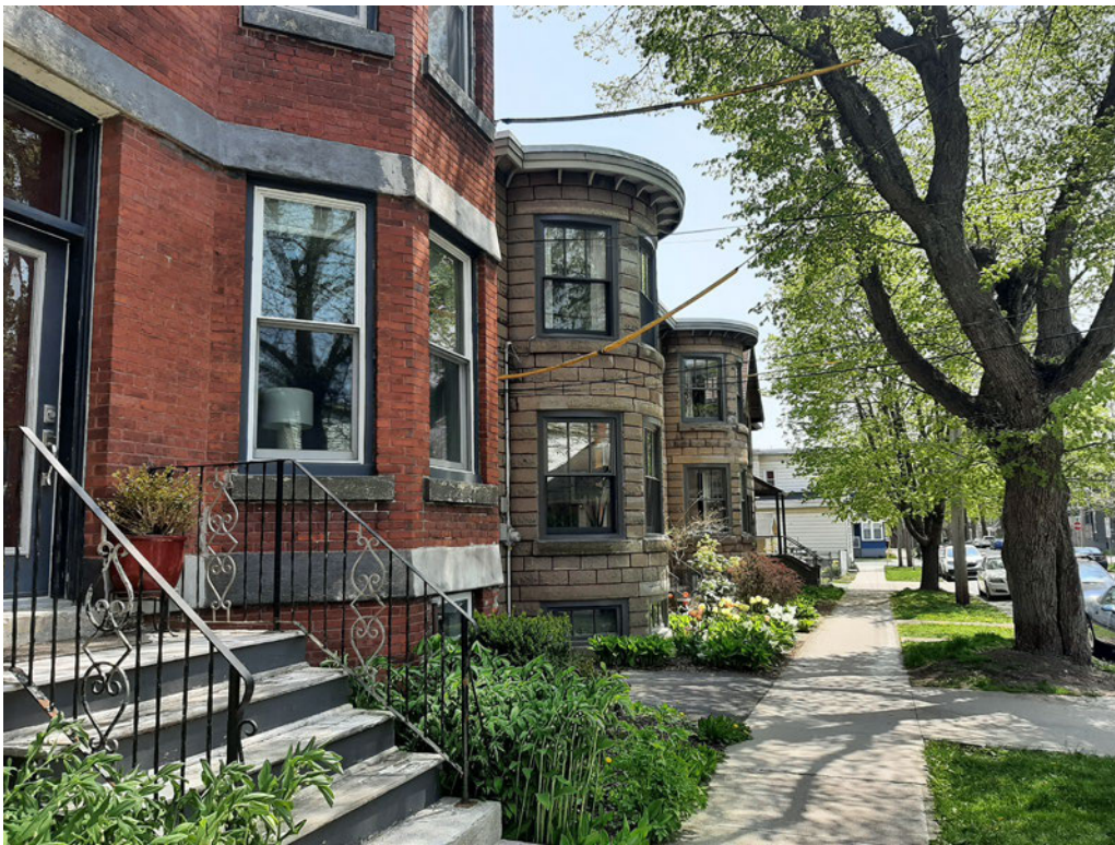
Figure 23: 1745 Henry Street facing south (19 May 2023)
