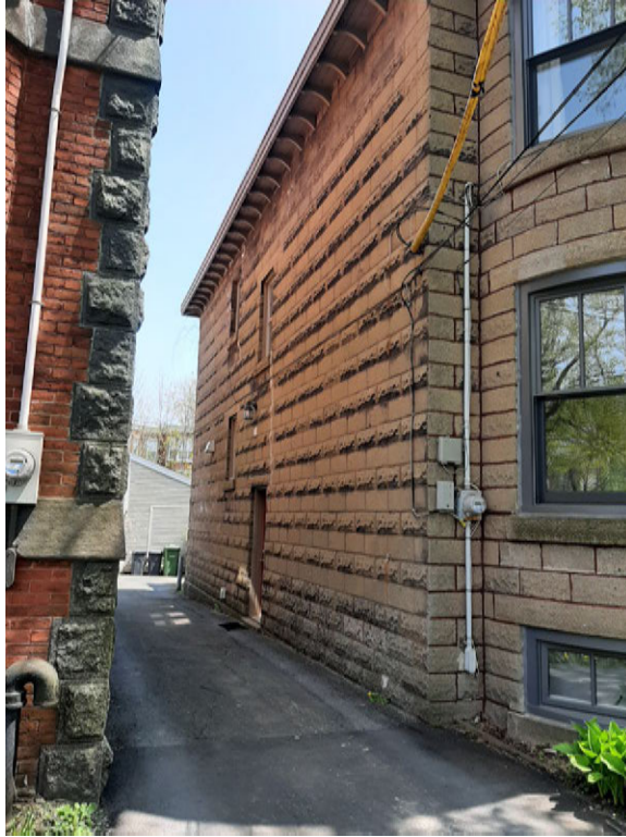
Figure 18: North elevation of 1745 Henry Street (19 May 2023)
