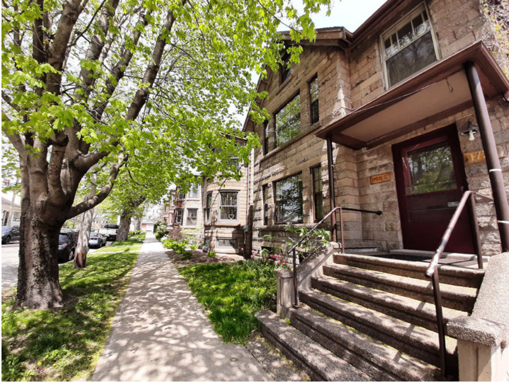
Figure 24: View of 1741-1743 and 1745 Henry Street facing north from 1735 Henry Street (19 May 2023)
