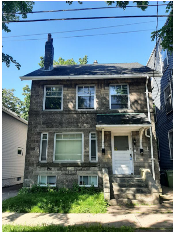
Figure 29: Concrete block house at 1740-1742 Henry Street (16 June 2023)
