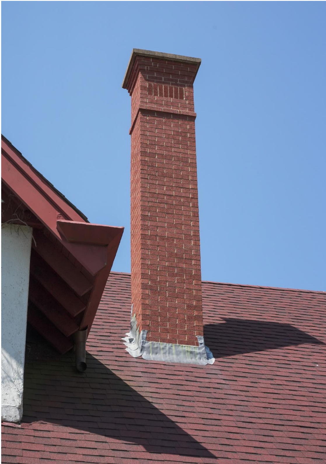
Figure 23: Detail of Chimney (Jun. 22, 2023)
