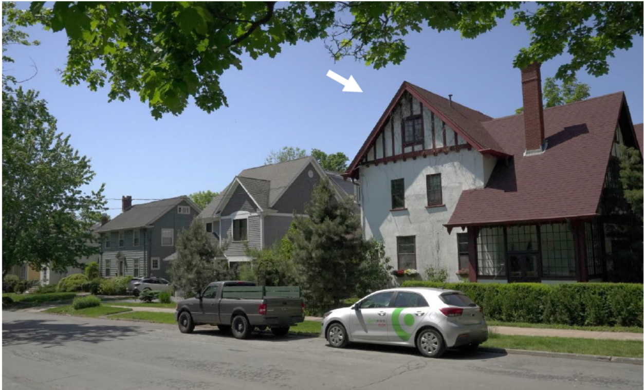
Figure 29: View looking southwest, with 6484 Jubilee Road highlighted by an arrow. (June 22, 2023)
