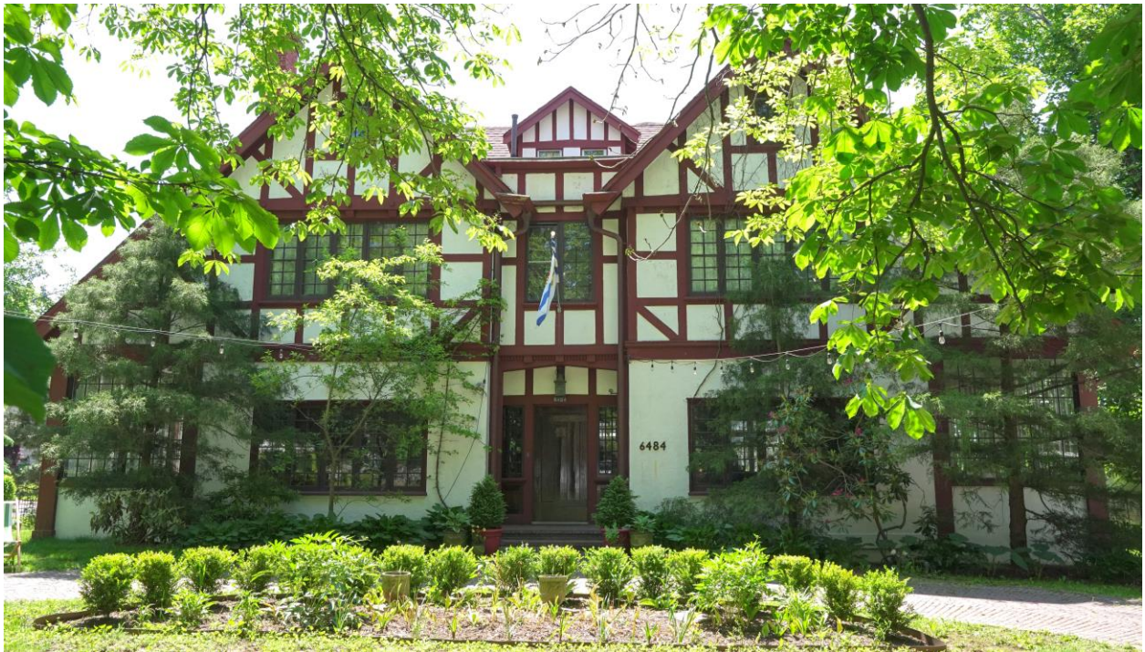
Figure 18: Northern elevation (Jun. 22, 2023)
