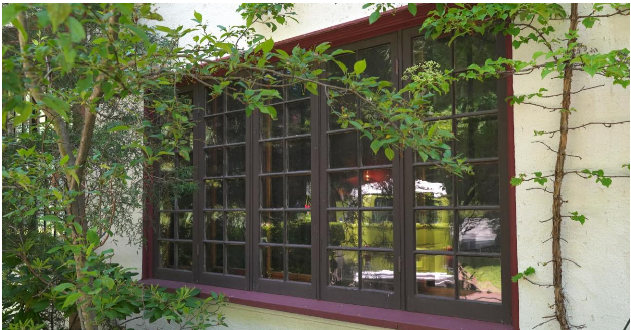
Figure 22: Detail of front window with wooden storm sashes. (Jun. 22, 2023)
