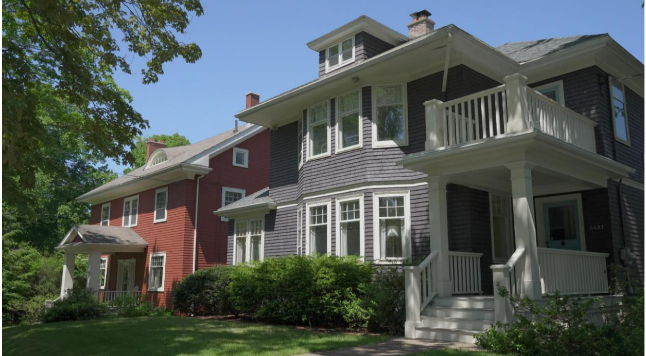
Figure 30: View opposite 6484 Jubilee Road, showing 6489 and 6481 Jubilee Road. (June 22, 2023)
