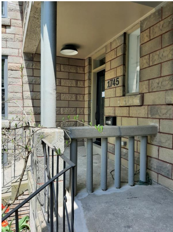
Figure 22: Front porch showing view of 1745 Henry Street entrance and colonettes (19 May 2023)
