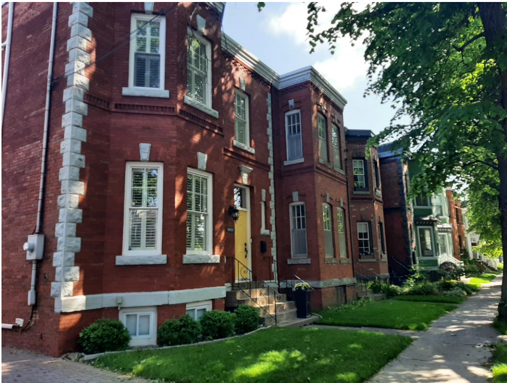
Figure 31: Maxwell homes on Jubilee Road, including registered properties at 6047 and 6053 Jubilee Road (16 June 2023)
