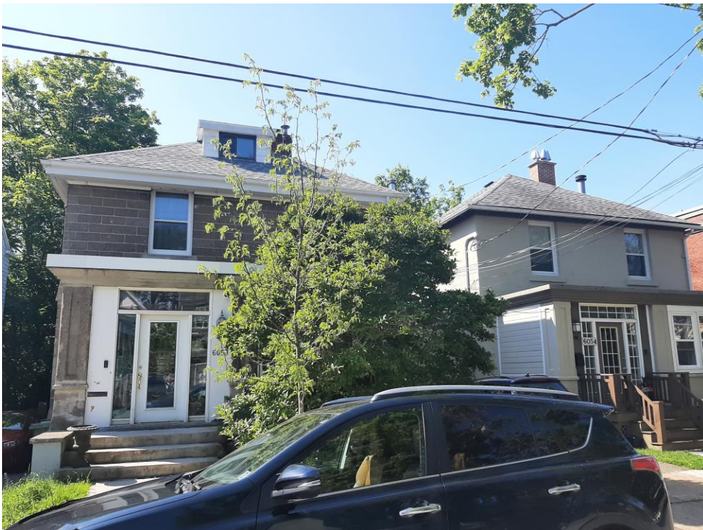
Figure 27: Concrete block homes on Cedar Street (16 June 2023)
