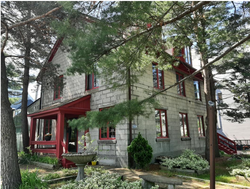
Figure 15: Hydrostone house at 5508 Novalea Drive (Staff Photo, 16 June 2023)
