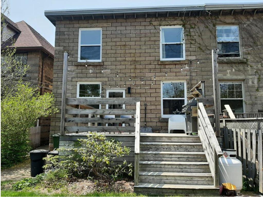
Figure 19: East elevation (19 May 2023)
