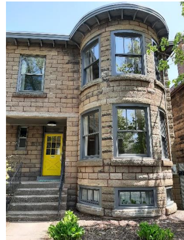
Figure 2: West elevation of 1741-1743 Henry Street (Staff photo, 19 May 2023)
