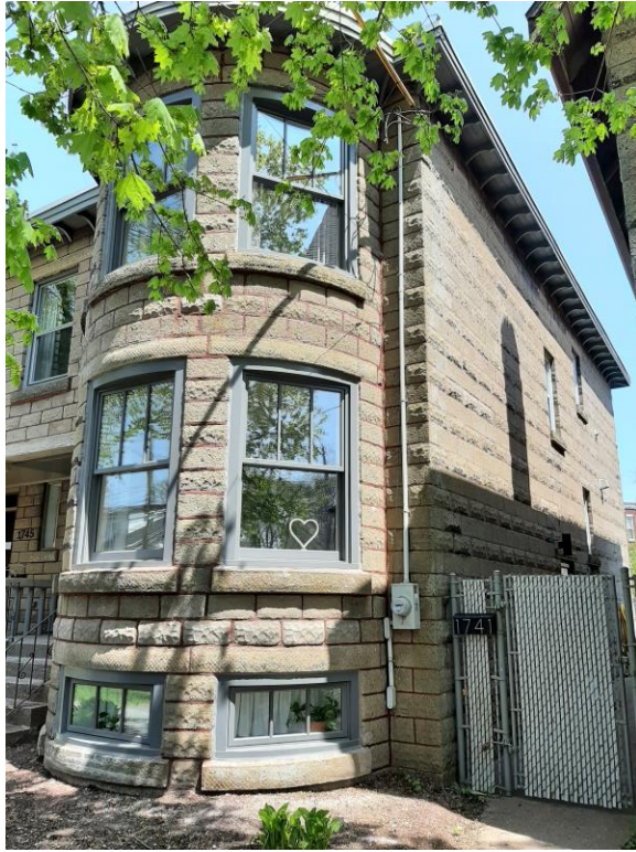
Figure 18: South and west elevation (Staff Photo, 19 May 2023)
