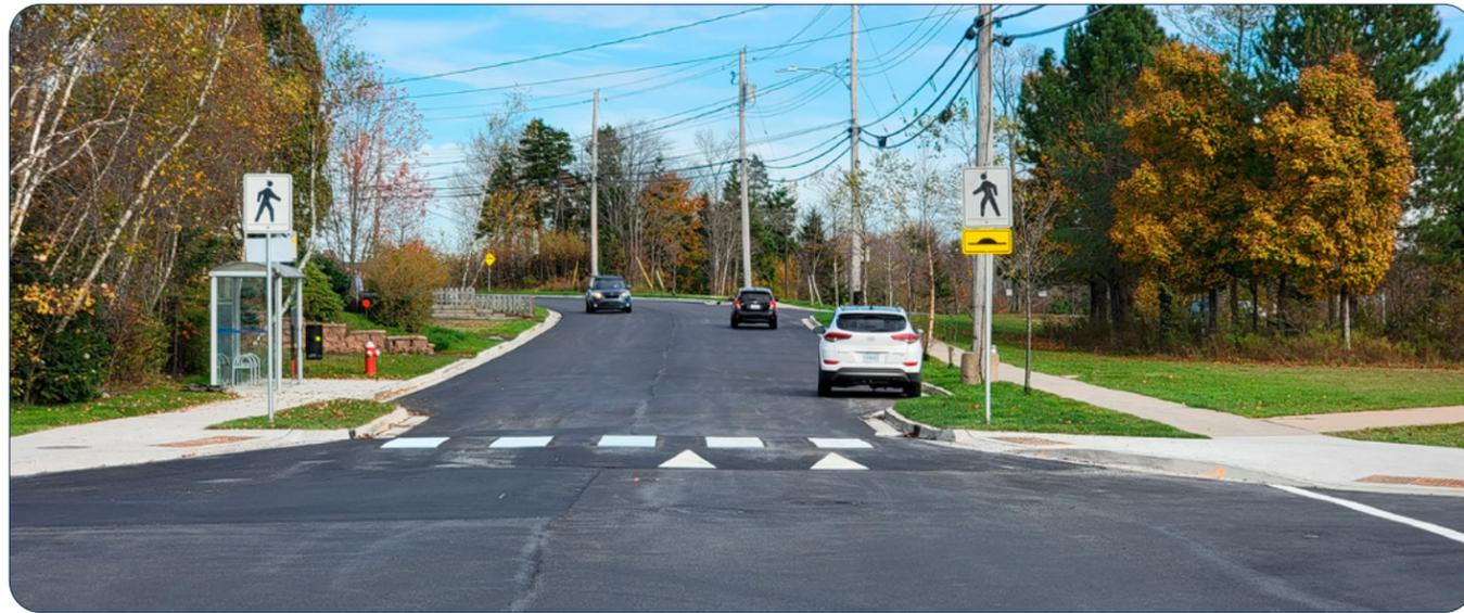
FIGURE 18: RAISED CROSSWALK INSTALLED ON AUBURN DRIVE, 2022 ^
