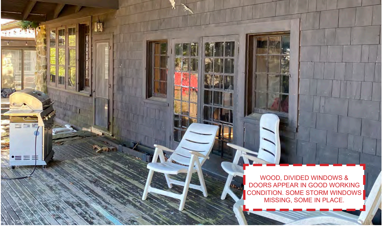
2.6 EXTERIOR WINDOWS & DOORS AT COVERED PORCH (EAST SIDE).
