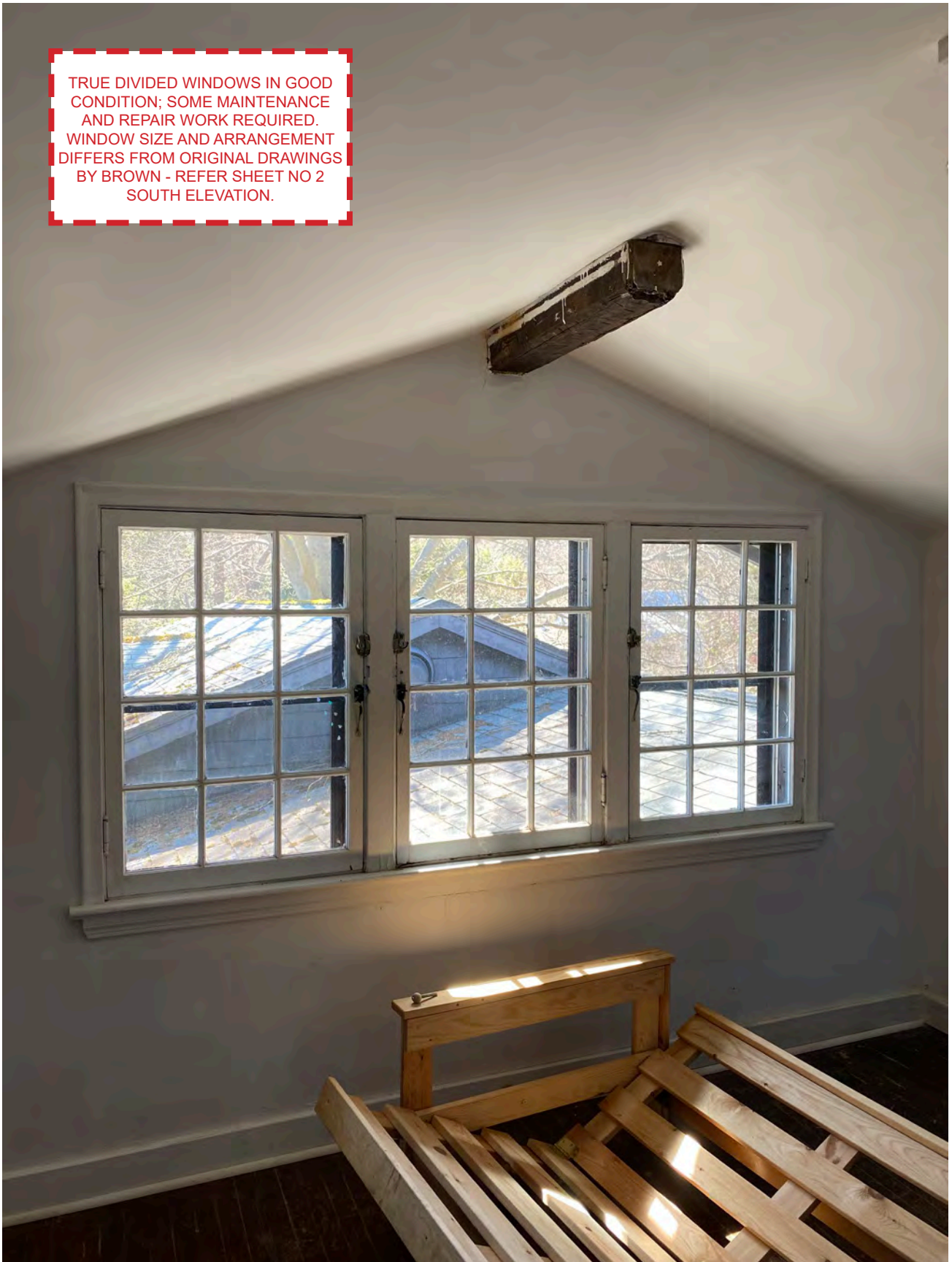
2.19 BEDROOM, UPPER FLOOR (SOUTH SIDE).
