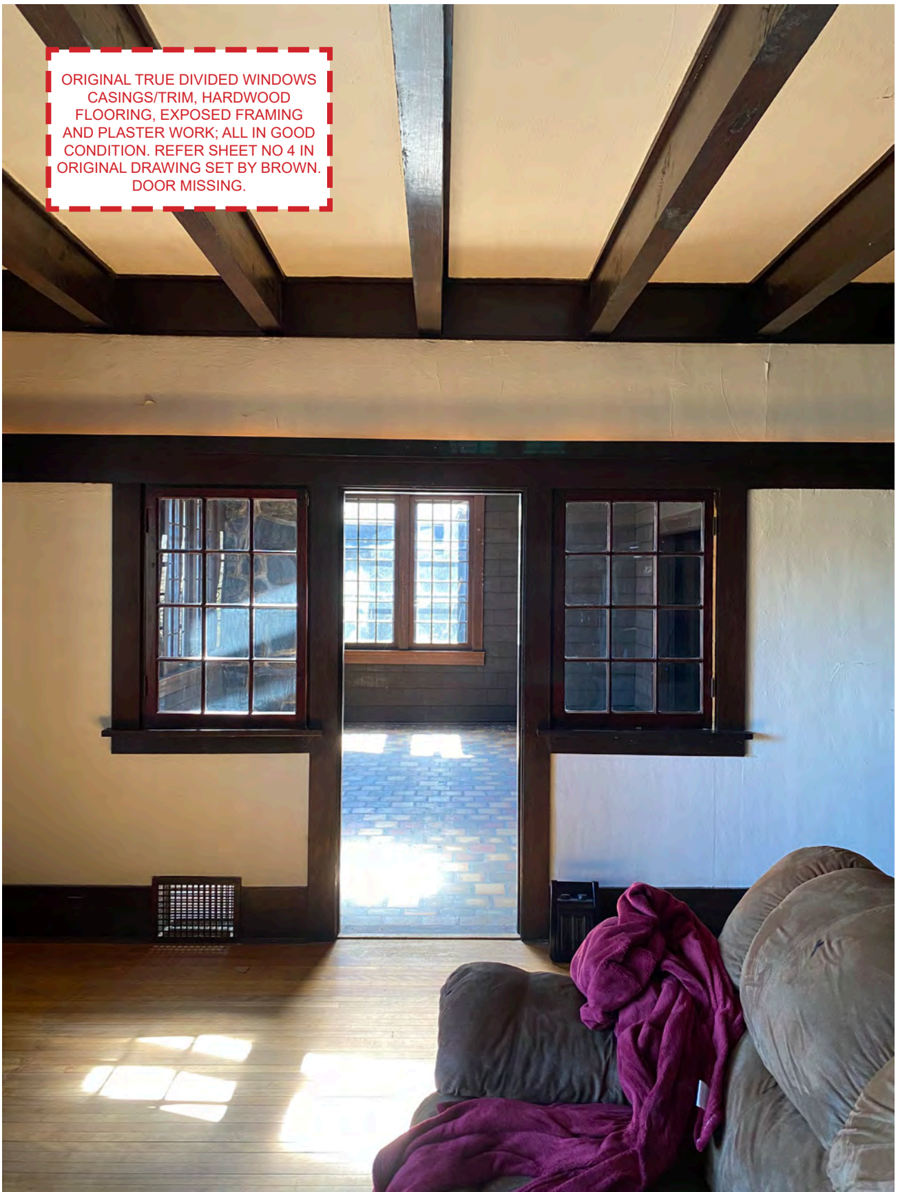
2.17 MAIN FLOOR LIVING ROOM (SOUTH).
