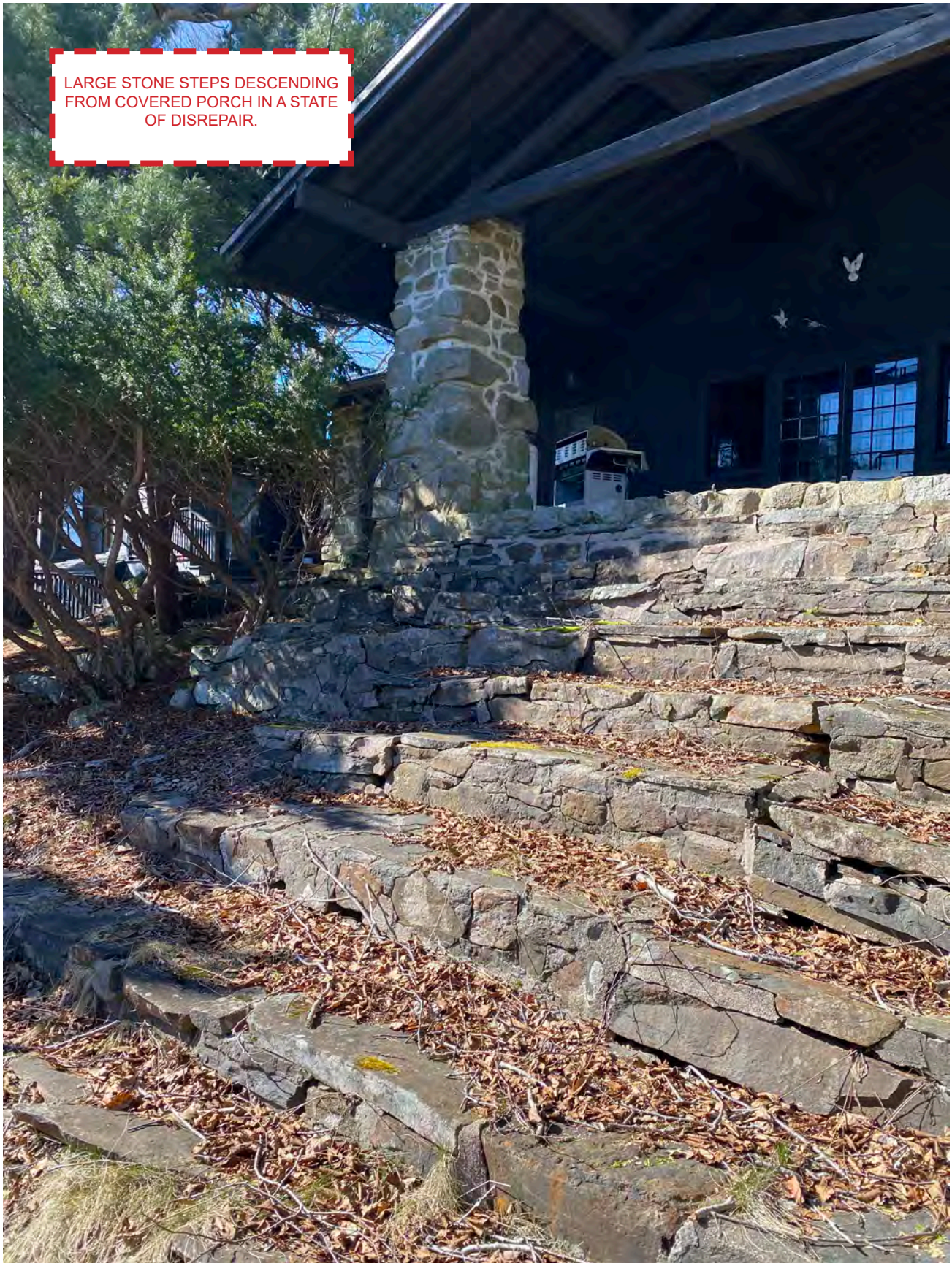
2.3 LARGE STONE STEPS AT COVERED PORCH (EAST SIDE).
