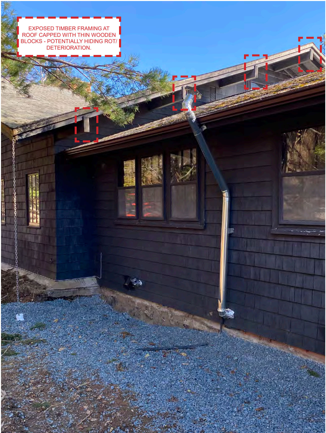
2.1 INTERSECTION OF ANNEX & MAIN HOUSE (SOUTH SIDE).
