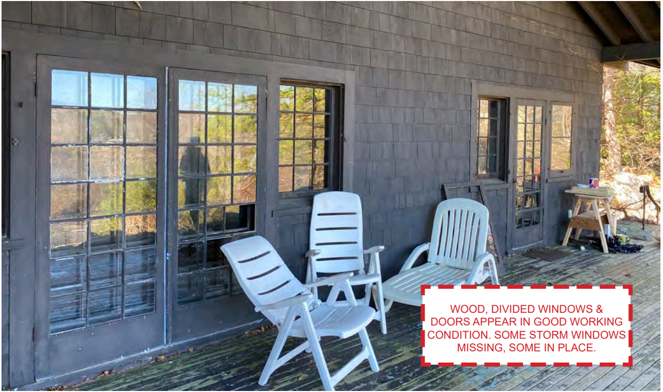
2.5 EXTERIOR WINDOWS & DOORS AT COVERED PORCH (EAST SIDE).
