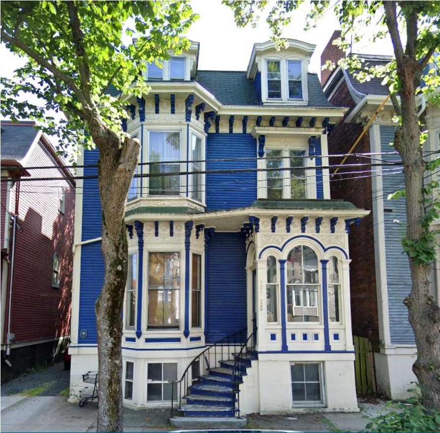
1099-1101 Tower Road, Halifax, front elevation.
