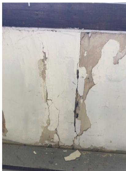
*Water damaged drywall underneath sliding window*
