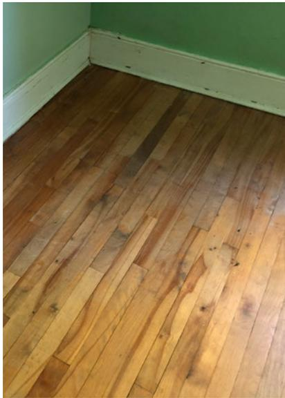
require few changes, except perhaps sanding and polishing. The carpet on the stairs should be removed and the wood underneath restored. All vinyl tiles on the first floor should be removed. It is presumed that these tiles were laid on an underlay overtop of historic, wood floors. If this is the case, the underlay should be removed and the wood floors restored. If this is not the case, the tiles should be replaced with period sensitive flooring.
