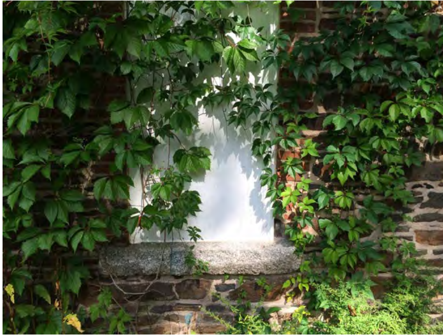
Figure 7 Ironstone foundation of original cottage
