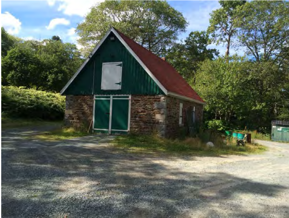
Figure 14 South elevation of barn
