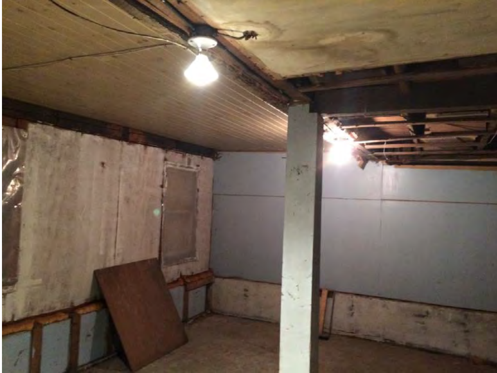
Figure 13 Basement of east addition
