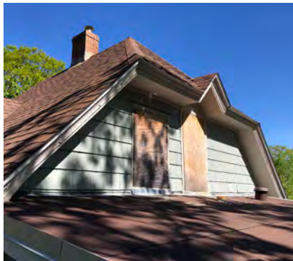
Asphalt shingle roof and modified bitumen roof
