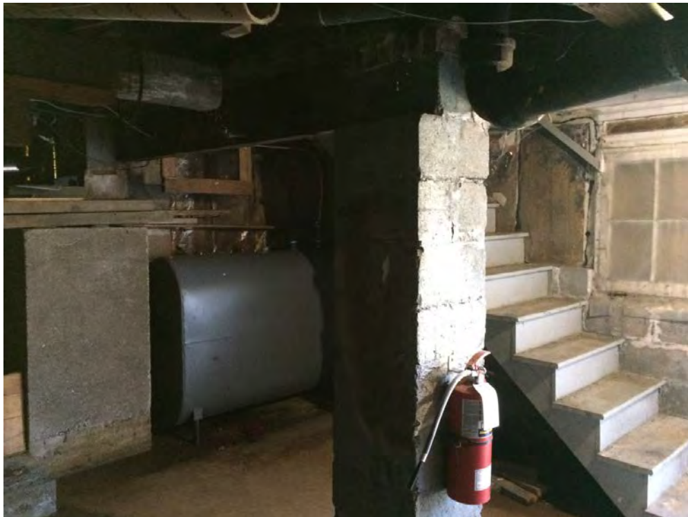
Figure 24 Stairs to basement
