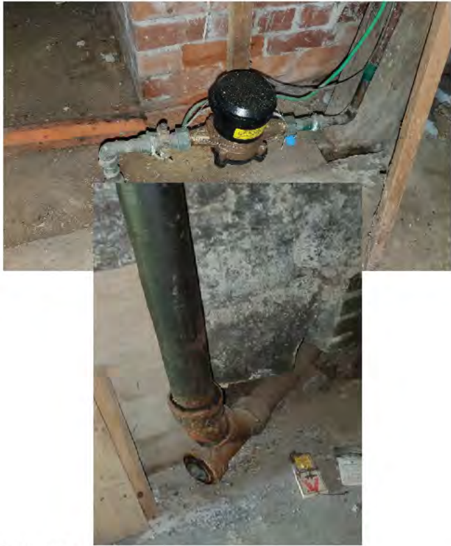
M1: Water Entrance
