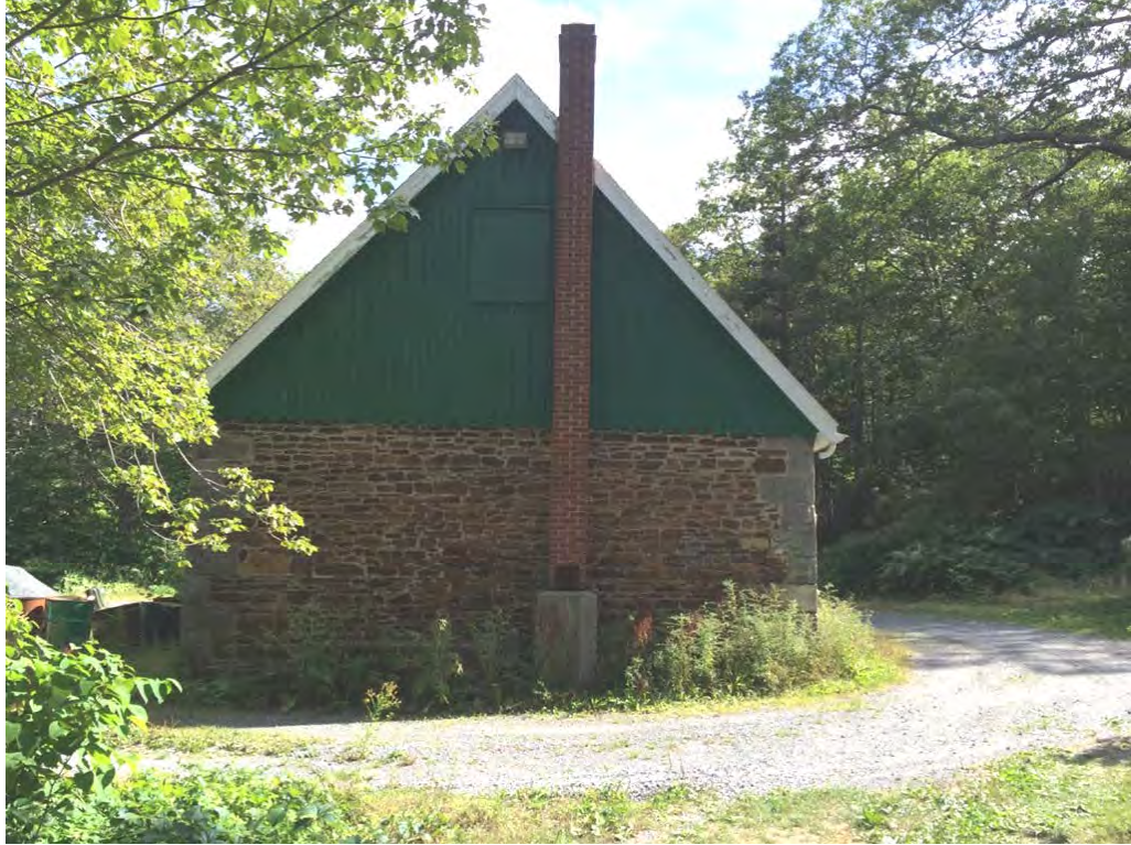
Figure 16 North elevation of barn
