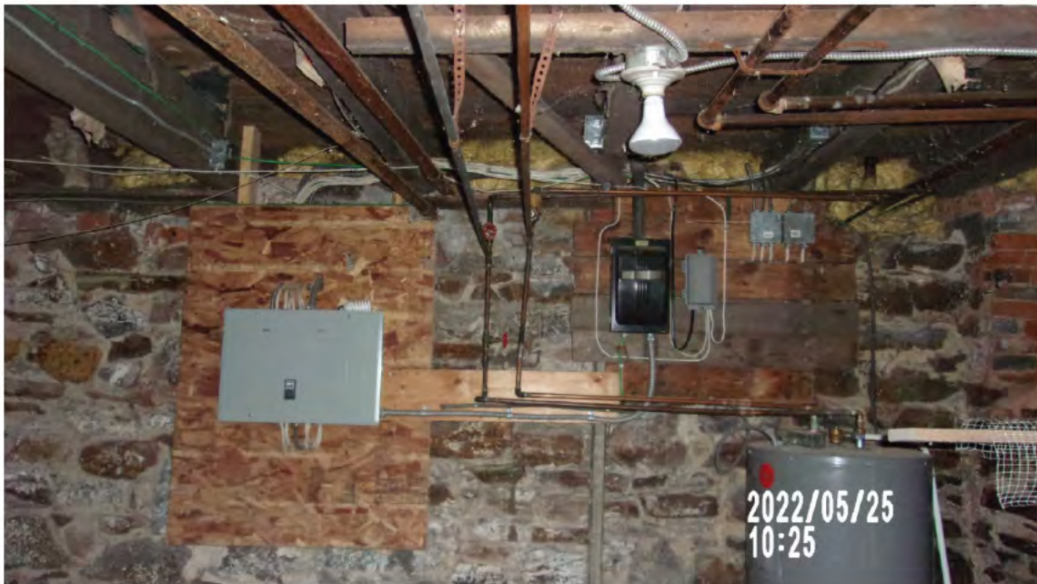
E2- Electrical Service Entrance Equipment
