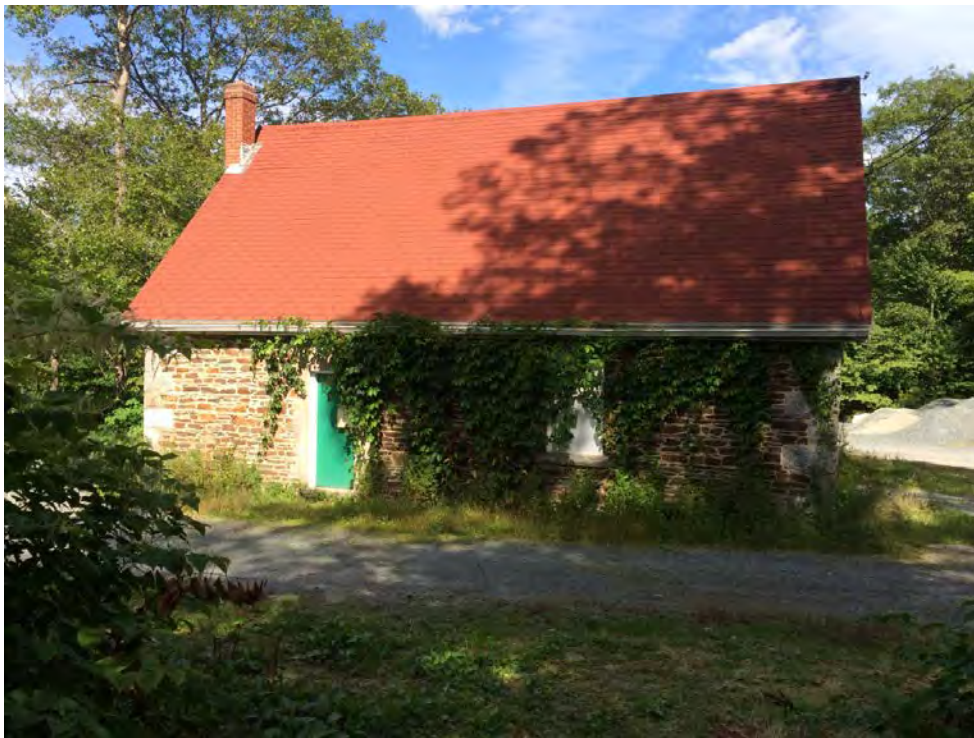
Figure 15 West elevation of barn
