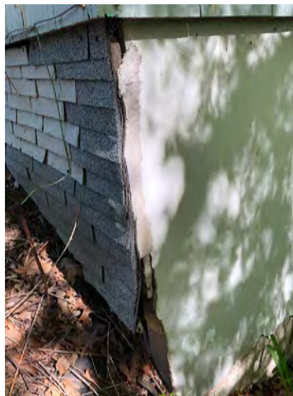
Concrete foundation wall and asphalt shingle clad foundation wall
