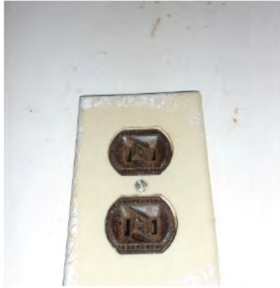
E7- Typical Ungrounded Receptacle.
