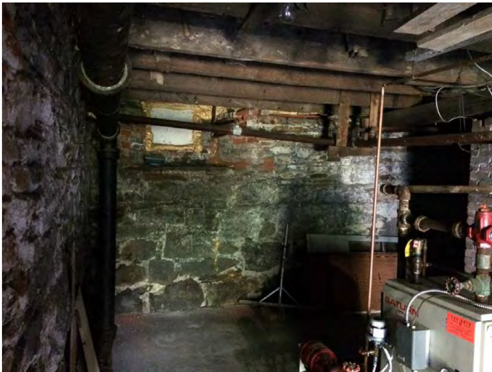
Figure 12 Ironstone foundation under original cottage
