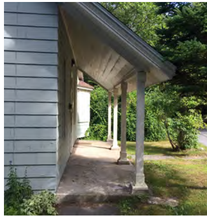
Step onto concrete porch
