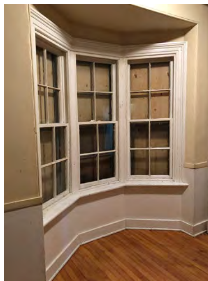
Original windows in kitchen
