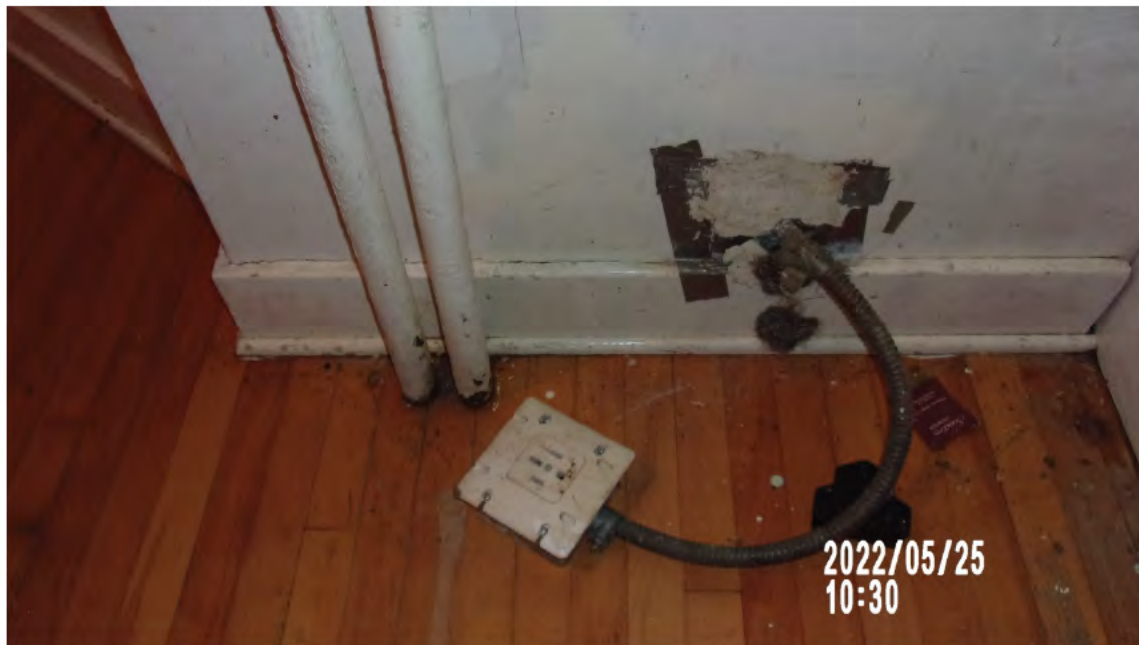
E7- Typical Ungrounded Receptacle.
