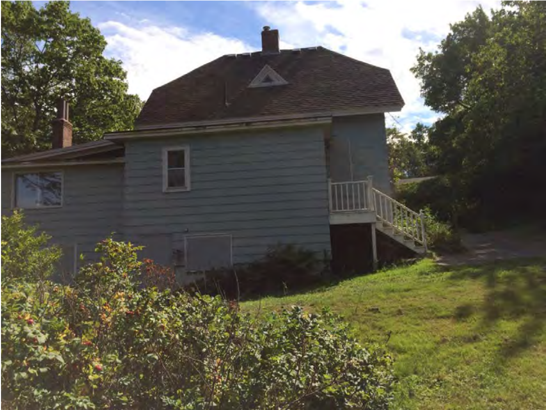
Figure 10 East addition viewed from north
