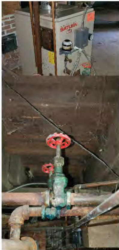
M4: Oil Fired Boiler
