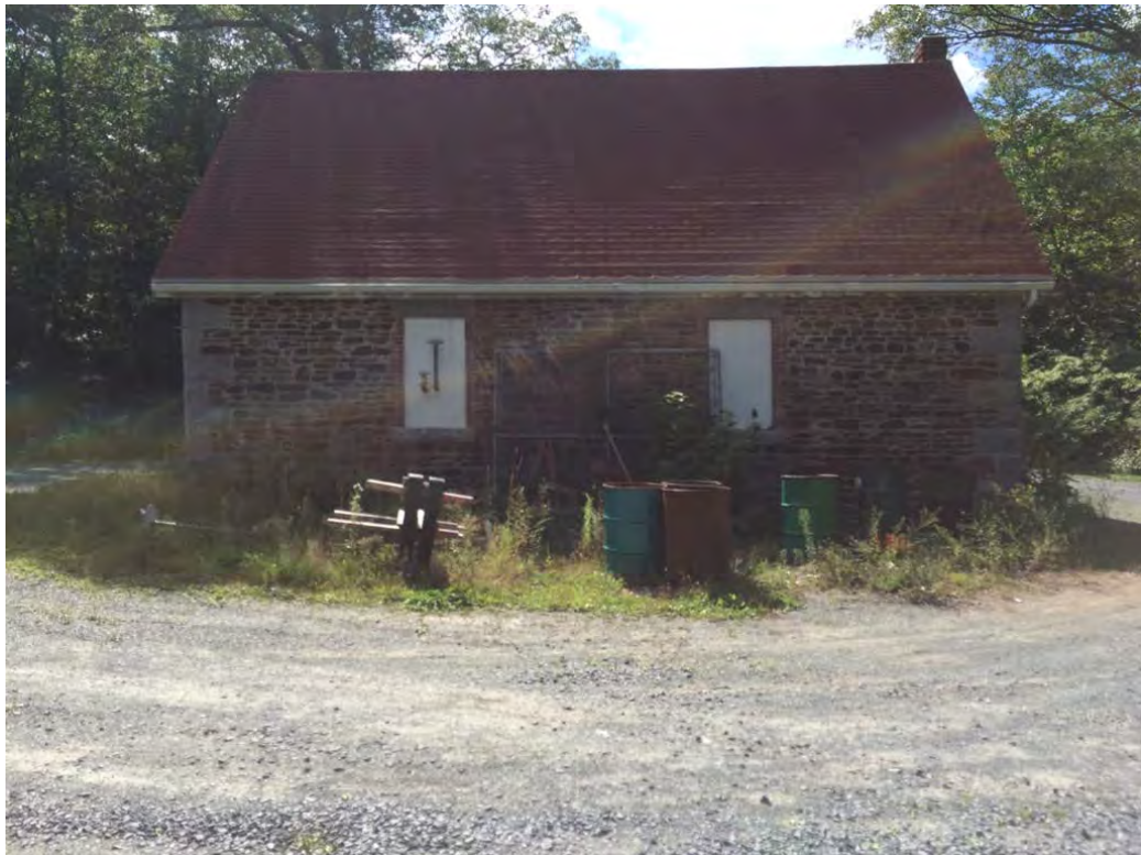
Figure 17 East elevation of barn
