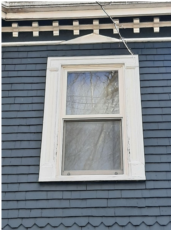
Figure 14: Second storey window with label-like trim (Staff photo, 22 February 2023)
