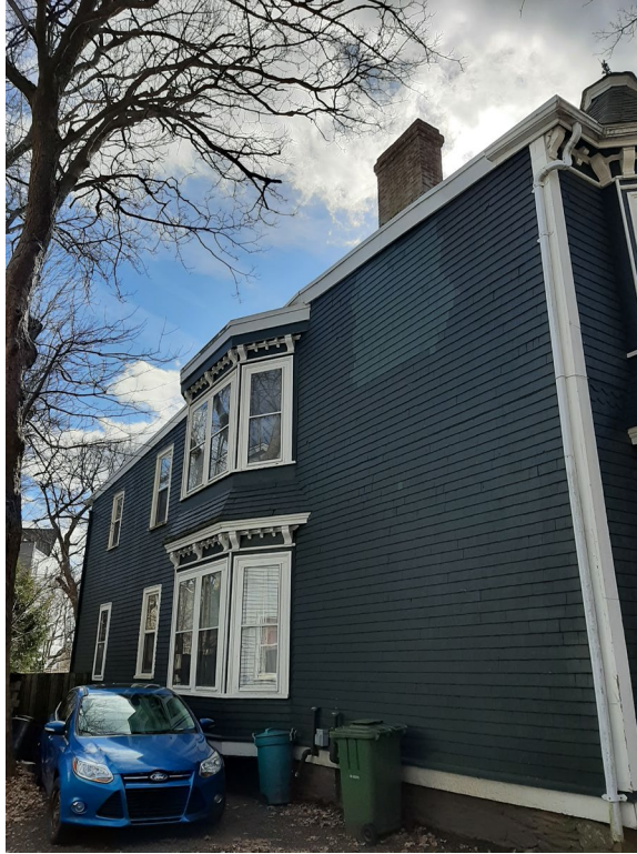
Figure 11: East elevation (Staff photo, 22 February 2023)
