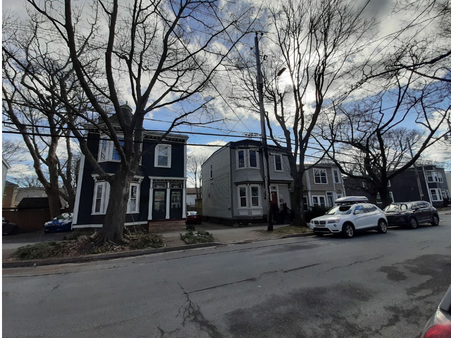
Figure 19: 6032-6034, 6038 and 6040 Charles Street (Staff photo, 22 February 2023)
