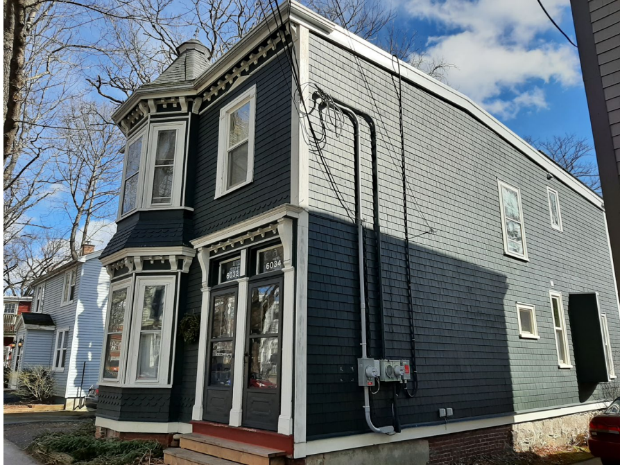
Figure 9: West elevation (Staff photo, 22 February 2023)
