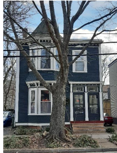
Figure 1: 6032-6034 Charles Street (Staff photo, February 22, 2023)
