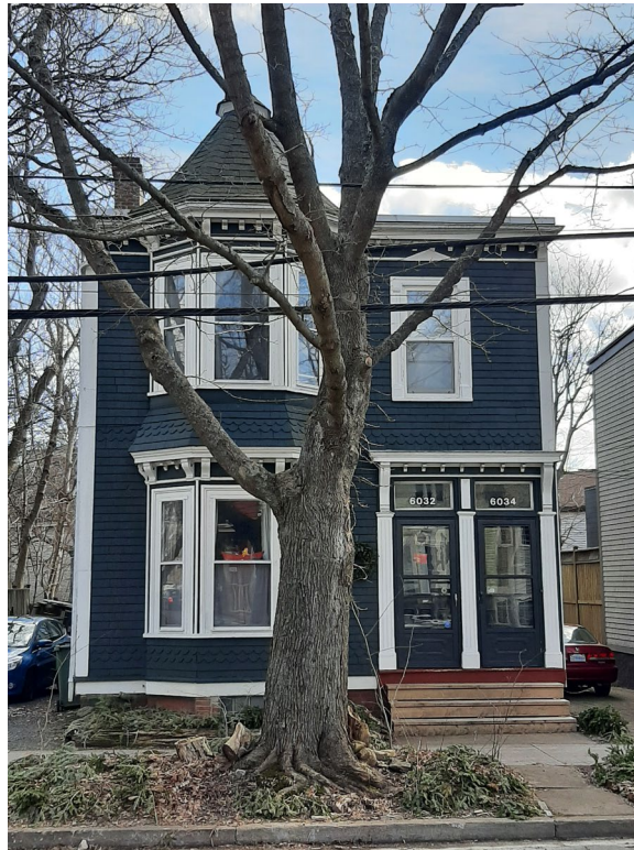
Figure 8: North elevation of 6032 Charles Street (Staff photo, 22 February 2023)
