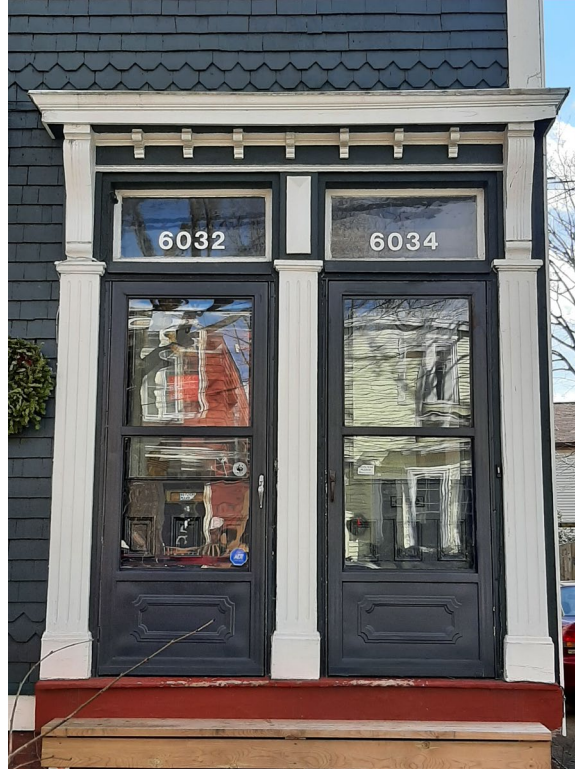
Figure 15: Main entrances to 6032-6034 Charles Street, with wood pilaster, corbels and brackets and transom (Staff photo, 22 February 2023)
