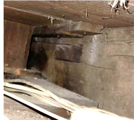
Figure 14: Photo by the property owners showing a large timber with a mortise and tenon joint. (February 28, 2022)
