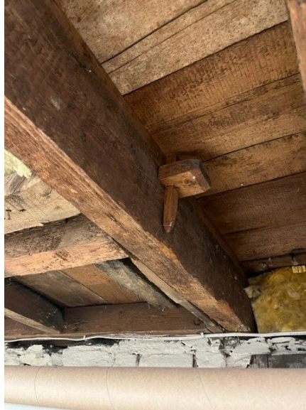
Figure 13: Mortise and tenon construction as visible from the basement of 1206 Robie Street (Source: Property Owner)
