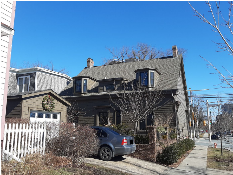
Figure 16: West elevation (Staff photo, 22 February 2023)
