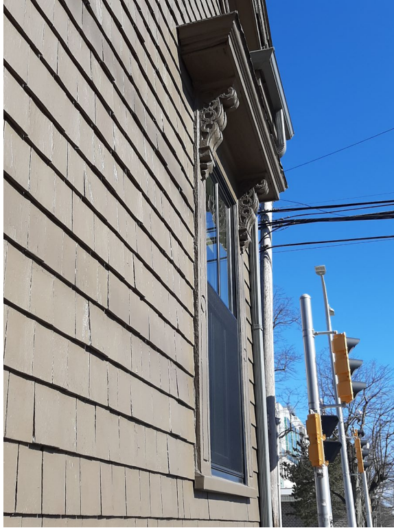
Figure 19: Corbel detailing on the moulded lintel, south elevation (Staff photo, 22 February 2023)
