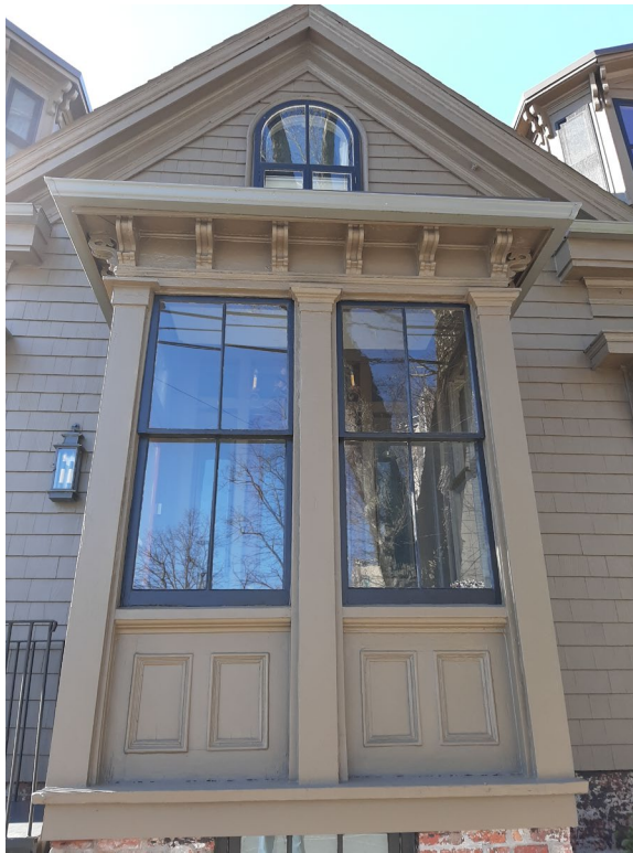
Figure 20: Centre gable with semi-circular window and storm porch, east elevation (Staff photo, 22 February 2023)
