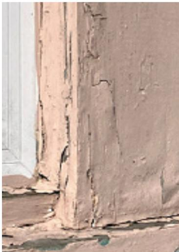
**Fig. 34** The window trim is mostly rotten and will be replaced. The vinyl windows are outworn and will be replaced with triple glazed vinyl windows to look original
