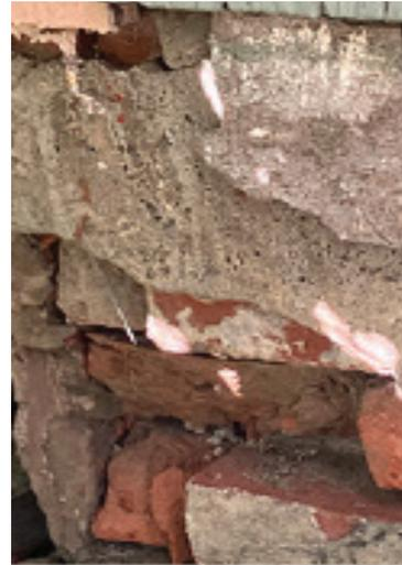
**Fig. 35** Foundation is structurally unsound, and will be replaced with a new foundation featuring reclaimed brick veneer.
