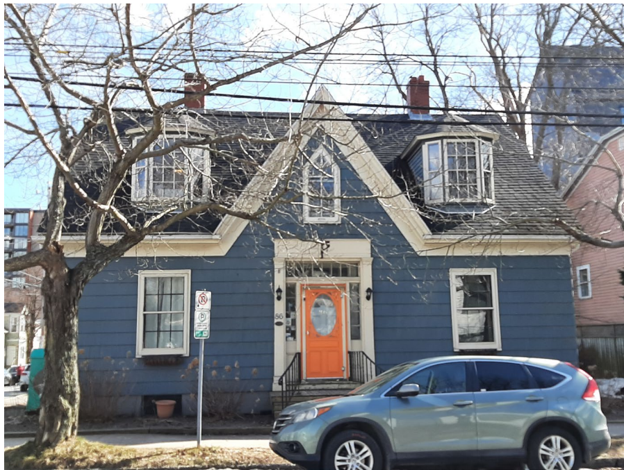
Figure 11: 86 Ochterloney Street (Staff photo, 22 February 2023)
