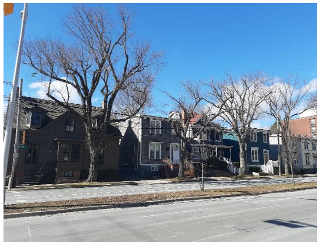
Figure 3: View of 1206 Robie Street from the northeast corner of the Robie and South Streets intersection (Staff photo, February 22, 2023)
