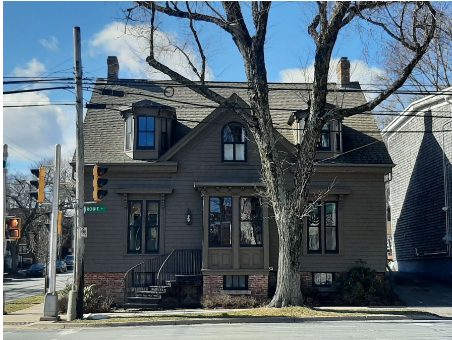
Figure 14: East elevation of 1206 Robie Street (Staff photo, 22 February 2023)
