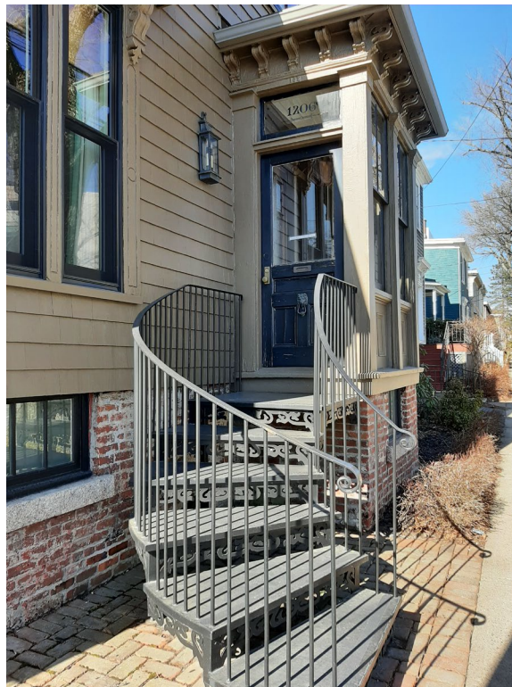
Figure 22: Curved staircase leading to the exterior wood glazed door with transom above on the storm porch. Original 132 civic address is visible above the transom (Staff photo, 22 February 2023)
