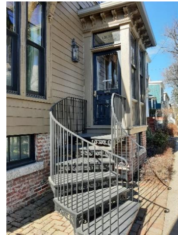
Figure 2: Curved metal staircase leading to the storm porch of 1206 Robie Street (Staff photo, 22 February, 2023)
