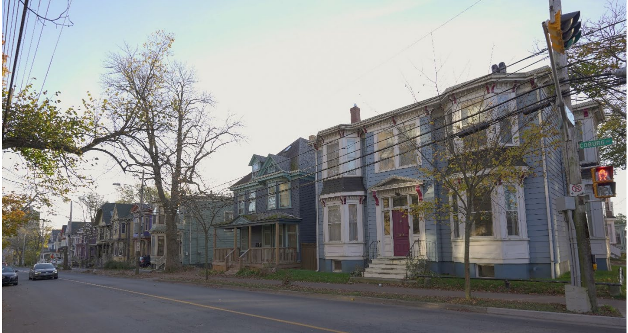
Figure 31: View looking east, with 6112 Coburg Road to the right. (Nov. 4, 2022)
