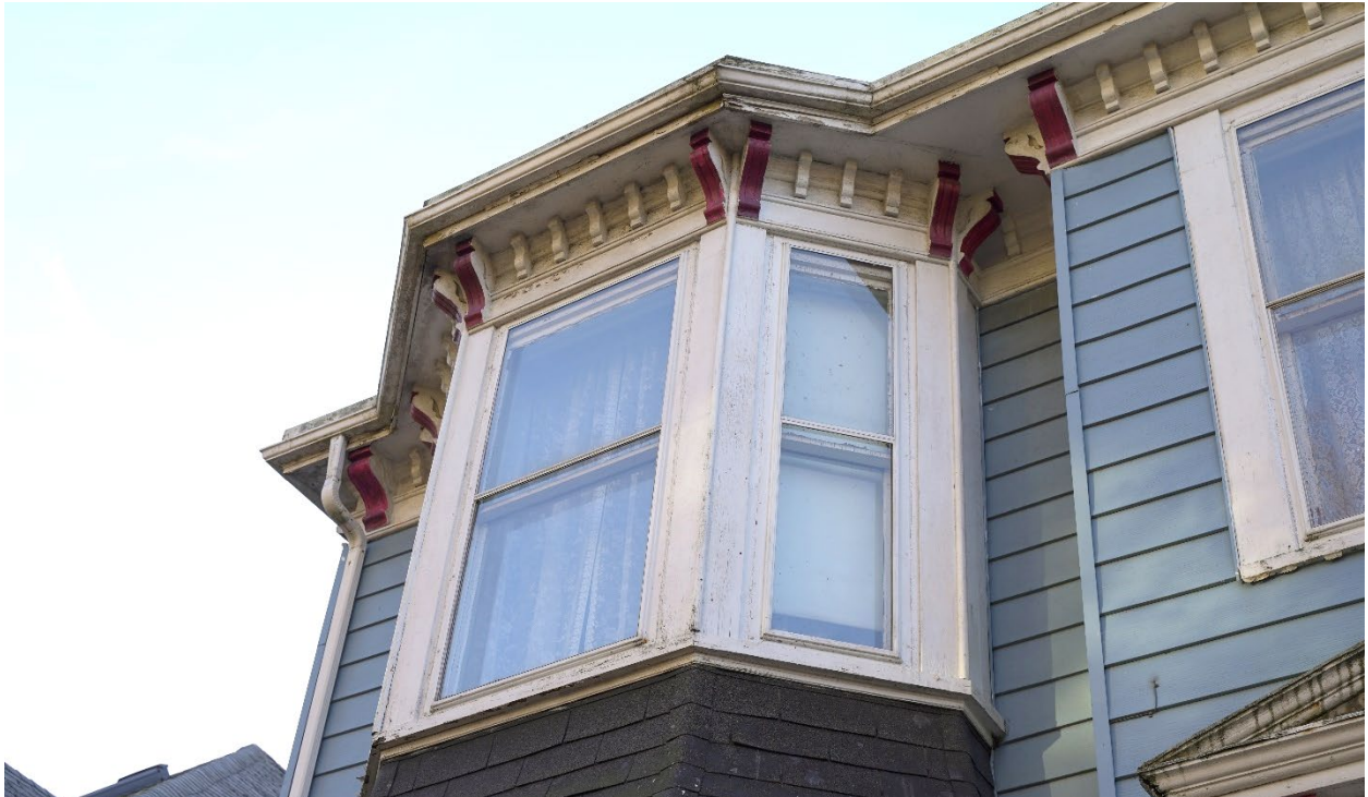
Figure 22: Detail of upper bay (Nov. 4, 2022)
