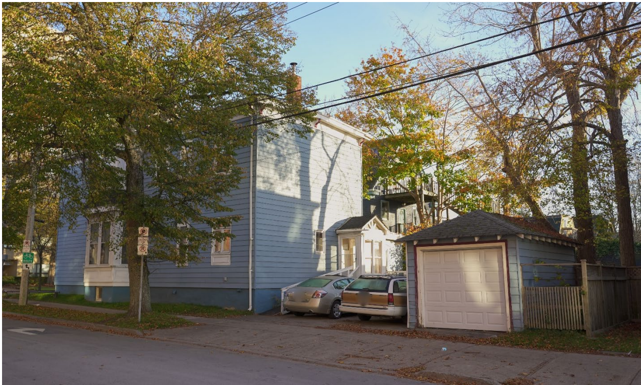
Figure 17: Rear elevation (Nov. 4, 2022)
