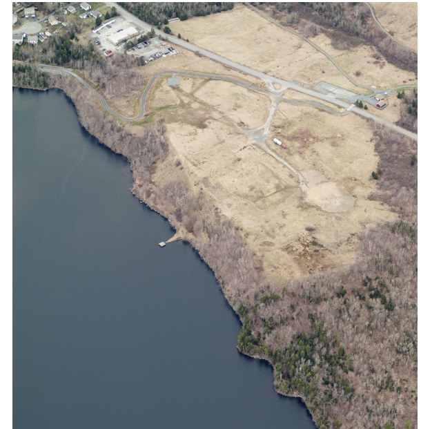
FIGURE 5: AERIAL PHOTO OF REHAB LANDS 2020 SHOWING THE BISSETT TRAIL AND SITE REMEDIATION
