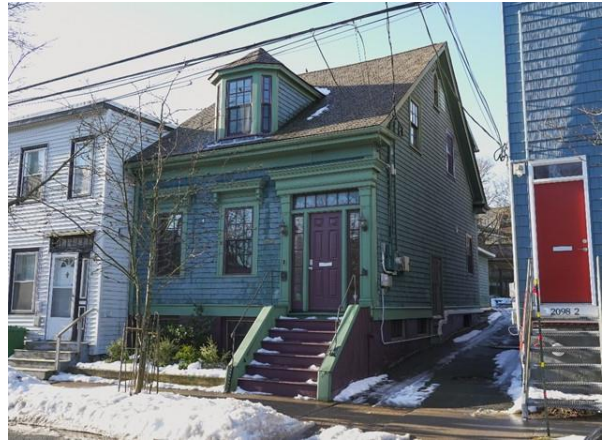
Figure 1: 2096 Creighton Street (Feb. 15, 2023)
