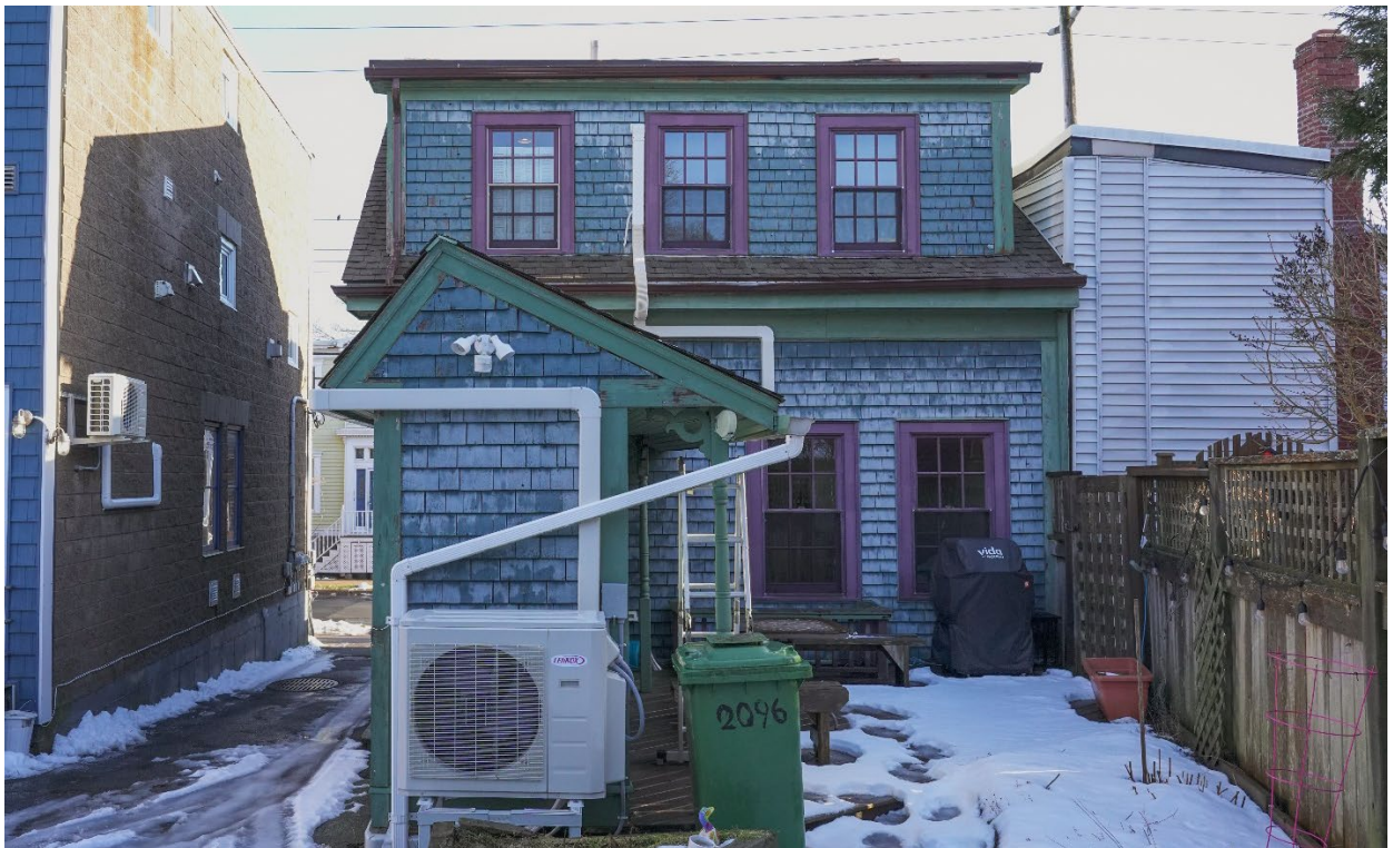
Figure 17: Western elevation (Feb. 15, 2023)
