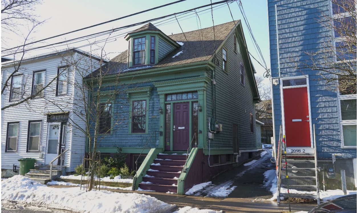
Figure 16: Northeastern elevation (Feb. 15, 2023)
