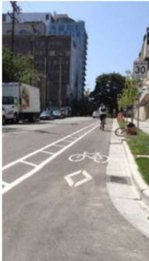
Paint Buffered Bike Lane
